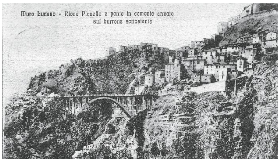
Image 2: The Pianello Bridge on a vintage postcard. Built between 1916 and 1918, it is one of the first reinforced concrete structures built in Southern Italy.
