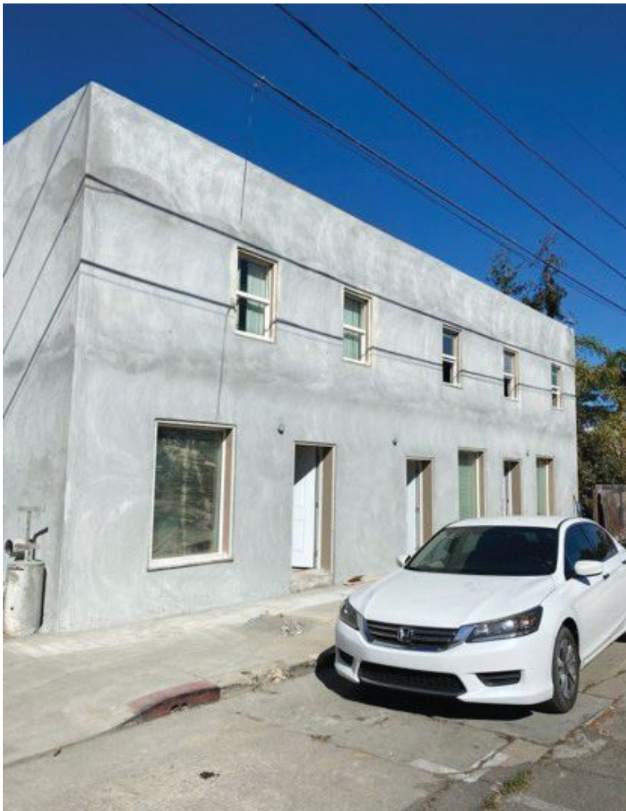
Figure 12: Structure exterior — after.
