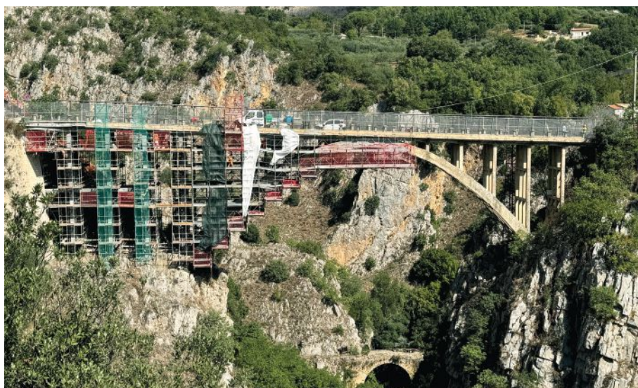
Image 3: The restoration of the Pianello Bridge in Italy using FRCM has secured one of the earliest reinforced concrete structures in Europe.
