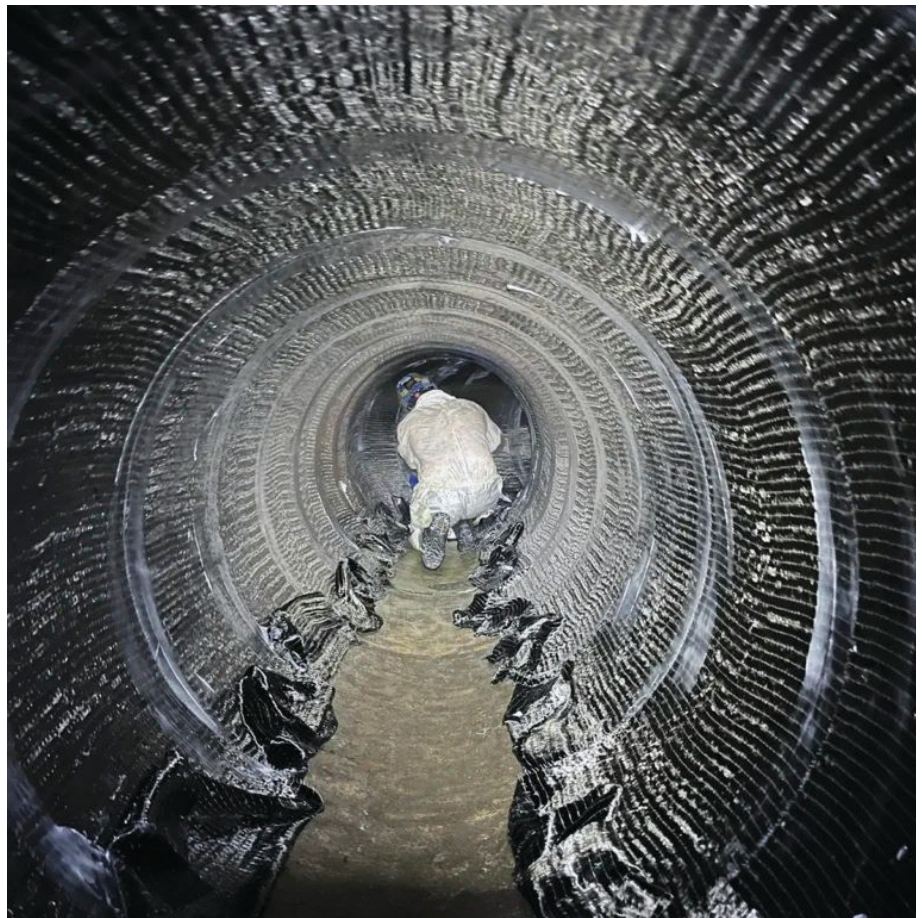
Figure 3: Working in cramped and confined spaces increases worker fatigue. (Courtesy of Structural Preservation Systems)
