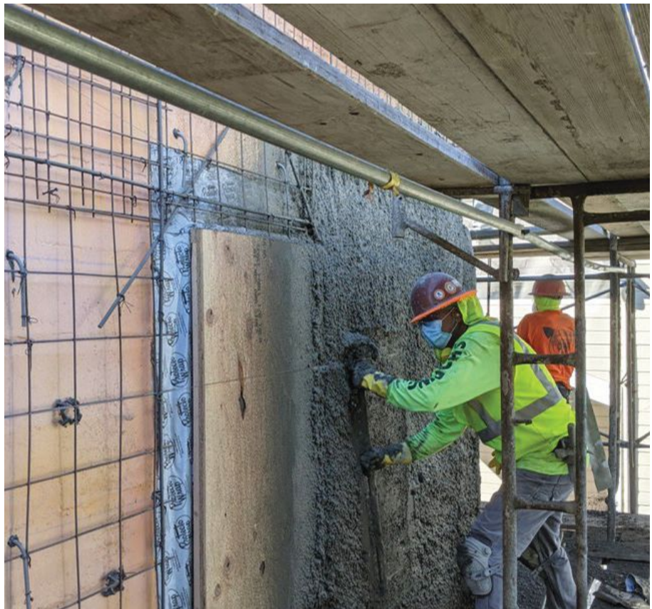
Figure 8: Structural shotcrete curtain construction.
