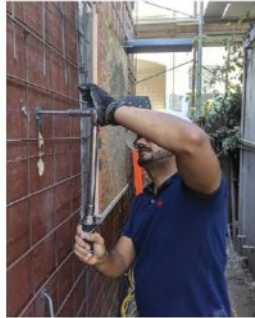
Torque Test on Wall Anchors
