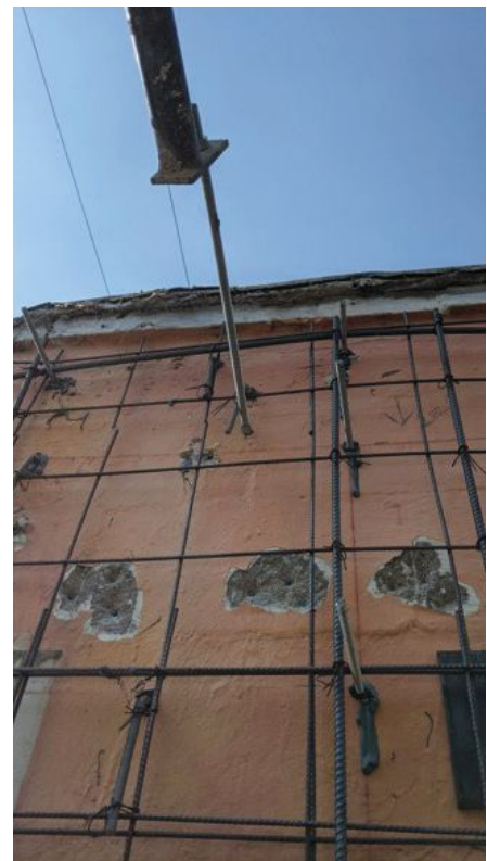
Figure 9: Curtain reinforcement template and installation.
