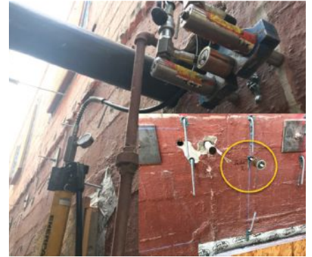
Figure 11: Wall anchor tension test.
