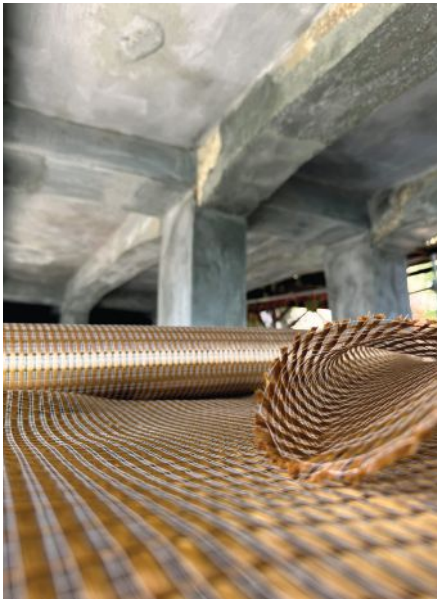
Image 4: The PBO-FRCM system, based on a bidirectional mesh combined with the inorganic matrix, installed on the bridge.
