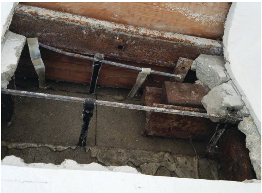
Figure 5: Wall interior — mixed materials.
