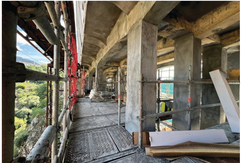
Image 5: View of the bridge's structural elements addressed by the reinforcement work using the FRCM system.
