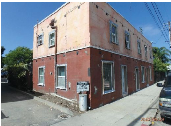
Figure 2: Structure exterior — before.
