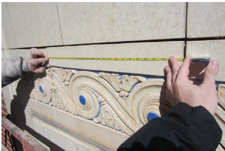
Fig. 2: Measurements of the polychromatic terra cotta units and total quantities were made to determine the available quantity for the reinstallation
