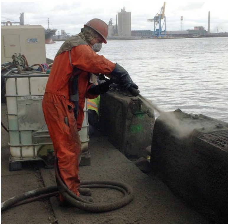
Fig. 6: Dry process shotcrete application
