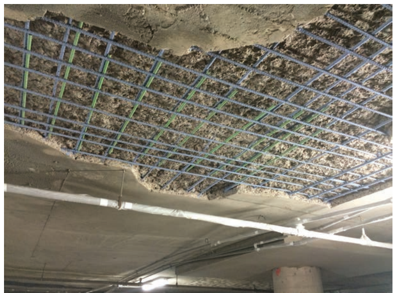
Fig. 4: Overhead repair in parking garage to receive dry process shotcrete
