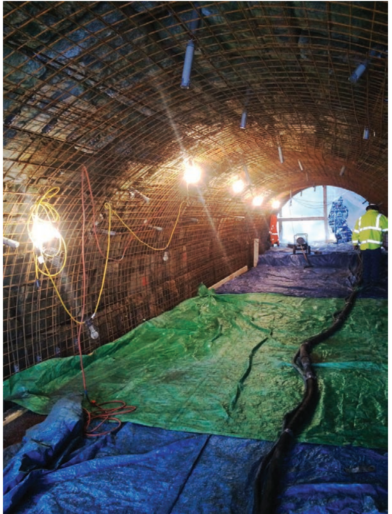
Fig. 3: Tunnel damaged by Hurricane Sandy ready to receive 8 in (203 mm) structural lining for repair and strengthening
