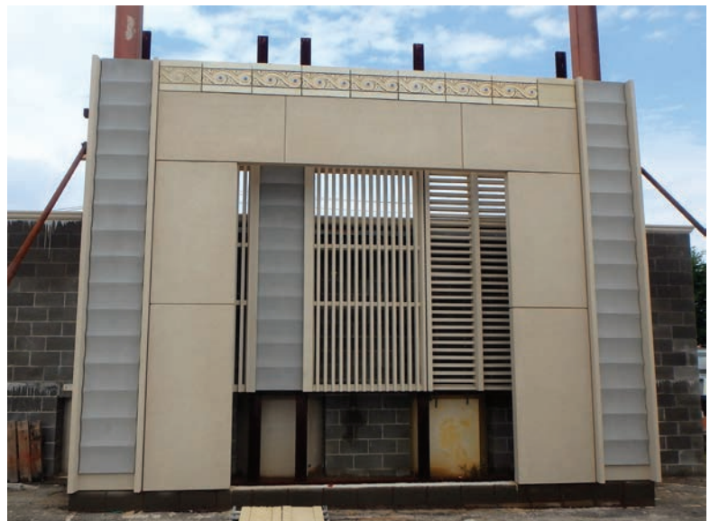
Fig. 6: Full scale mock-up of the terra cotta frieze installed into the GFRC panel (note that the end pieces were recreated units being reviewed for acceptance in the final installation)
