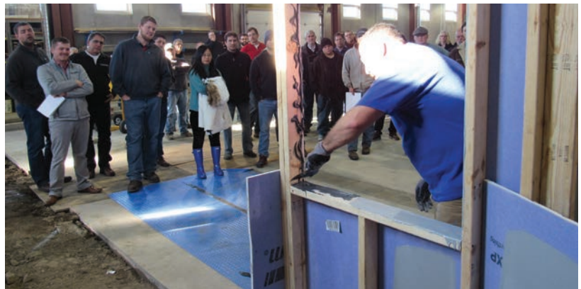
Garet Hovest with BASF demonstrates detail work for thin-mil air & vapor barriers
