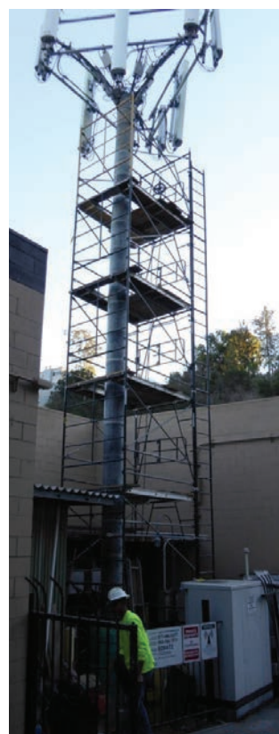
Fig. 7: Retrofitted pole prior to the application of paint and removal of the scaffolding
