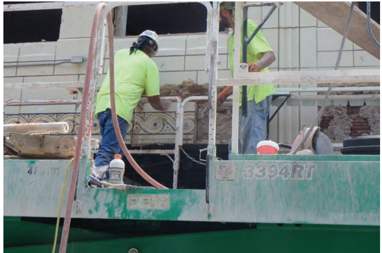
Fig. 5: Frequent visits to the site allowed for opportunities to observe and provide alternate strategy for removal of the terra cotta
