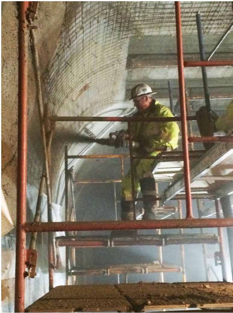
Fig. 9: Wet process shotcrete application
