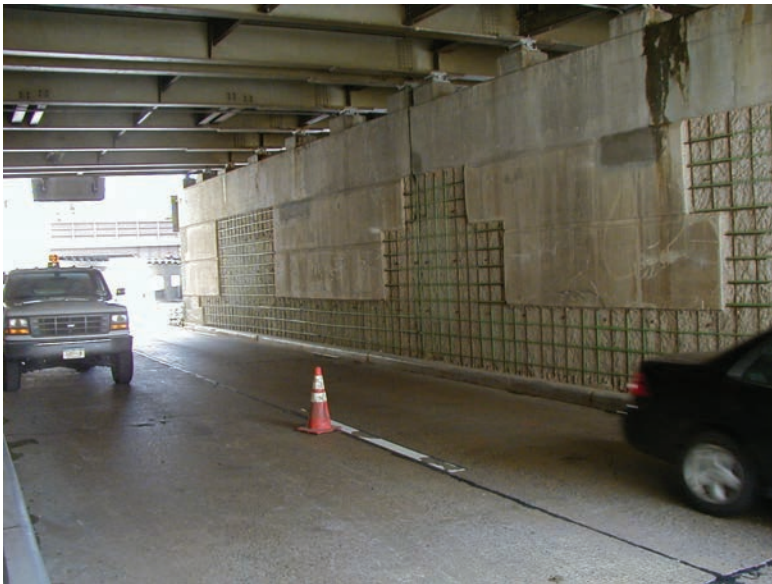
Fig. 1: Large continuous vertical repair areas are particularly suited for PACM
