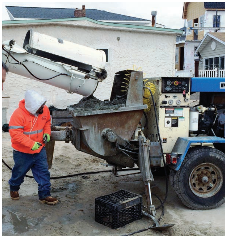
Fig. 8: Ready-mix shotcrete used for wet process application
