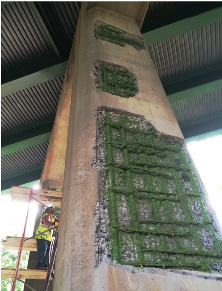
Fig. 5: Repair areas ready to receive shotcrete at column
