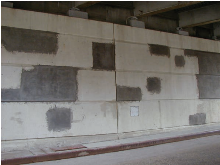
Fig. 2: Multiple areas repaired using PACM
