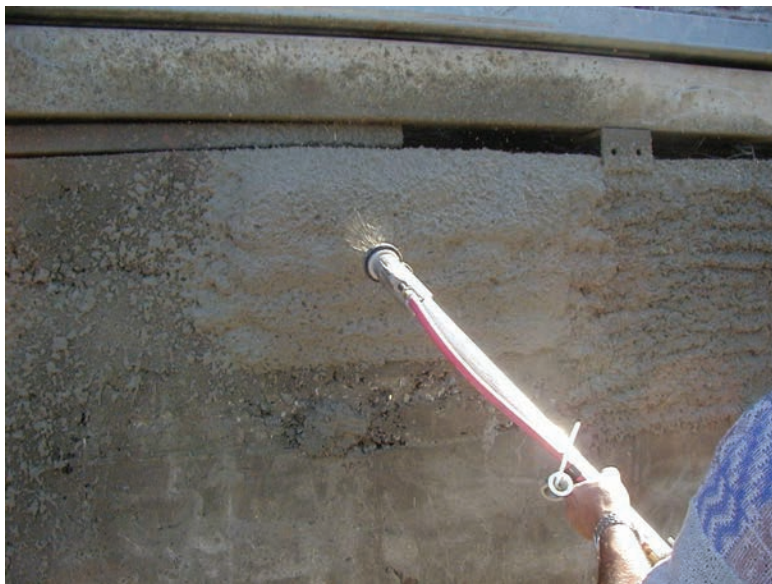
Fig. 11: Wet spray propels material at much lower velocity than shotcrete
