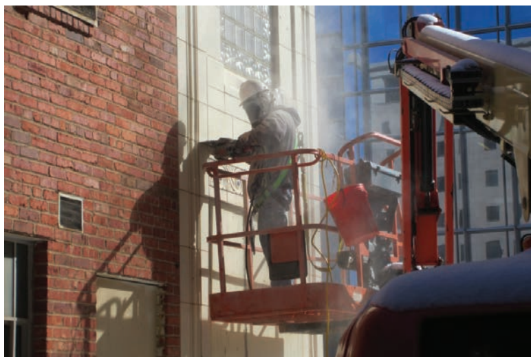
Fig. 3: Selective removal and exploratory openings during the investigation were used to determine the type of connection of the terra cotta to the back-up wall
