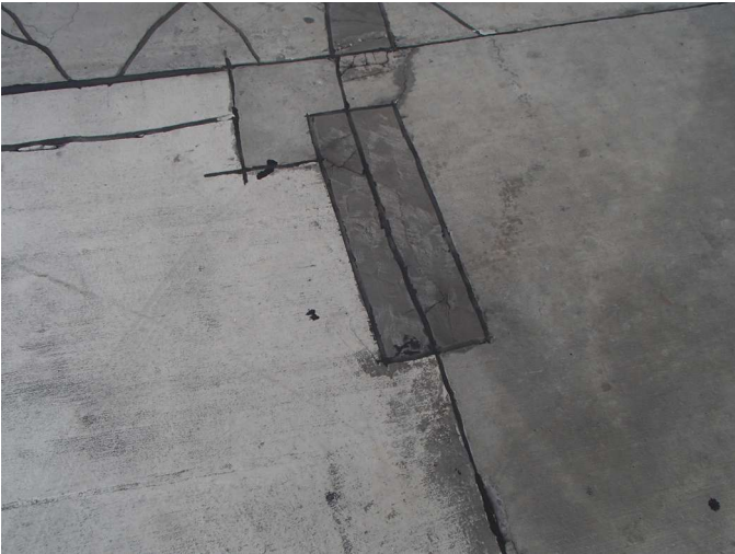
Fig. 6: Example of monitoring for replacement of deteriorating concrete repair where past repairs are critical to extending the long-term service life of the structure
