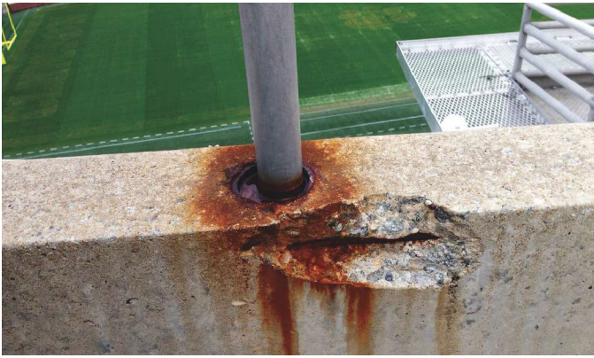
Fig. 5: Typical concrete and handrail damage that occurred over time
