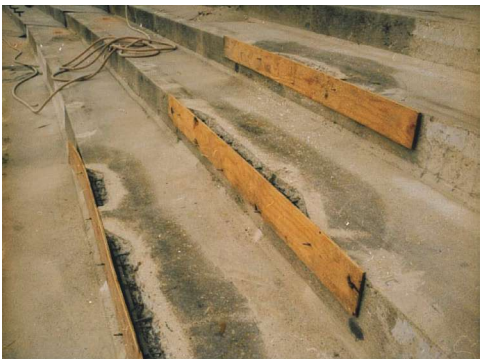
Fig. 9: Forming concrete risers for repair material installation
