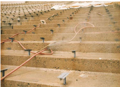
Fig. 8: The required substrate moisture conditions were achieved by soaking for 24 hours
