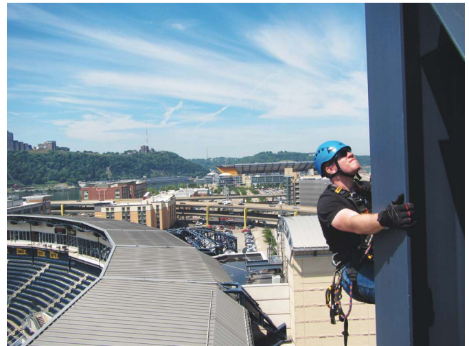
Fig. 2: Rope access was used to visually review lighting mast steel connections close up
