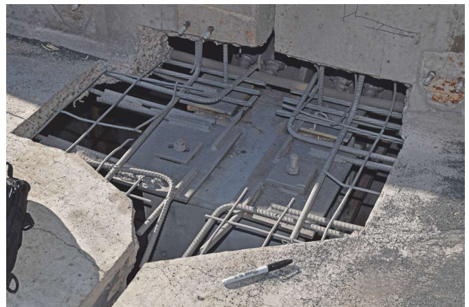
Fig. 9: Typical precast joint repairs—seismic restraint plate (embed with bolt) and precast bearing seat assembly (below prestressing strands) after existing plates replaced, rebar welded back, and sandblasted prior to epoxy coating and pour back.
