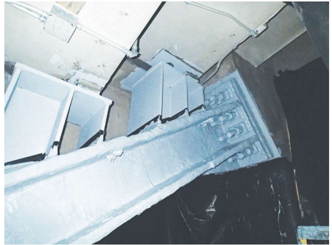
Fig. 7: Raker truss tieback anchor connection—completed repair with epoxy intumescent fireproofing to achieve 3 hour fire rating and provide corrosion protection to the beam and threaded rebar anchors.
