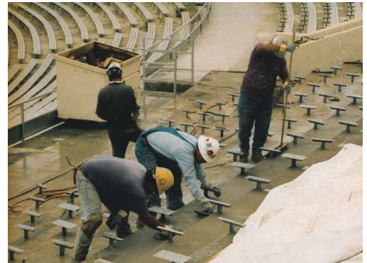
Fig. 11: Team approach—resurfacing, finishing, and curing
