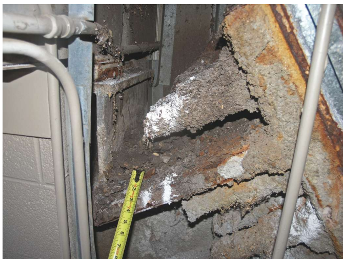
Fig. 5: Threaded rebar anchor—large mound at end of tape measure is peanut shells and debris washed through failed joint above.
