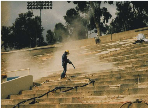
Fig. 6: High-pressure water blasting to clean and prepare concrete surface
