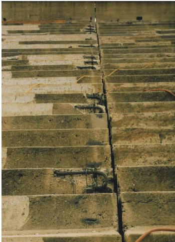
Fig. 7: Areas of prepared and un-prepared concrete
