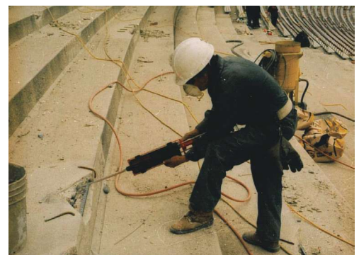
Fig. 5: Removing damaged concrete with chipping hammer
