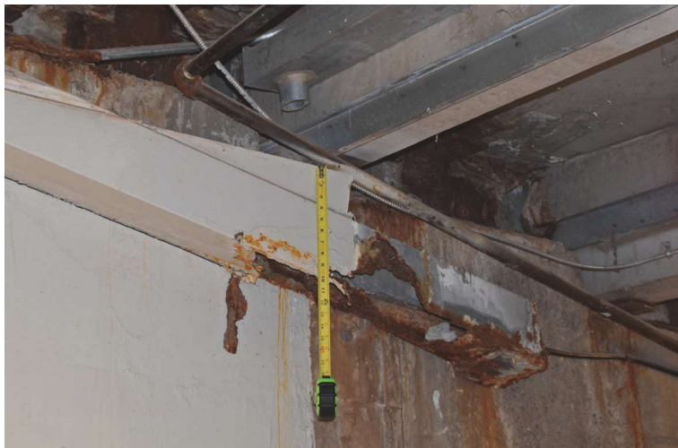
Fig. 2: Bottom side of seating riser at support—seating riser bearings and seismic restraint plates are visible on the bottom side. Moisture penetration through building expansion joint into mineral wool (each side of L-shaped plate) resulted in severe corrosion. Rain gutter system completely corroded through as it enters uninhabited space.
