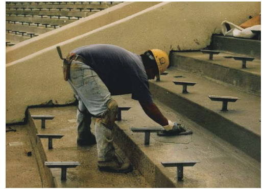
Fig. 10: Resurfacing concrete
