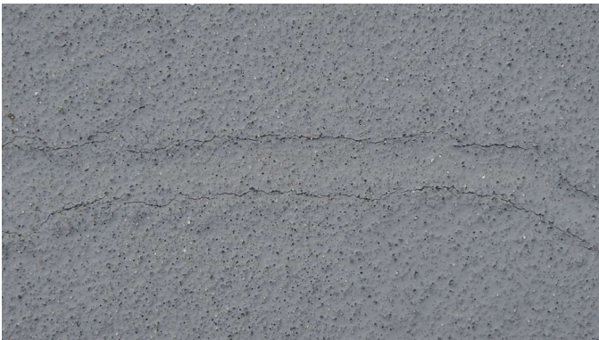
Fig. 7: Example of failing traffic coating spanning over a crack that when identified promptly for repair will improve the performance of this critical protective system
