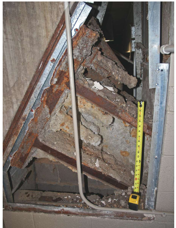
Fig. 3: Raker truss tieback anchor—connection between steel raker truss and concrete frame with sixteen 1-3/8" (35mm) diameter high strength threaded rebar anchor rods. Connection is completely hidden between two masonry walls in a dead space with leaking precast joint directly above. Spray-applied fireproofing absorbs water and never dries out.
