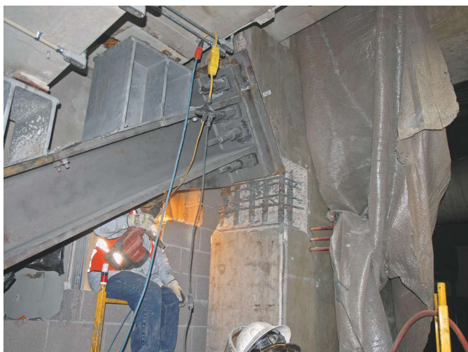
Fig. 6: Raker truss tieback anchor connection—overall view of the threaded rebar anchor assembly after initial sandblasting.
