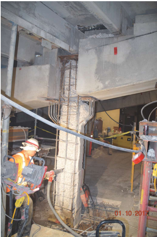
Fig. 10: Concrete column repairs—due to placement logistics, the contractor elected to repair this column rather than replace it.
