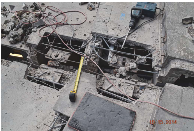
Fig. 11: Typical Precast Joint Repairs - Water leaking through building expansion joint between precast seating sections was absorbed by mineral wool fireproofing in the joint, resulting in severe deterioration. Large steel plates are seismic restraints.
