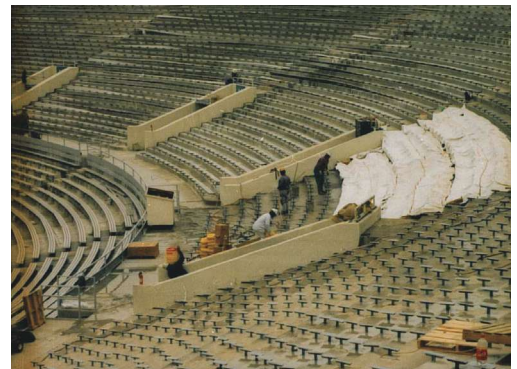
Fig. 12: Large repair areas were cured with saturated curing blankets
