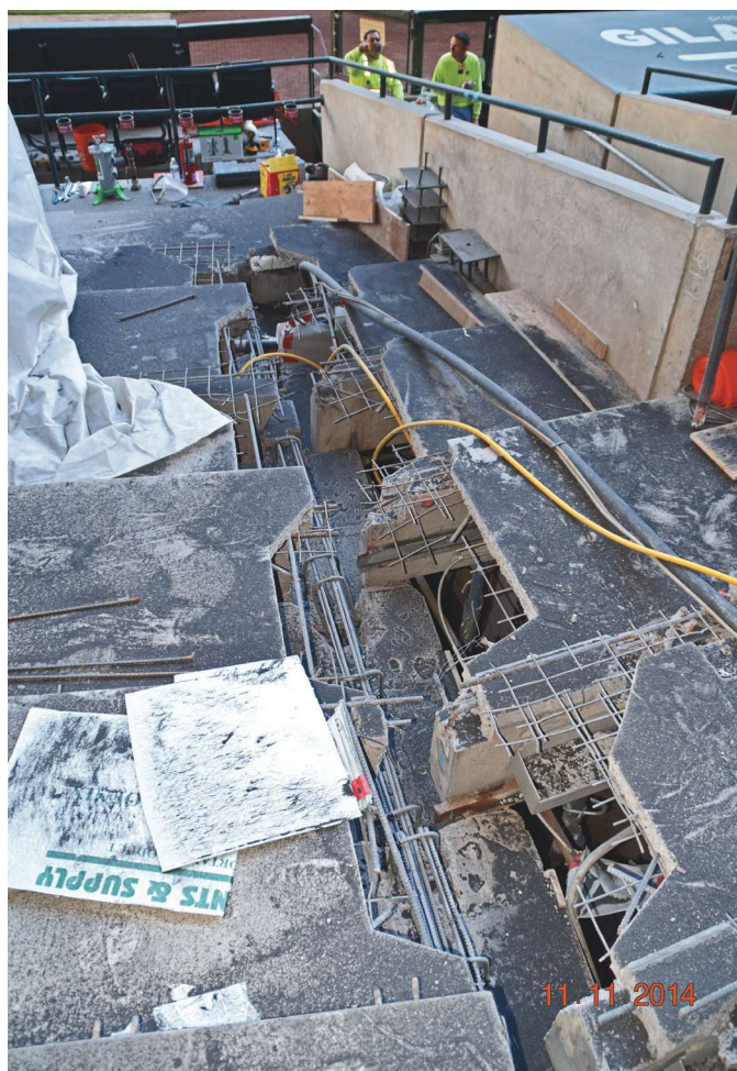
Fig. 12: Precast joint repairs—typical example of demolition required to repair the joints between the precast seating sections. Seismic restraint plates have been completely removed for replacement. Bearing repairs for stems have not started. Virtually every row was affected.
