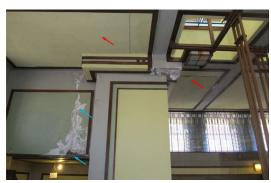
Fig. 3: Concrete deterioration of concrete beam (blue arrows) and water damage to plaster finish at interior of Unity Temple Sanctuary—roof slab underside delaminations were removed and covered with plywood (red arrows) to address potential falling hazards prior to restoration
