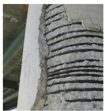
Fig. 2: Column deterioration during the bridge inspection
