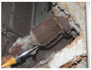
Fig. 4: Threaded rebar anchor nut—Severe deterioration of the nut. Corrosion of the threaded anchor rod is not visible due to fireproofing and debris.
