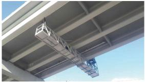
Fig. 6: Protective coating installation at bridge underside
