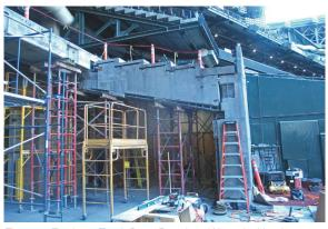
Fig. 10: Elephant Trunk Door Repairs—Water leaking between the door and precast resulted in severe corrosion, requiring emergency shoring during the baseball season.
