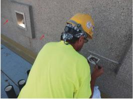
Fig. 7: Routed and sealed construction joint repair (arrows point to completed joint repair)—crack repair was similar
