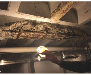
Fig. 2: Concrete deterioration at existing concrete beam.
