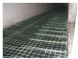
Fig. 9: Steel reinforcement for new pan-joist system (Phase 1)
