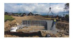
The Superior Walls Xi Plus wall systems selected by the Hermitage Club construction team include one-inch foam insulated concrete studs and one-inch foam insulation on the bond beams to
