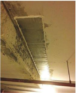
Fig. 7: Sacrificial zinc sheet at slab soffit
