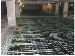
Fig. 10: Steel reinforcement for new pan-joist system (Phase 2)
