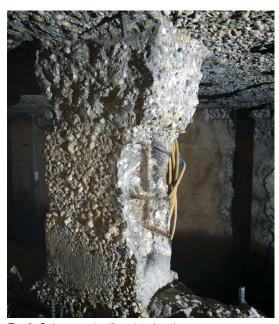
Fig. 2: Column and ceiling deterioration
