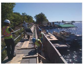
Fig. 6: Placing deck concrete
