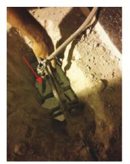
Fig. 3: Electrical conduit (red arrow) and PT cables from top of slab
