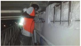
Fig. 5: Concrete repairs performed from swinging platform
