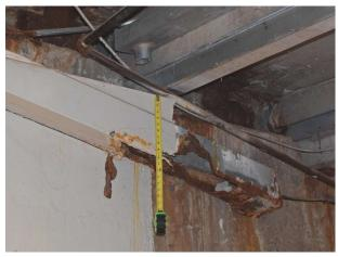
Fig. 2: Bottom side of seating riser at support—seating riser bearings and seismic restraint plates are visible on the bottom side. Moisture penetration through building expansion joint into mineral wool (each side of L-shaped plate) resulted in severe corrosion. Rain gutter system completely corroded through as it enters uninhabited space.
