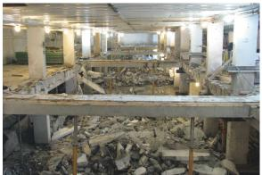
Fig. 6: Demolition and temporary lateral bracing in Phase 2
