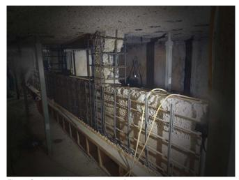
Fig. 4: Overlay reinforcement at overflow weir
