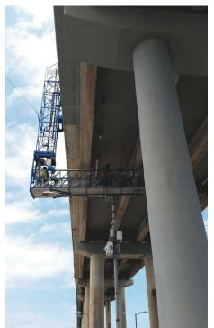
Fig. 4: Swinging platform to perform spall repairs and apply coating
