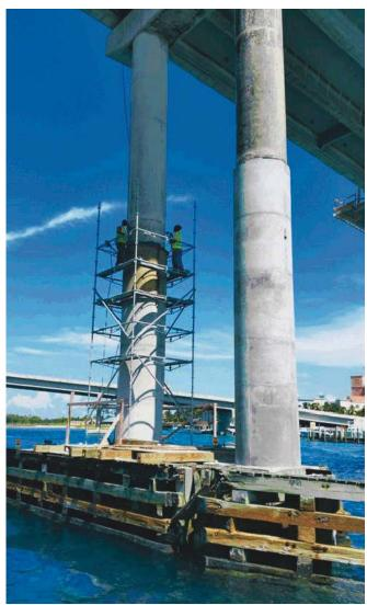
Fig. 3: Repair work at one of the columns
