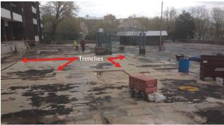
Fig. 5: Plaza demolition revealed topping slabs that overlaid the structural deck
