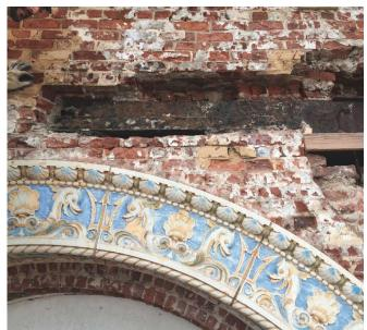
Fig. 3: Steel deterioration near window openings
