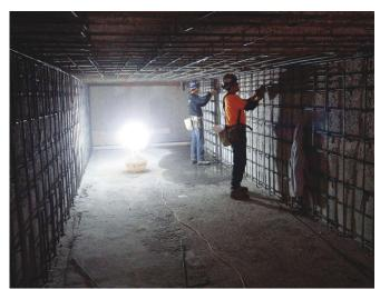
Fig. 3: Reinforcing installation within channel
