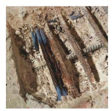
Fig. 4: Localized corrosion in previous concrete repair
