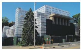
Fig. 5: Weather enclosure at front (north) elevation of Unity Temple during restoration
