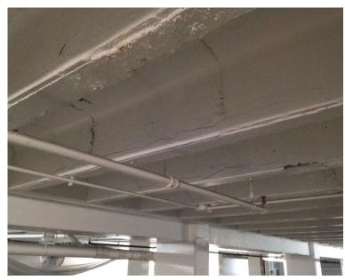
Fig. 1: Concrete deterioration at existing concrete joist.
