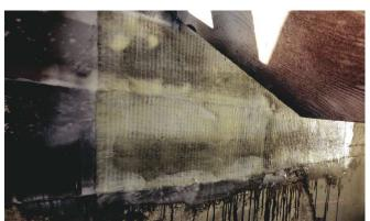
Fig. 9: Repair application of FRP at horizontal joint prior to new parge coat
