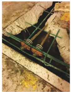
Fig. 8: New encapsulated PT anchors at expansion joint
