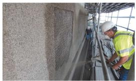
Fig. 6: Localized exterior wall repair using wet-process shotcrete
