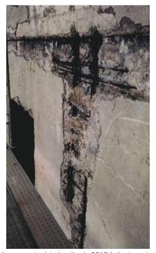
Fig. 6: Exterior concrete deterioration in 2016 (prior to restoration)
