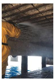
The repair program included the following items: Cementbased rustproofing, with migrating corrosion inhibitor, was applied to protect steel surfaces. Deteriorated concrete was
