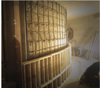
Fig. 5: Wall liner, reinforcement, and formwork
