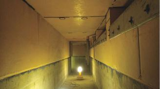
Fig. 8: Nearing completion of overlay and HDPE liner assembly at overflow weir
