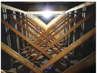
Fig. 6: Formwork and bracing
