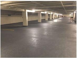
Fig.11: Vehicular traffic-bearing waterproofing (VTBW) system installed on Level G1
