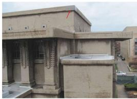
Fig. 2: Concrete cracking and deterioration on exterior walls and cantilevered roof slabs—loose spall at corner of parapet wall (arrow) was removed and covered to address potential falling hazard prior to restoration
