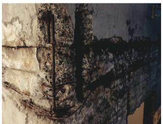
Fig. 8: Cold joint revealed during parge coat demolition
