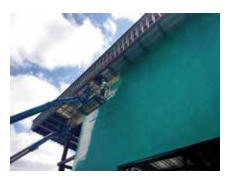
AIR-SHIELD TMP has been specifically formulated to act as an air and liquid moisture barrier, allowing vapor to pass through it. It may be applied to most common surfaces and integrated into various wall systems. AIR-SHIELD TMP is suitable for both new construction and retrofit applications.
