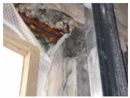
Fig. 9: Rusted rebar caused spalling at window lintel
