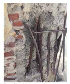
Fig. 5: Spalled concrete column at northwest corner
