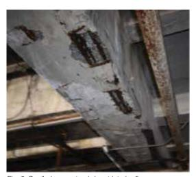
Fig. 6: Spalled concrete girder at interior floor
