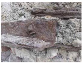
Fig. 7: Corroded shelf angles supporting terra cotta veneer
