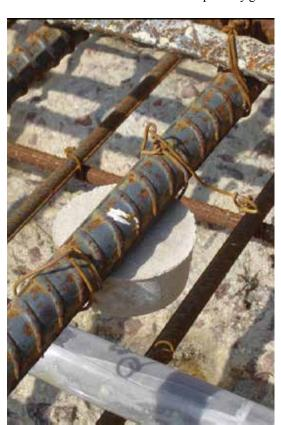
Fig. 3: Sacrificial anode installed within concrete repair area
