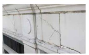
Fig. 3: Cracked terra cotta above windows at north face
