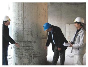
Fig. 3: Poor condition of concrete column
