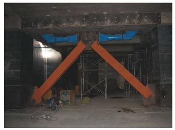
Fig. 6: Inverted V-bracing with viscous dampers
