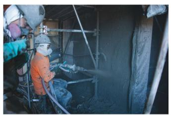
Fig. 5: FRCM application over the prepared surface
