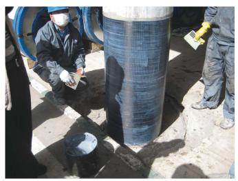
Fig. 8: CFRP confinement of column
