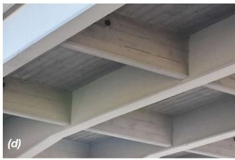
Fig. 6: Installation of titanium bars on Mosier Bridge: (a) Cutting of groove; (b) Inserting epoxy in the groove; (c) Inserted titanium bar in the prepared groove; (d) Completed install (photos courtesy of ODOT)
