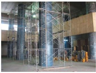
Fig. 7: Columns at lobby wrapped by CFRP
