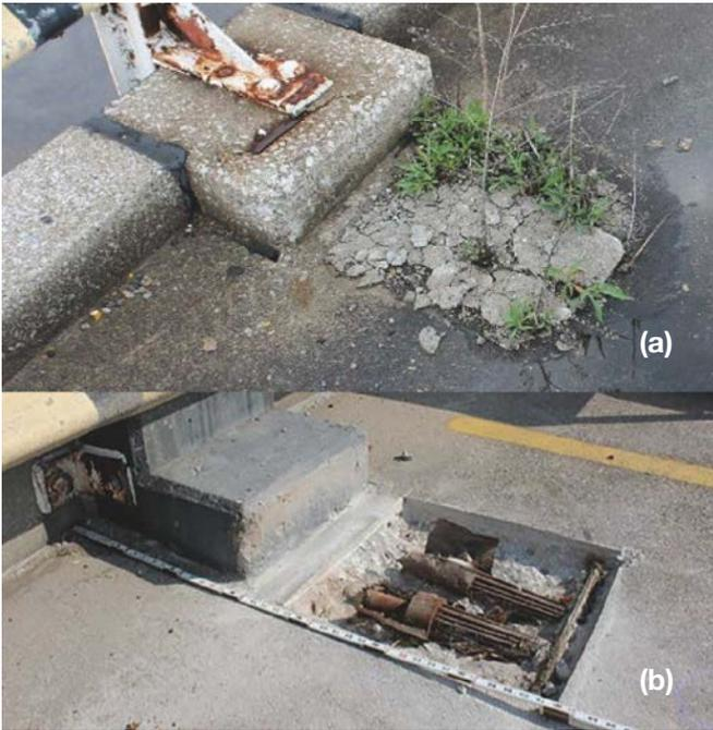
Fig. 5: (a) Many grout pockets on the roof were delaminated and some had vegetation growing, and (b) Grout pocket after concrete removal and cleaning
