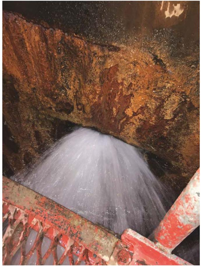
*Fig. 2: Major water penetration points were blasting masses of water 12 in (300 mm) wide across the 23 ft (7 m) diameter of the shaft. The extreme pressure of the water was causing damage to the shaft structure and made the repair a very dangerous project.*
