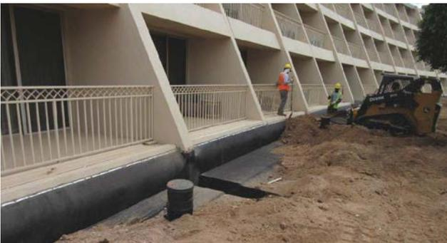
Fig. 7: Foam blocks and backfilling in progress after completion of waterproofing repairs along the expansion joint
