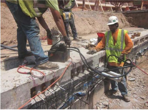
Fig. 5: Post-tension repairs in progress (stressing end)
