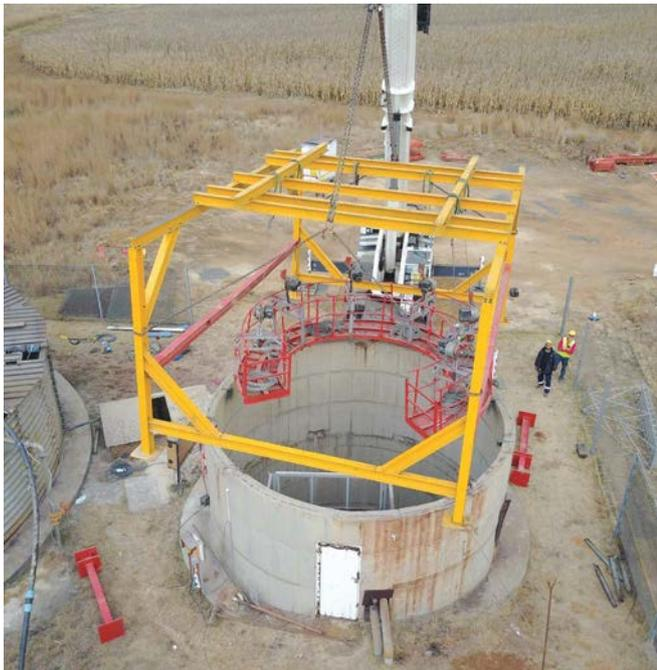
Fig. 3: Access to the shaft was a huge safety and logistical concern. The access specialists were able to supply a custom-built cradle to lower workers into the shaft. This cradle was anchored to the sides of the shaft to ensure no movement during the high-pressure cleaning and sandblasting.
