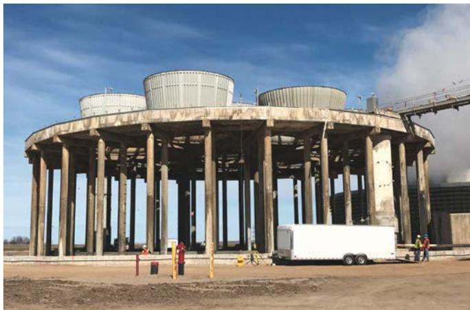
following May. A visual inspection and sounding survey was conducted to identify defects, estimate quantities of repair, develop a repair strategy, and to create a detailed project schedule.
