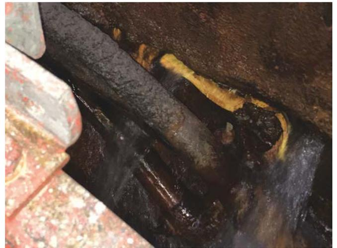
Fig. 5: The waterproofing specialists tested the swelling waterstop on the ingress points to ensure the waterstop would swell to its maximum capacity to alleviate water pressure to continue with the crystalline leak repair system.
