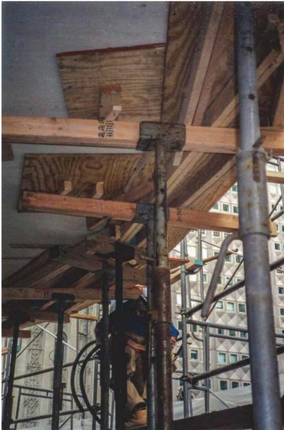
Fig. 6: Slab edge formwork and shoring
