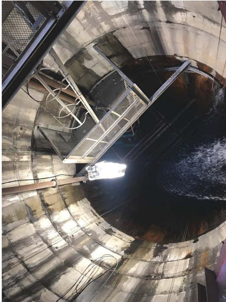
*Fig. 1: View from the top of the shaft during the site inspection. The extreme water ingress points are evident all the way down the ventilation shaft. The base of the ventilation shaft was filled with water for 35 years.*
