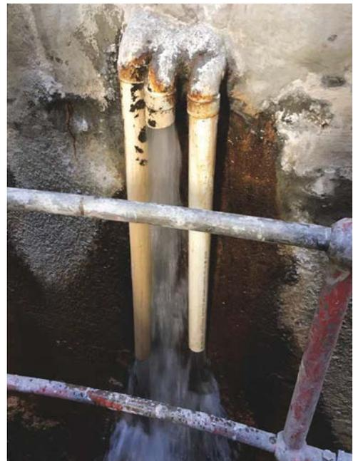
Fig. 6: Using a rapid-setting hydraulic cement and a swelling waterstop, the waterproofing specialists were able to successfully contain the flow of water to a single access point, thus making the water more manageable.
