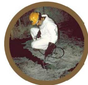
Azo-Grout™ by Azon, is a diverse family of polyurethane-based waterstop products used for concrete crack repair, stopping water infiltration and soil stabilization
