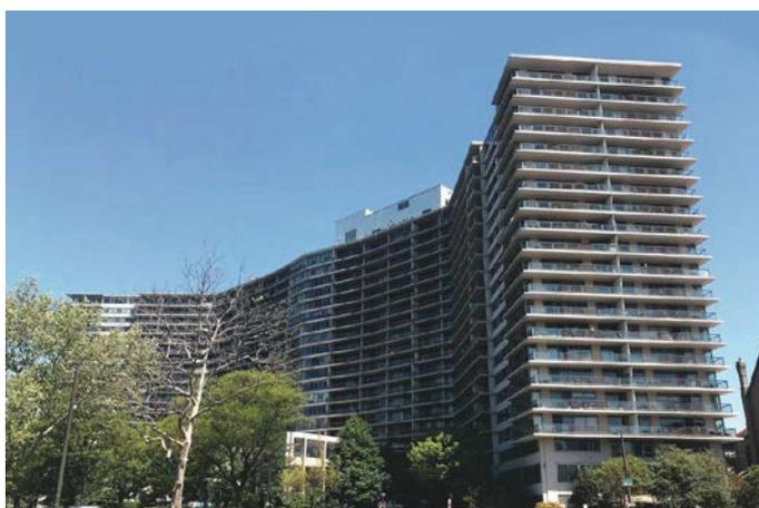
The owner has done a good job maintaining this building. In 2013, a façade inspection indicated cracks and concrete spalls in some of the balconies, eyebrows and columns. Further evaluation of the balconies indicated the handrails were structurally deficient due to post pockets containing gypsum grout. This dramatically increased the scope of work.
