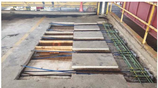
Fig. 4: Placement of new PT anchors
