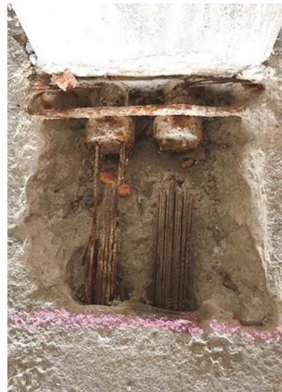
Fig. 3: Many beams were observed to have completely corroded through tendons
