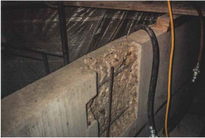
Fig. 8: Knee wall vertical repair demolition
