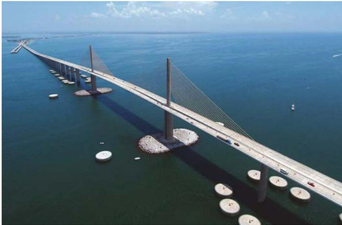
190 ft (58 m). Built at a cost of US \$244 million, it opened to traffic in 1987. The current cable stay bridge is a replacement for the previous steel, cantilevered truss bridge that was tragically struck by a freighter back in 1980 when a 1,200 ft (366 m) span collapsed into Tampa Bay, killing 35 people. It took seven years before a signature replacement bridge could be built.
