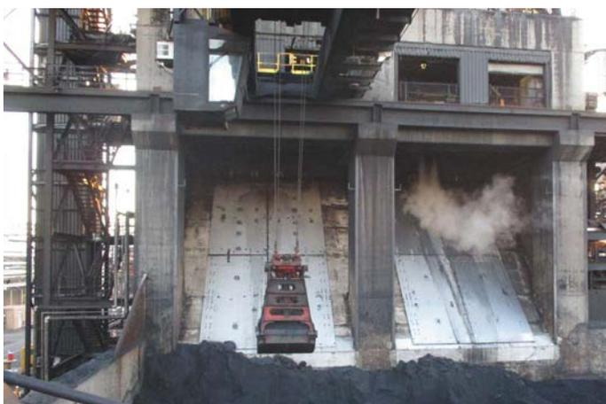
Over years of operation in this intense environment, the coking unit in a refinery in the United States was experiencing deterioration of both the steel plates and the approximate 64 x 33 ft (20 x 10 m) x 3.5 ft (1 m) thick concrete chute slab. After a comprehensive condition assessment, testing showed cracks and warps in the coking unit due to expansion of the embedded steel anchors for the plate. Although minor repairs were made in the past to the plates, an innovative floating
