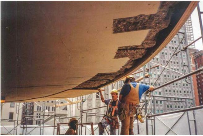
Fig. 5: Slab edge soffit demolition and formwork
