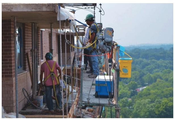
Fig. 1: Each employee is tied off to vertical ropes with rope grabs through the suspended scaffold rigging assembly
