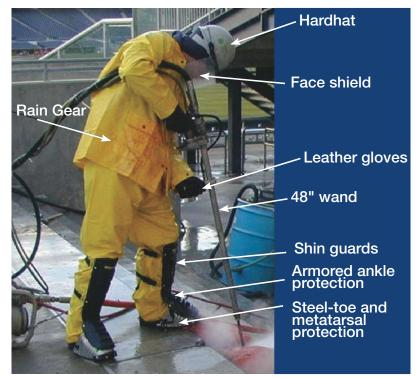
Fig. 5: Typical PPE for hand lance operation
