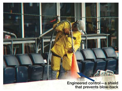
Fig. 3: Engineered control to protect operator
