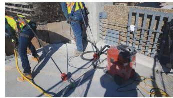
Fig. 2: Employees are tied off on 10 ft (3 m) retractable lanyards attached to a temporary horizontal cable lifeline (fall hazards are eliminated, without any freefall)
