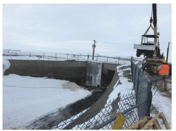
Fig. 6: Lowering materials and equipment to siphon entrance after clearing snow and ice
