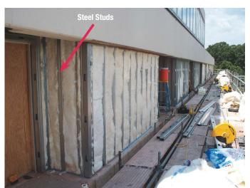
Fig. 10: Exterior wall replacement
