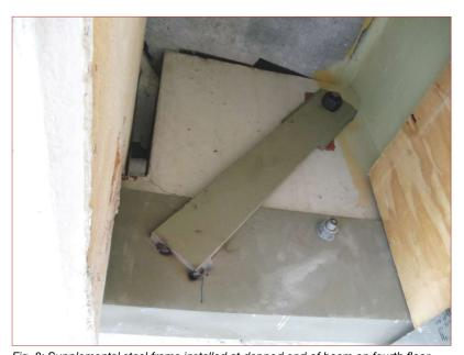
Fig. 8: Supplemental steel frame installed at dapped end of beam on fourth floor
