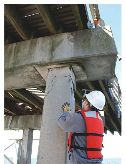
Fig. 7: Sounding at affected piles
