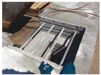
Fig. 11: Pile-beam connection prior to assembly
