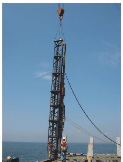
Fig. 10: Overview of driving new replacement pile
