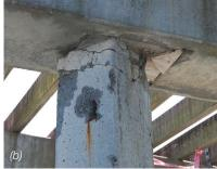
Fig. 5a & b: Views of (typical) shear failures at piles
