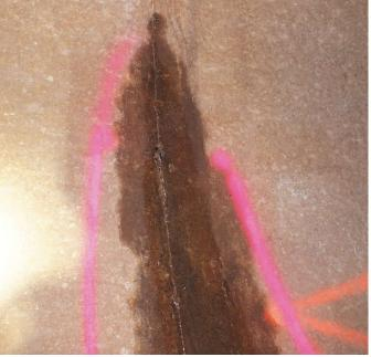
Fig. 4: Water leakage through a joint in the siphon barrel
