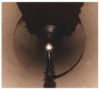
Fig. 3: Looking upstream from inside the siphon. Due to the slope of the siphon, condensation and leakage water also collects on the crown of the siphon
