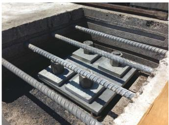
Fig. 12: Pile – beam connection after installation of threaded bars, couplers, plates, washers, and nuts
