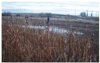
Fig. 2: Water ponding above siphon barrels
