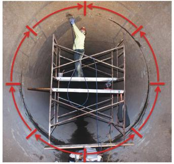
Fig. 7: Grouting sequence
