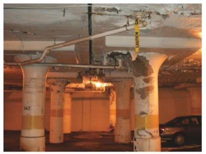
Fig. 3: Representative conditions at underside of track deck before rehabilitation
