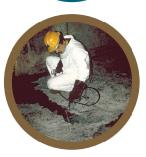
Azo-Grout™ by Azon, is a diverse family of polyurethane-based waterstop products used for concrete crack repair, stopping water infiltration and soil stabilization
