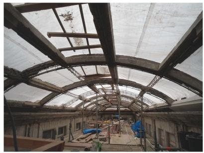
Fig. 2: Concrete repair and corrosion mitigation of concrete atrium arches and beams at James Ensor Gallery (Ostend, Belgium)
