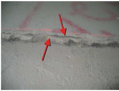
Fig. 3: Overlays of varying thickness covering the top surface of the structural slab
