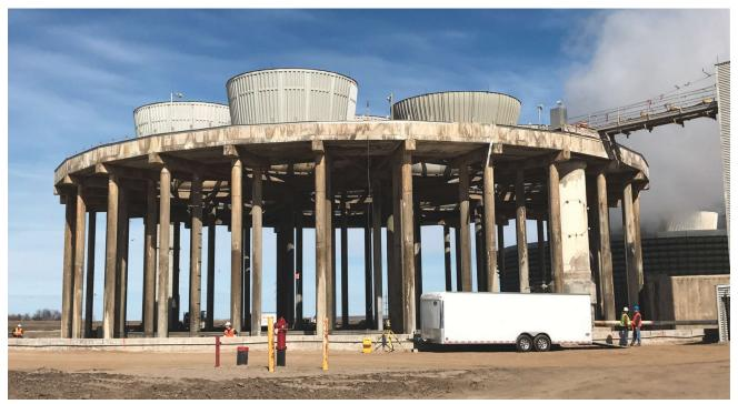
Fig.1: Concrete repairs, strengthening, and protection of concrete cooling towers (North Dakota)
