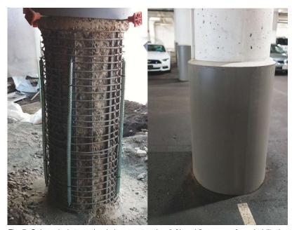
Fig. 7: Column jacket repairs during construction (left) and five years after rehabilitation (right)
