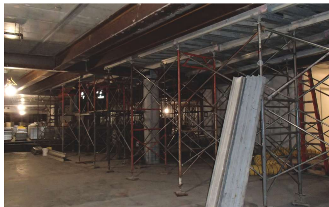
Fig. 5: Structural steel and shoring below opening
