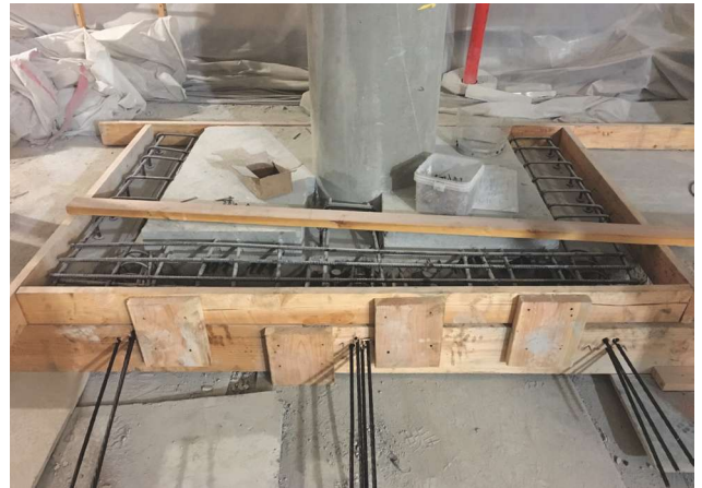
Fig. 9: Multihead anchor within slab thickening at column locations
