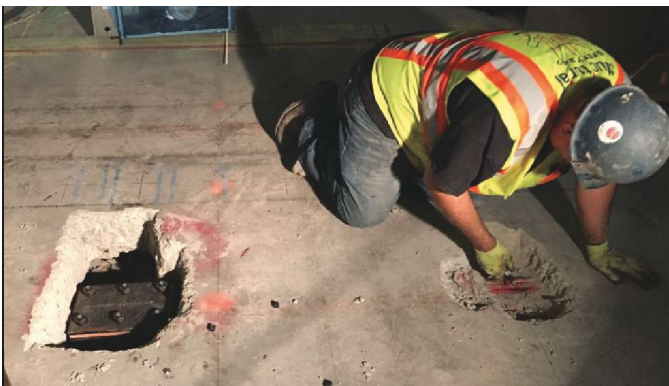
Fig. 7b: Lockdown device installed prior to detensioning
