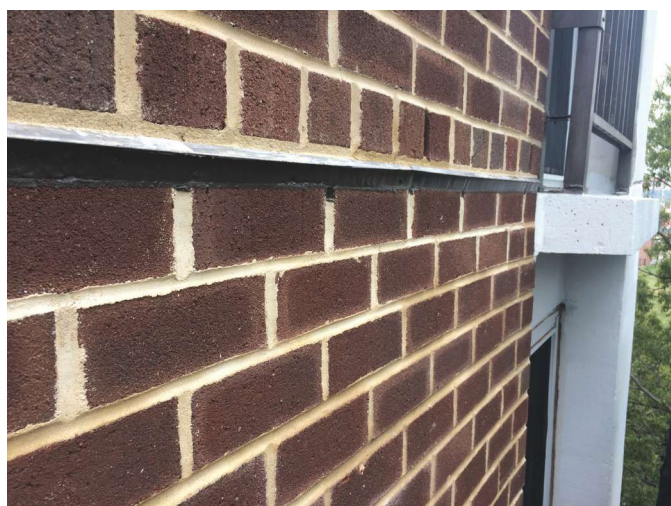
Fig. 6: Shelf angle installation after repairs and waterproofing
