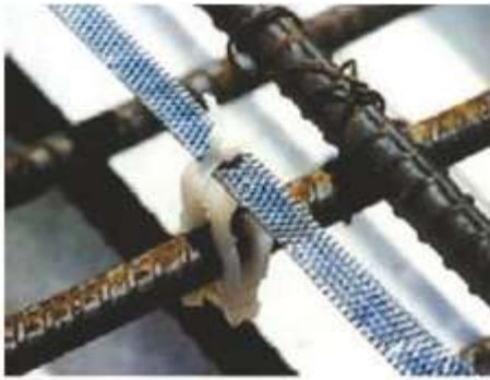
Fig. 2: Expanded mesh anode ribbon installed
