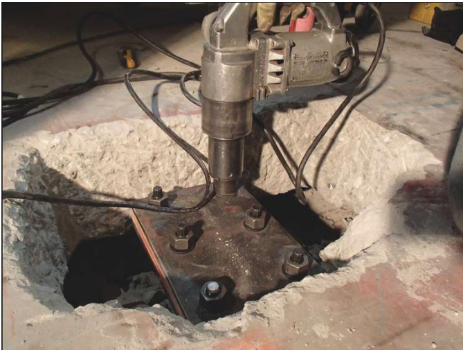
Fig. 7a: Installation of lockdown device
