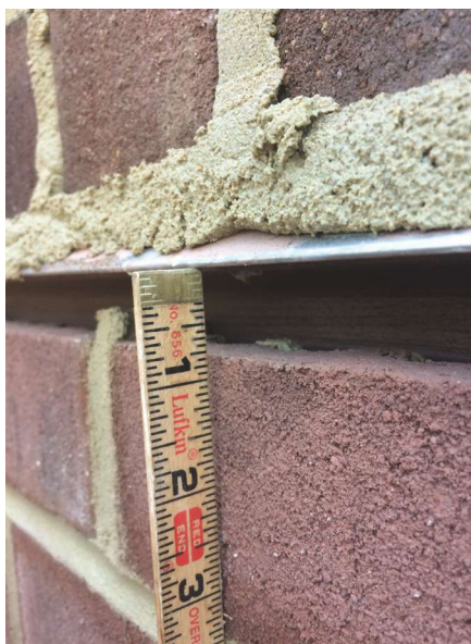
Fig. 5: Joint spacing is provided for movement
