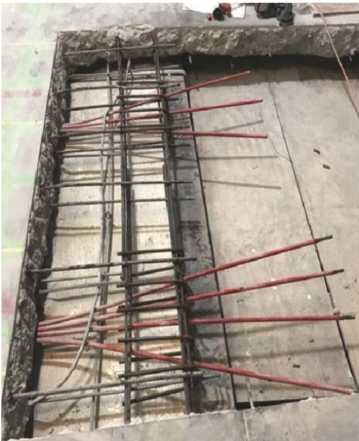
Fig. 8: Phase 1 post-tensioned tendons within new anchorage zone
