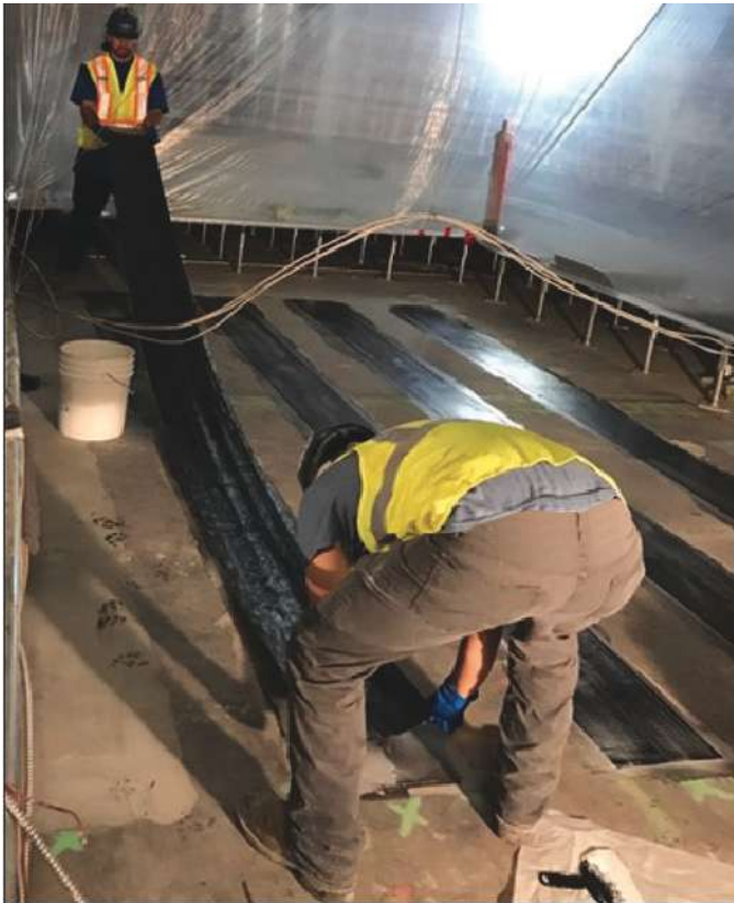
Fig. 6: Topside FRP installed at deficient bending location
