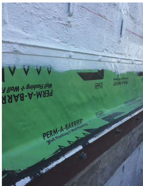
Fig. 4: Waterproofed shelf angle and masonry substrate
