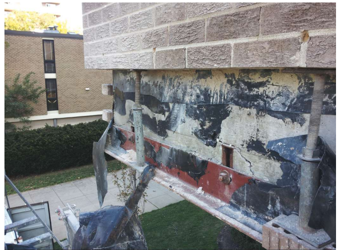
Fig. 2: Shear failures at anchor embeds
