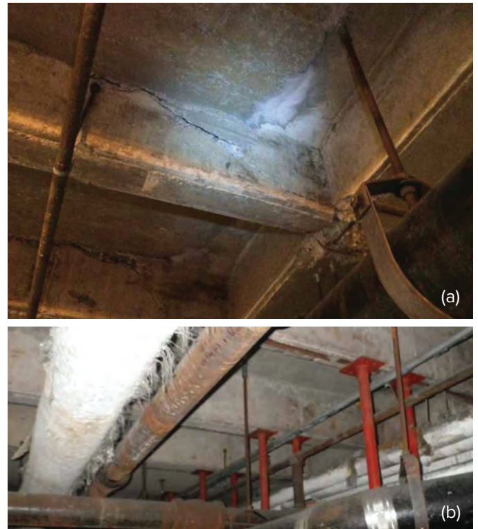
Fig. 5: Observed unsafe condition (a) and shoring used to temporarily address the condition (b)
