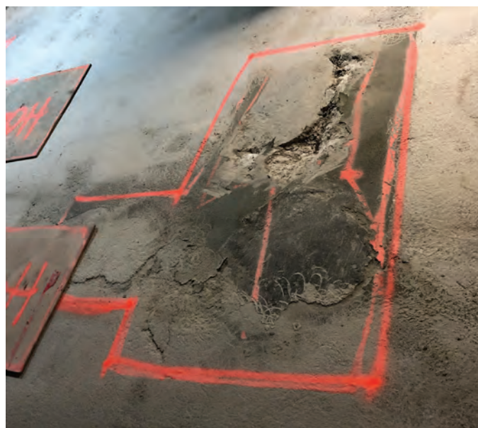
Fig. 3: Improper repair techniques can lead to continued corrosion and concrete delamination
