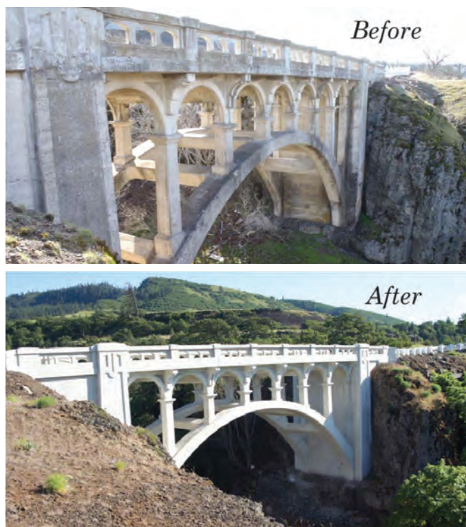
Fig. 6: Historic Dry Canyon Bridge: before (top) and after (bottom) rehabilitation
