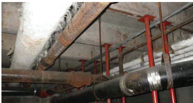
Fig. 2: Nonstructural elements may preclude the use of standard details. Shoring plans must be specific to the existing conditions (photo courtesy of Keith Kesner, CVM Engineers, King of Prussia, PA)
