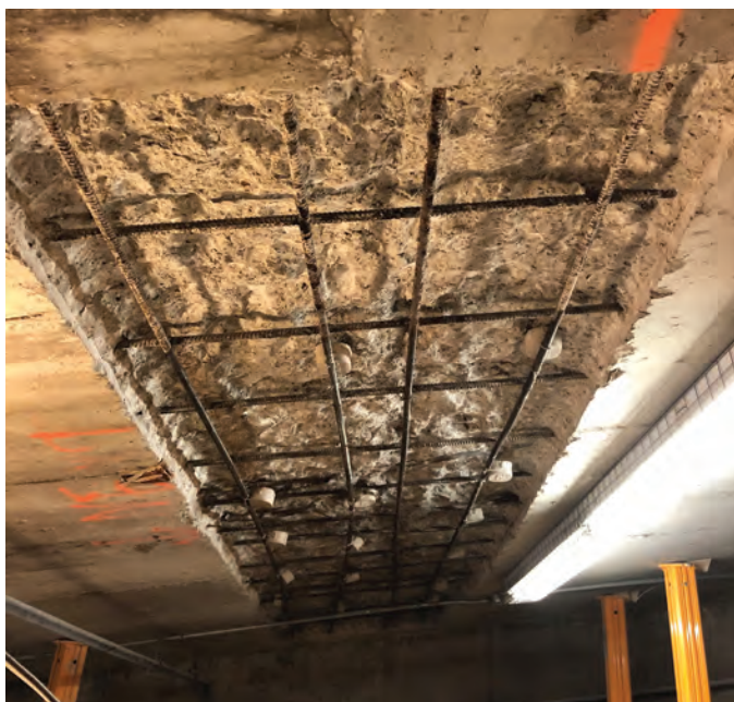
Fig. 4: Properly detailed concrete removal per ICRI 110.1/310.1R 20 and ACI 546 21 /563 with completion of concrete repairs per ACI 562 to improve durability and service life (Goals #2, #3 and #4)
