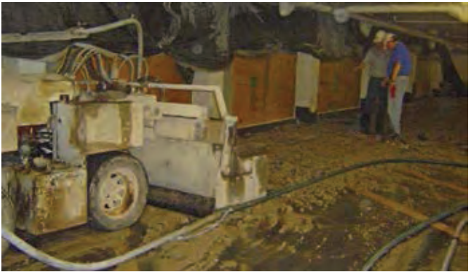
Fig. 2: Removal of 3-1/2 in. of slab by hydrodemolition (Fig. 7.2b from Reference 4)
