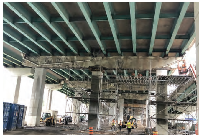
Fig. 2: Repair and galvanic encasement of deteriorated columns has been completed and scaffolding is being installed to facilitate repair and protection of the deteriorated pier caps
