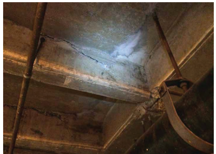
Fig. 1: Shear cracks in a one-way joist system are examples of substantial structural damage (unsafe conditions) that must be identified in the basis of design report (photo courtesy of Keith Kesner, CVM Engineers, King of Prussia, PA)
