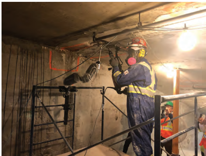
Fig. 5: Use of proper personal protective equipment (PPE) and ergonomic tools improve worker health and safety by reducing exposure to silica and repetitive stress injuries (Goal #6)
