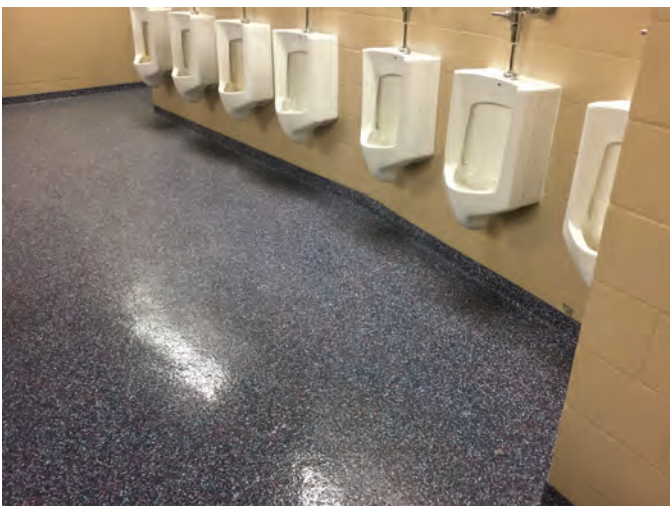
Fig. 13: Restroom floors after installation of resinous waterproofing with flake finish
