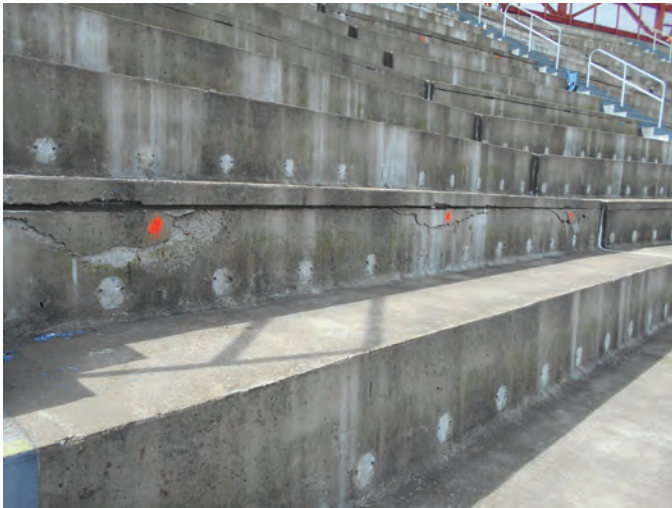
Fig. 8: Failed sealants and distressed precast connections as observed after seat removal as part of the concurrent work
