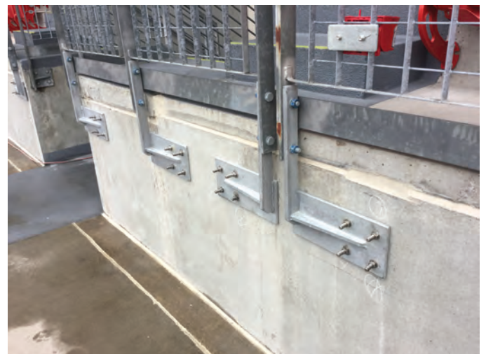
Fig. 7: Modified guardrail anchorages and new silicone sealants
