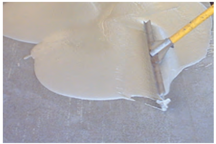
Fig. 3: Applying base coat
