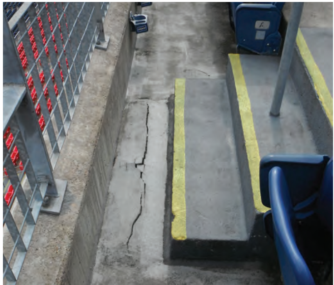
Fig. 10: Example of Row A distress
