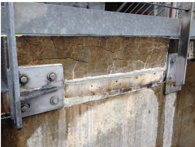
Fig. 6: Distressed concrete landings with deficient guardrail anchorage and aged sealants prior to replacement
