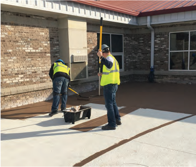
Fig. 5: Application of pigmented acrylic stain sealer
