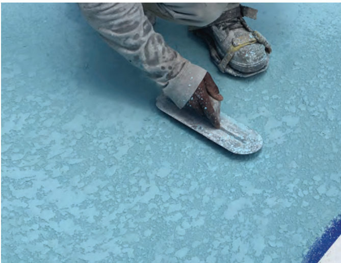
Fig. 7: Application of spray (texture) coat over color coat on multi-color project
