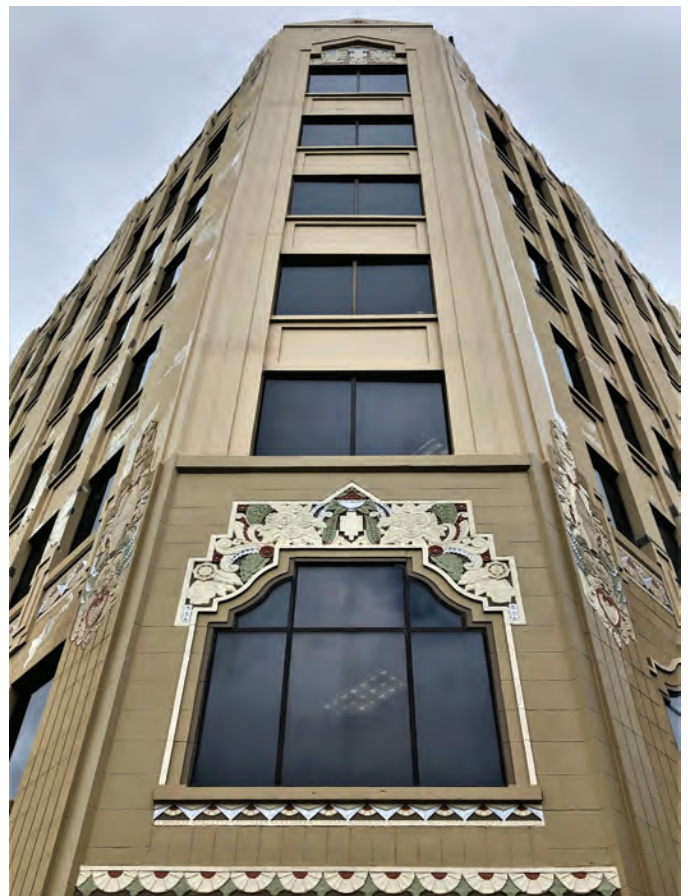
Fig. 4: Repaired elevation awaiting paint coatings
