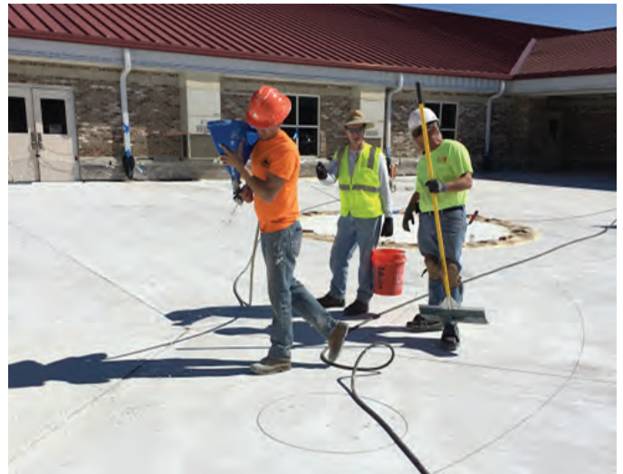
Fig. 4: Applying spray (texture) with compressor, hopper, and gun
