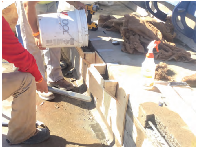
Fig. 9: Repairs in progress at upper deck (note that repairs also included installation of supplemental angles on the back of risers)
