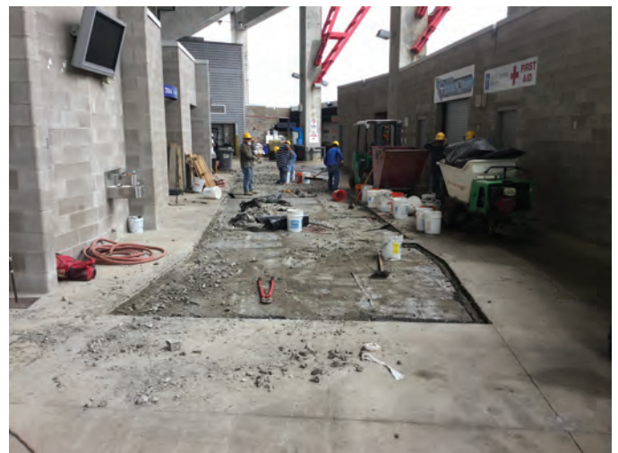
Fig. 14: Concourse slab repairs in progress
