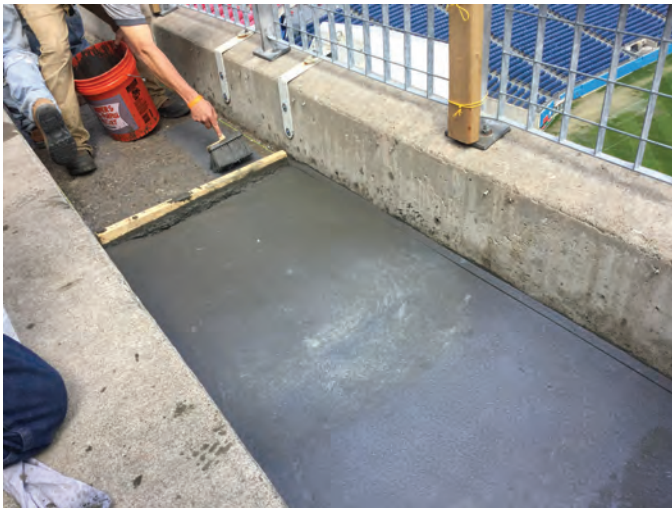
Fig. 11: Installation of scrub coat and sloped bonded overlay at Row A
