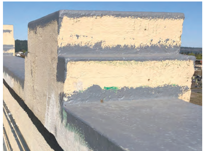
Fig. 7: Elastomeric aliphatic roof coating protecting parapet cap
