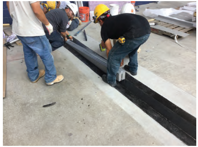
Fig. 3: Expansion joint system installation at concourse after installation of angle, adjacent concrete repair, and nosing materials
