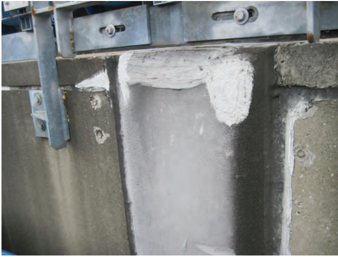
Fig. 2: Example of pre-existing expansion joint condition at upper deck
