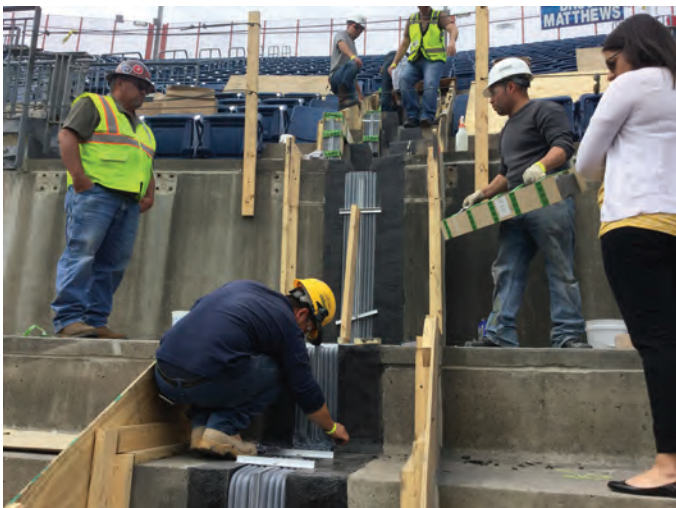
Fig. 4: Expansion joint material installation at upper deck after sawcutting and nosing installation (note removed guardrails for repairs)
