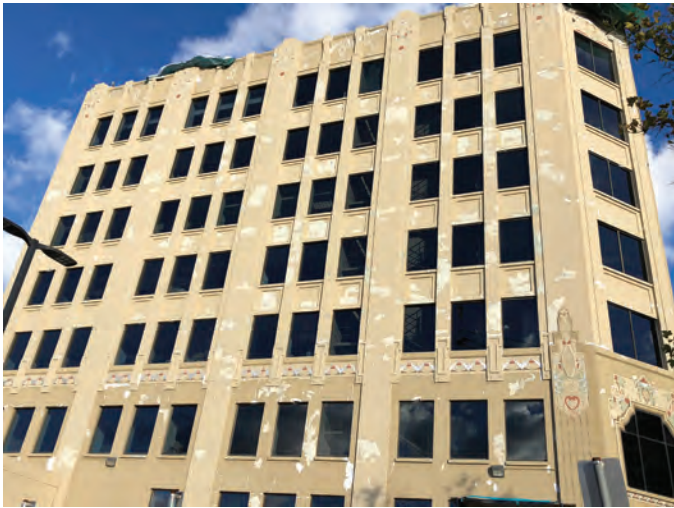
Fig. 2: Typical damage to the building prior to restoration
