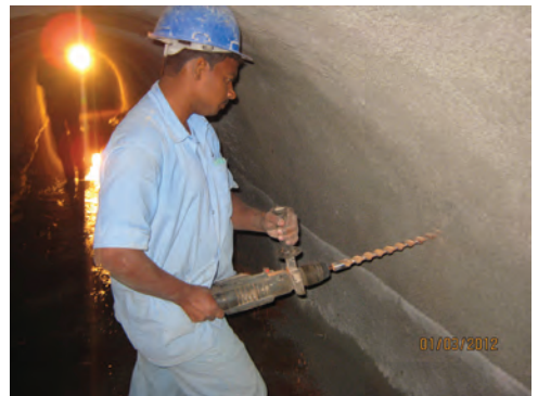
Fig. 10: Drilling holes into the brick masonry
