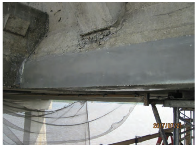
Fig. 5: Repaired girder using mortar concrete
