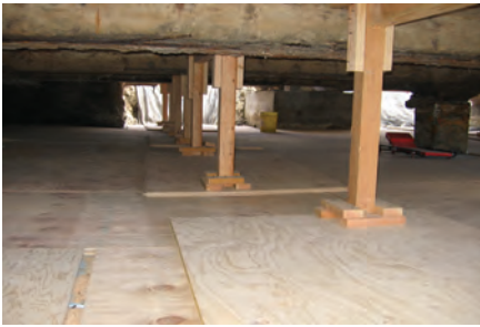
Fig. 5: Work platform and shoring installed ahead of demolition (note corroded steel throughout and the tight working conditions)
