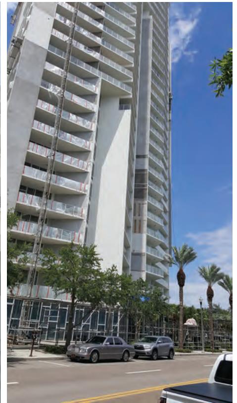
Fig. 8: Stucco replacement, CMU grouting, guardrail protection, overhead protection, and mast climber/swing stage access
