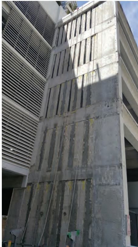
Fig. 7: Parking garage shear wall/barrier wall being reinforced
