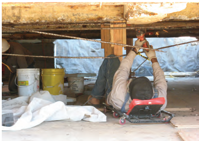
Fig. 4: A worker works off his back on a mechanics crawler to grind and clean the reinforcing steel
