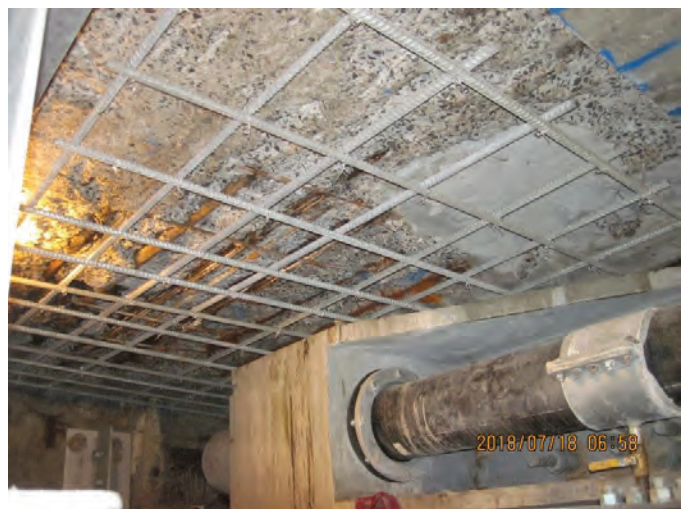
Fig. 6: Underside heavy duty slab repair prior to adding forms, concrete and steel deck and transverse beams
