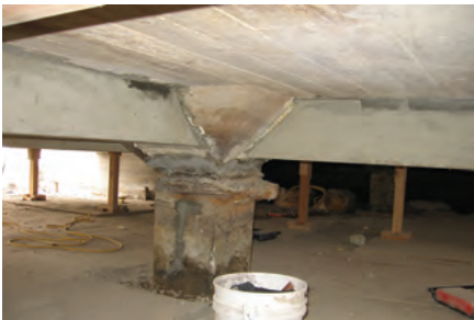
Fig. 8: Girders after concrete placement and repair
