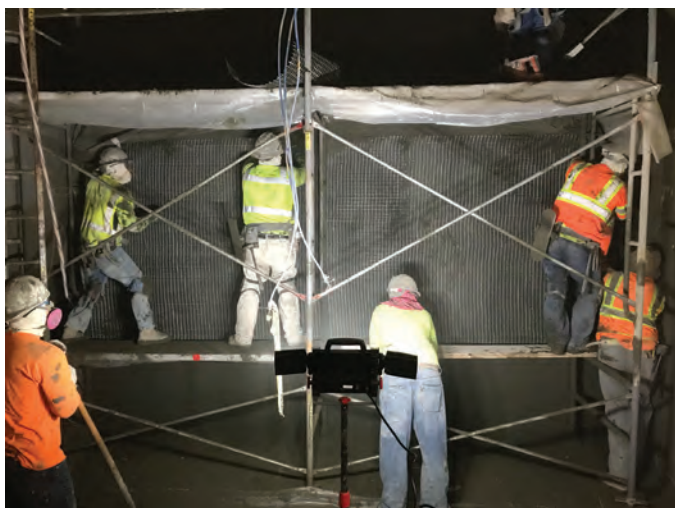
Fig. 5: Reinforcing a wall with the FRCM system
