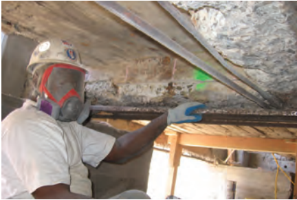
Fig. 6: Significant demolition required to remove spalled concrete and expose corroded reinforcing steel
