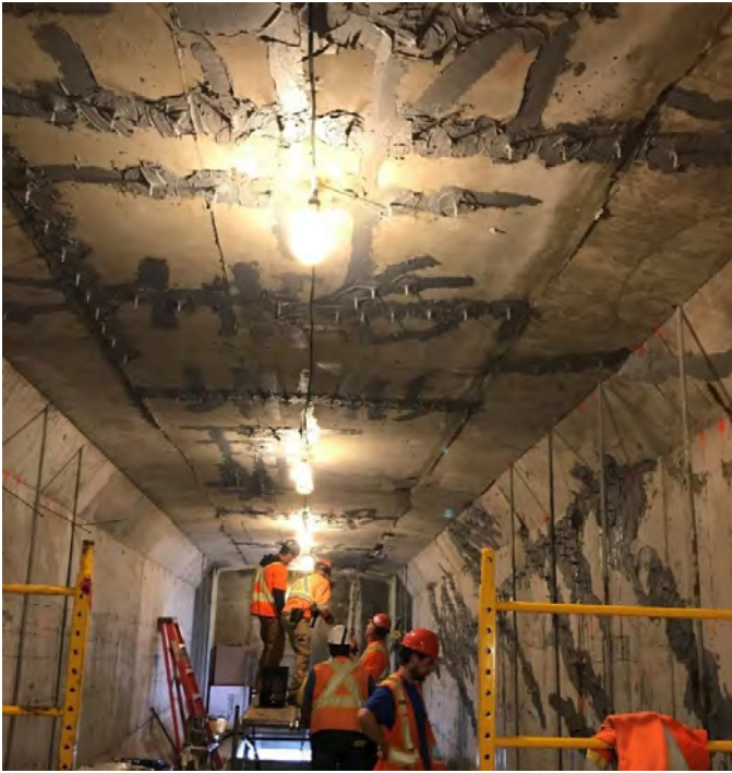
Fig. 7: Crack injection preparation
