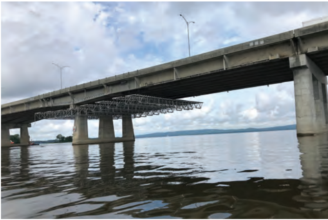
Fig. 1: Working platforms over the maritime corridor
