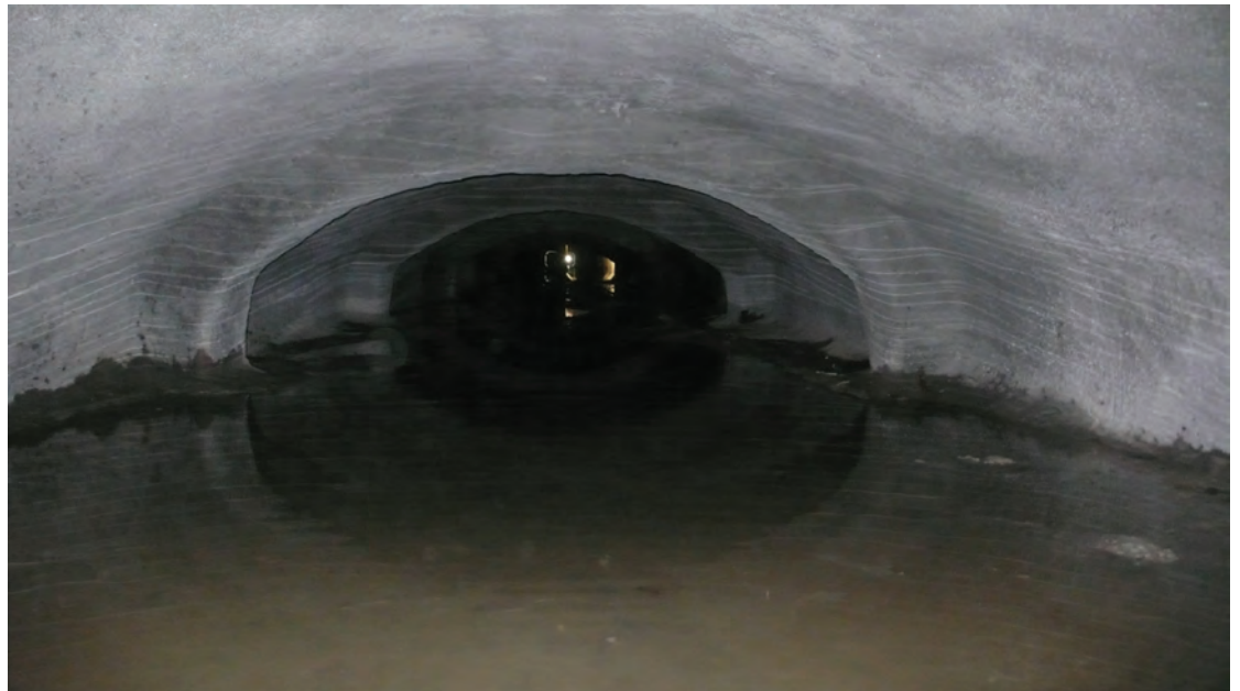
Fig. 1: Completed repair of the storm water drains in the City of Mumbai, India that are more than a century old and constructed of brick arch masonry during the British era
