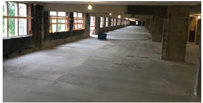
Fig. 2: Barrack slabs prepared by shotblasting before installing the crack infills and CFRP
