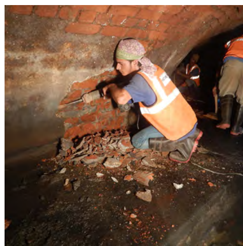
Fig. 5: Demolition of deteriorated brick lining with lightweight breaker
