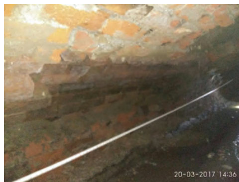
Fig. 2: Delaminated and spalling of brick lining
