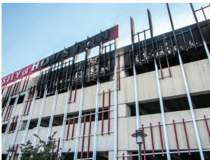
Fig. 3: Fire damage at exterior of garage
