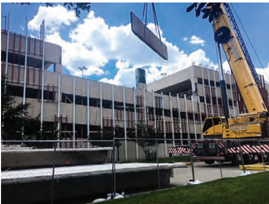
Fig. 6: Spandrel beam replacement
