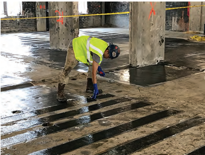
Fig. 6: Installing the final epoxy resin layer for CFRP (also performed to "knock down" any fiber edges)
