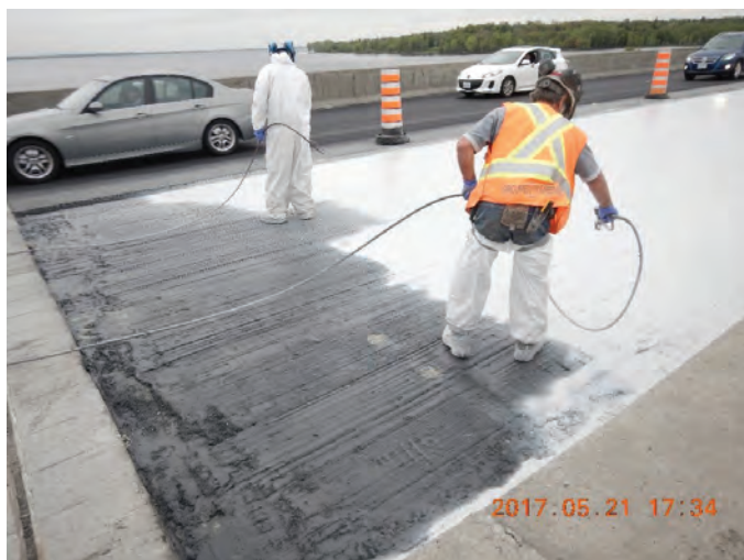
Fig. 15: Spray applied waterproofing deck membrane application
