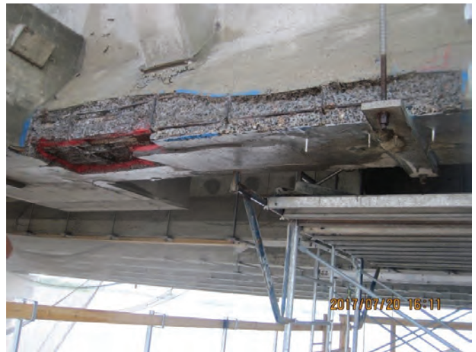
Fig. 4: Typical lower flange girder concrete demolition
