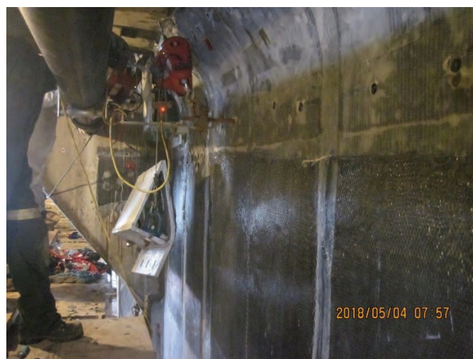
Fig. 12: Installed CFRP strips
