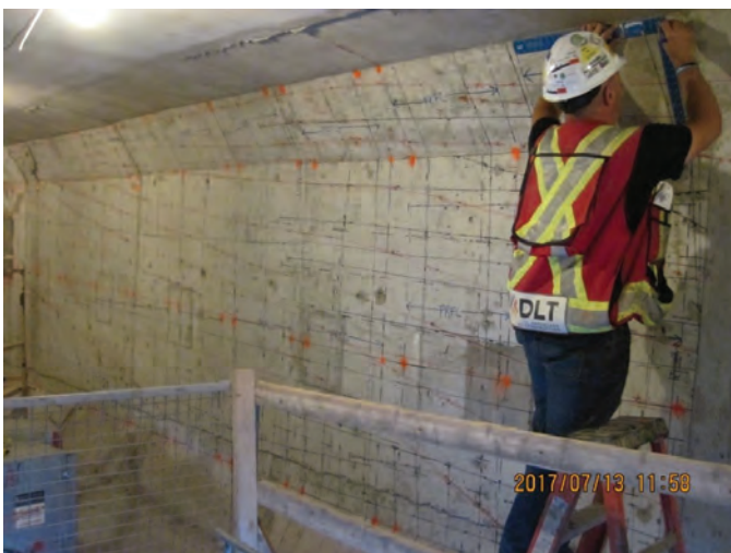
Fig. 3: Rebar and strand identification
