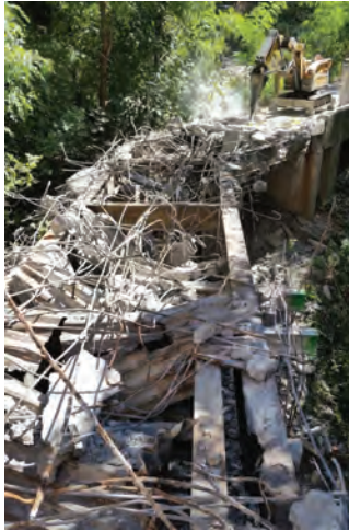
Fig. 6: Pedestrian bridge demolition
