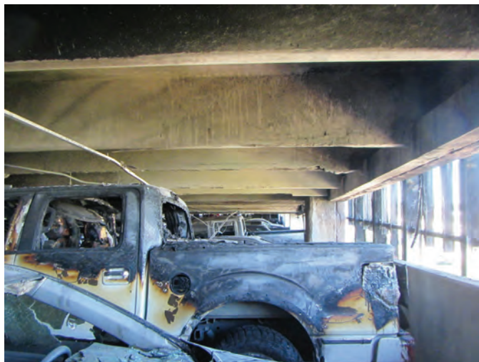
Fig. 2: Fire damage on Level 3 of parking garage
