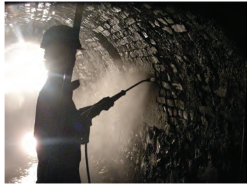
Fig. 6: High-pressure waterjet washing
