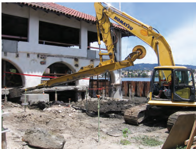
Fig. 3: Modified excavation equipment to remove the mucky soil under the supported slab
