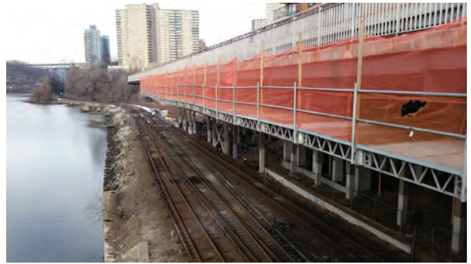
Fig. 2: Work platform suspended under the building
