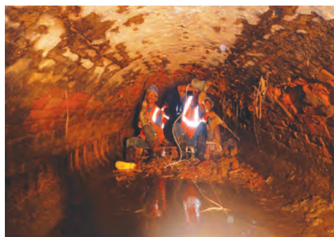
Fig. 4: Root penetration
