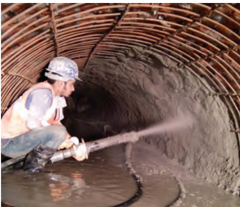
Fig. 9: Installing wet-mix shotcrete
