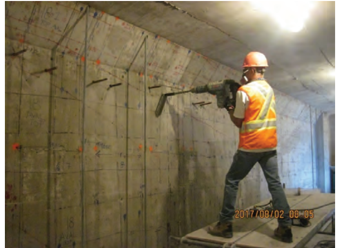
Fig. 8: Steel CFRP anchor plate horizontal hole drilling
