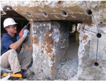
Fig. 7: Anodes installed throughout to combat the high chloride content in the concrete
