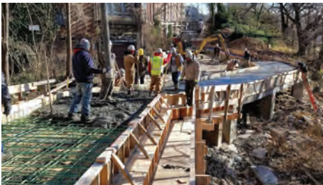
Fig. 7: Concrete placement at the pedestrian bridge
