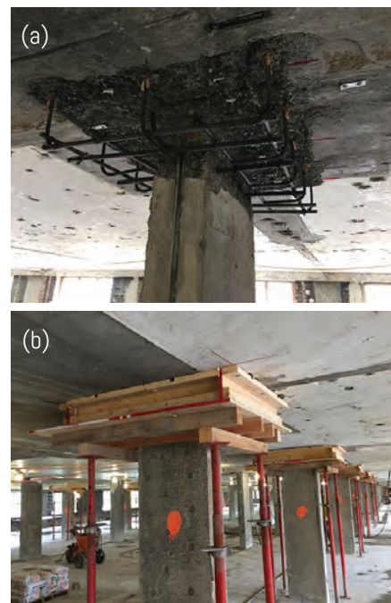
Fig. 4: Shear capital repair - (a) preparing and reinforcing the concrete surface, and (b) installed formwork prior to concrete pumping
