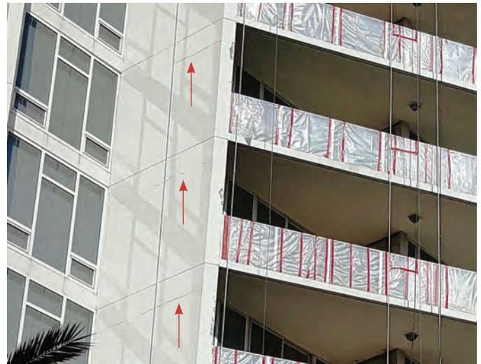
Fig. 2: Cracks in stucco on every floor at bottom of turndown beam to top of wall
