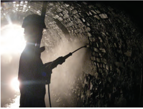
Fig. 6: High-pressure waterjet washing
