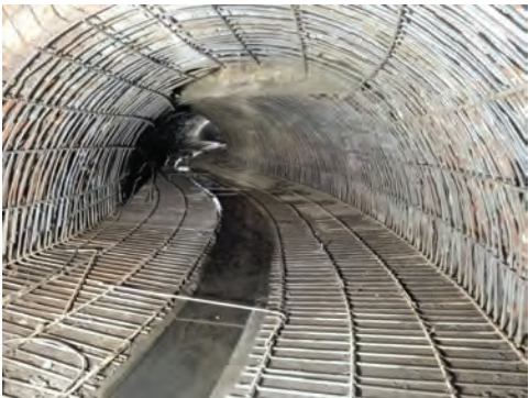
Fig. 8: Fixing reinforcement FE 500D
