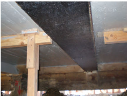
Fig. 9: Girder after application of CFRP and slab after application of epoxy coating (note areas of shoring that required later touchup)
