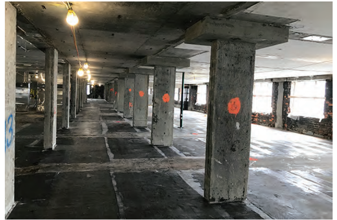
Fig. 8: The hallway and room slabs after the CFRP installation, focusing on the 50 in (1270 mm) wide application
