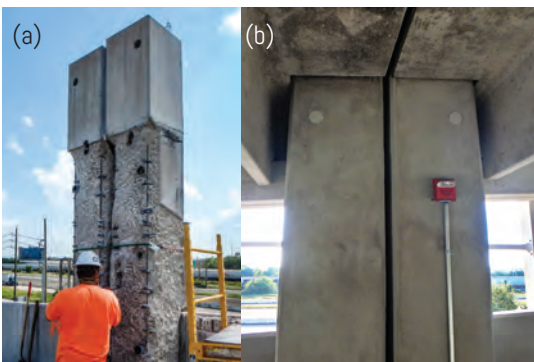
Fig. 8: Column repair (a and b)
