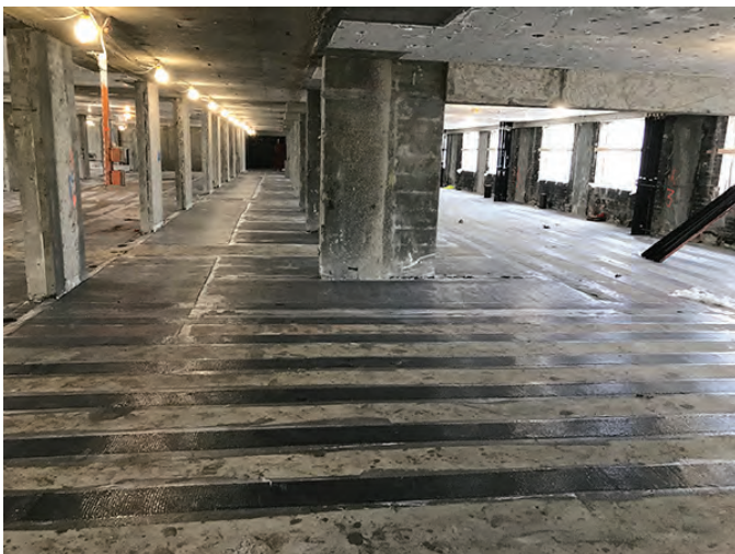
Fig. 7: The hallway and room slabs after the CFRP installation, focusing on the 8 in (200 mm) wide application
