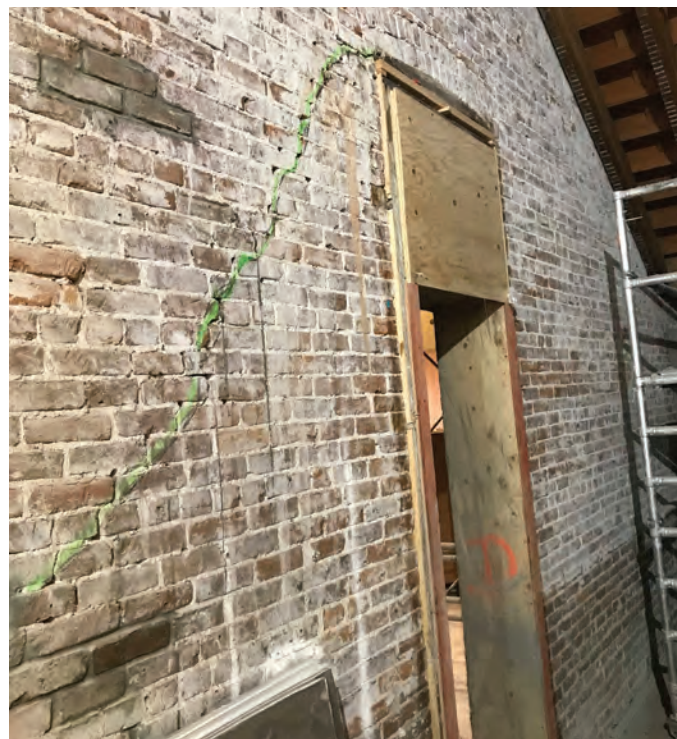
Fig. 3: The unreinforced masonry walls crumbled while the glass from the vaulted glass dome on the second floor was undamaged
