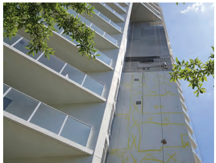
Fig. 3: Stucco marked up for removal after sounding
