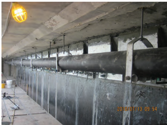
Fig. 13: External post-tensioning system
