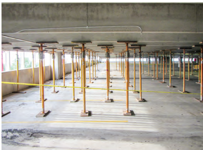
Fig. 4: Shoring installed in affected area
