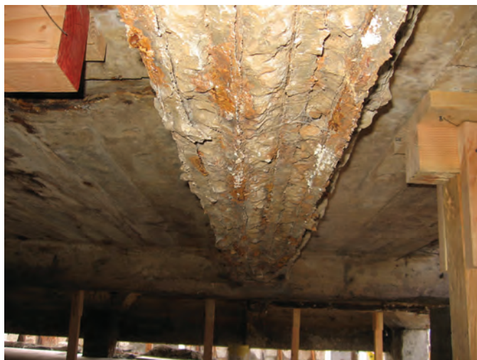
Fig. 2: Extensive spalling of the beams, girders, and slabs caused by severe corrosion of the reinforcing steel
