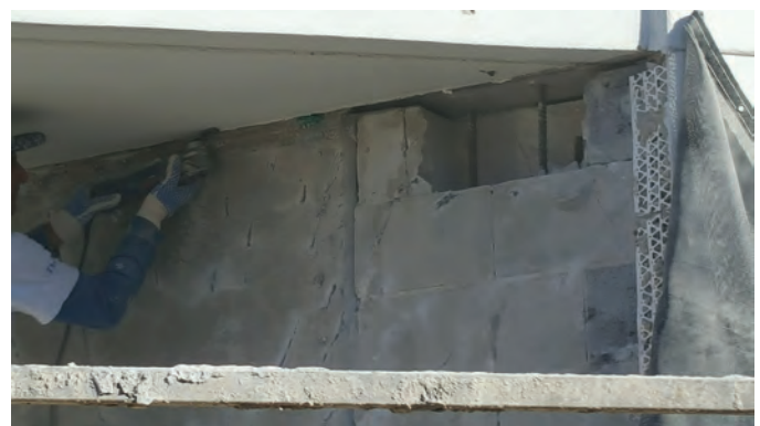
Fig. 4: CMU reinforced cells missing grout
