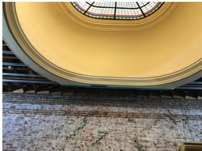
Fig. 2: The unreinforced masonry walls crumbled while the glass from the vaulted glass dome on the second floor was undamaged
