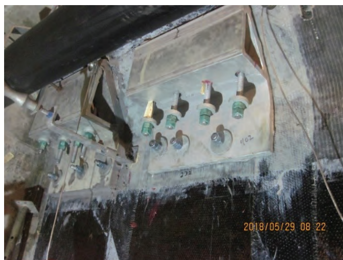
Fig. 11: Steel CFRP anchor plates
