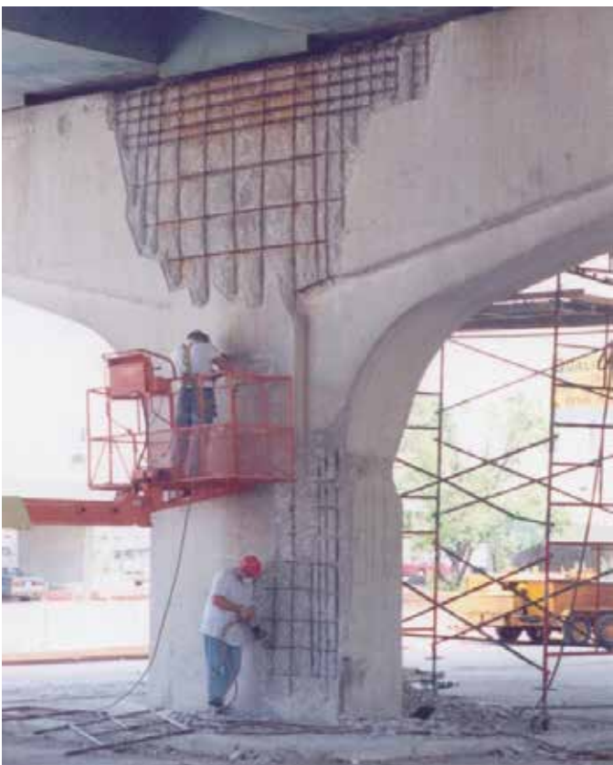
Fig. 4: Removal of delaminated and spalled concrete
