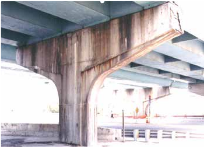
Fig. 3: Pre-treatment pier condition
