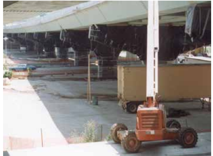
Fig. 7: ECE treatment in progress
