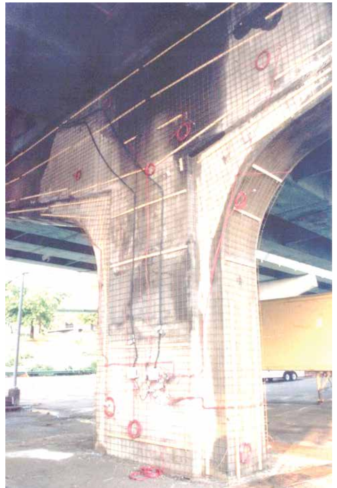
Fig. 5: Application of temporary external anode
