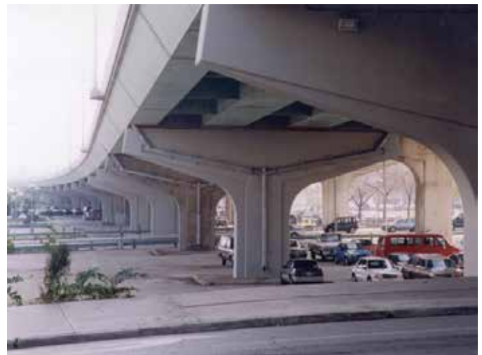
Fig. 8: Completed ECE process and coated piers
