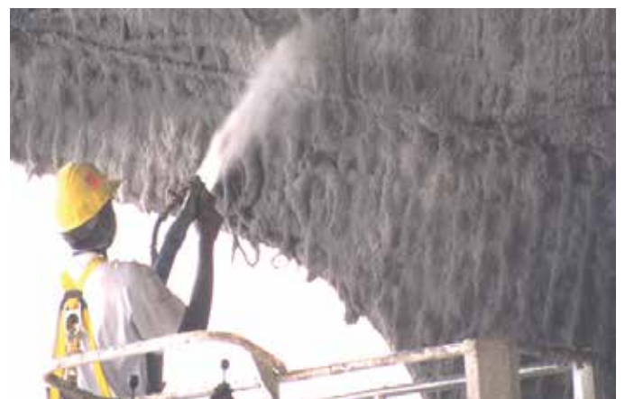
Fig. 6: Application of cellulose electrolyte
