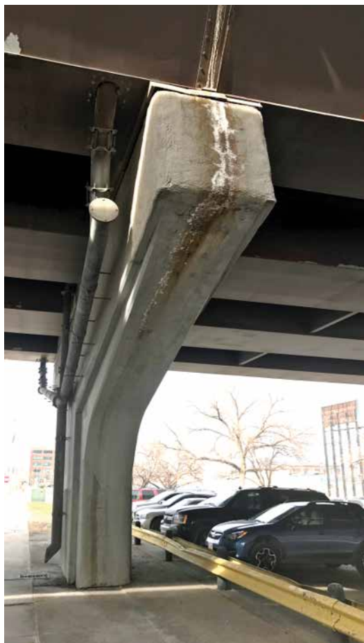
Fig. 11: Potential deterioration at leaking joint
