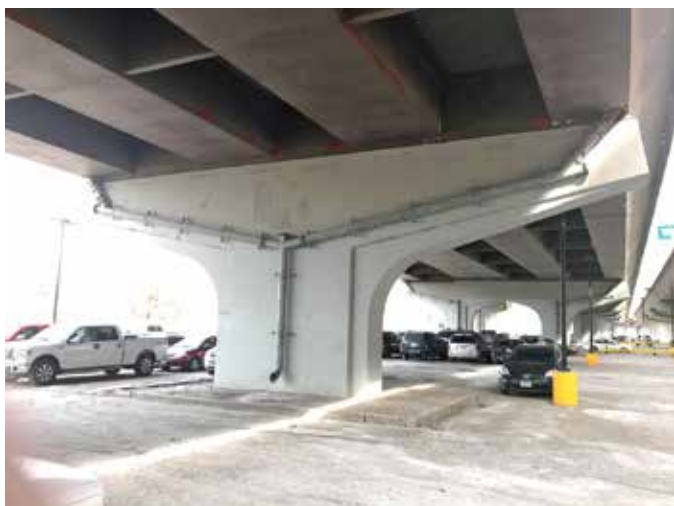
Fig. 10: Typical pier at 20 years after ECE treatment
