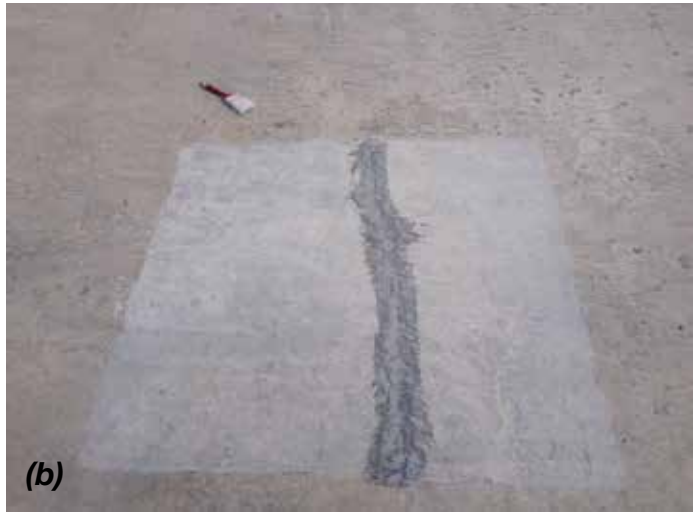
Linear transverse cracks on new bridge deck due to plastic shrinkage—surface grinding to open the face of the crack (a) and sealing with epoxy (b)
