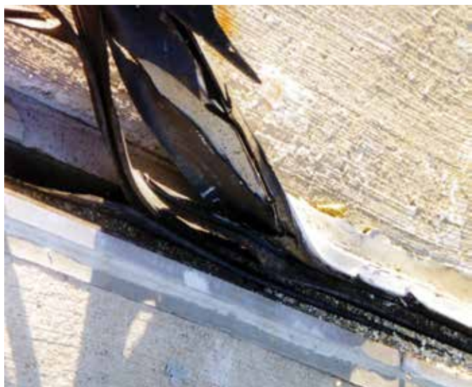
Fig. 7: Expansion joint seal damaged by snowplow
