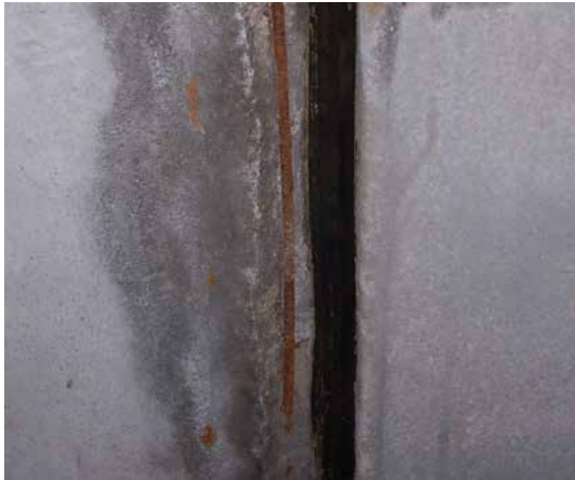
Fig. 1: Expansion joint “failure” showing water and rust staining at the slab underside
