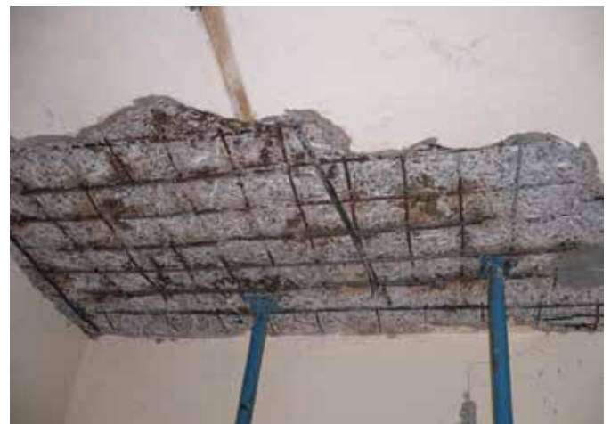
Soffits severely corroded due to roof leakages into a residential building
