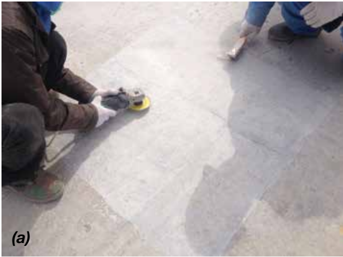
Linear transverse cracks on new bridge deck due to plastic shrinkage—surface grinding to open the face of the crack (a) and sealing with epoxy (b)
