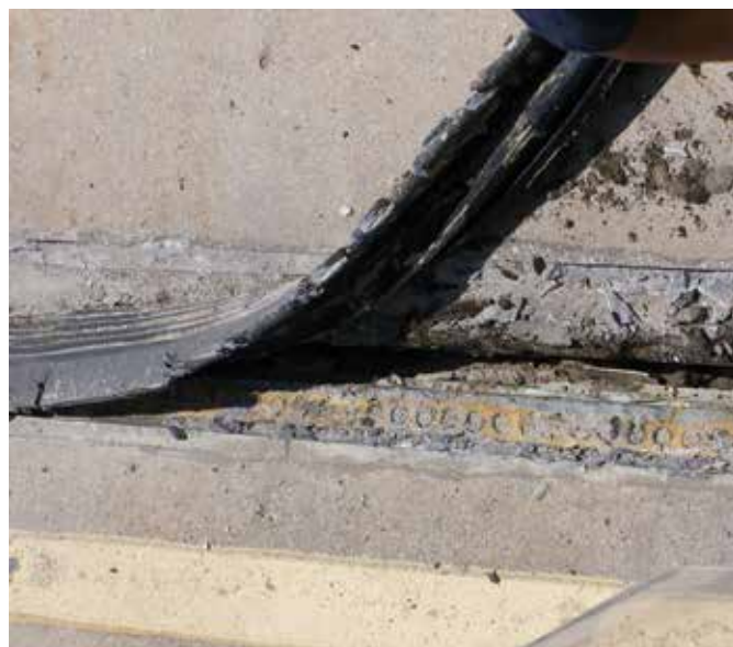
Fig. 2: Restoration projects present unique challenges – difficult to assess extent of repairs required until existing material is removed
