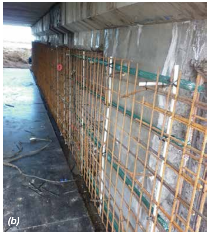
Cathodic protection to bridge piers affected by cracks, corrosion and spalled concrete, using embedded galvanic anode units (a) and distributed galvanic anode system (b)
