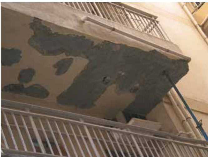
Repair of balcony concrete corrosion and spalling due to multiple factors
