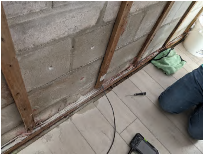
Fig. 5: Investigative exploratory opening inside condo unit revealing water intrusion
