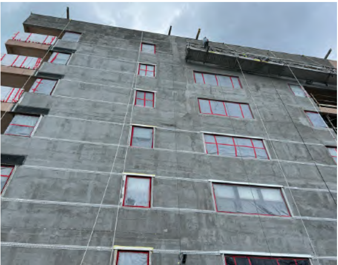
Fig. 8: Stucco installation in progress
