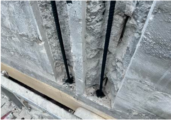
Fig. 6: Structural strengthening installation at the exterior of the building
