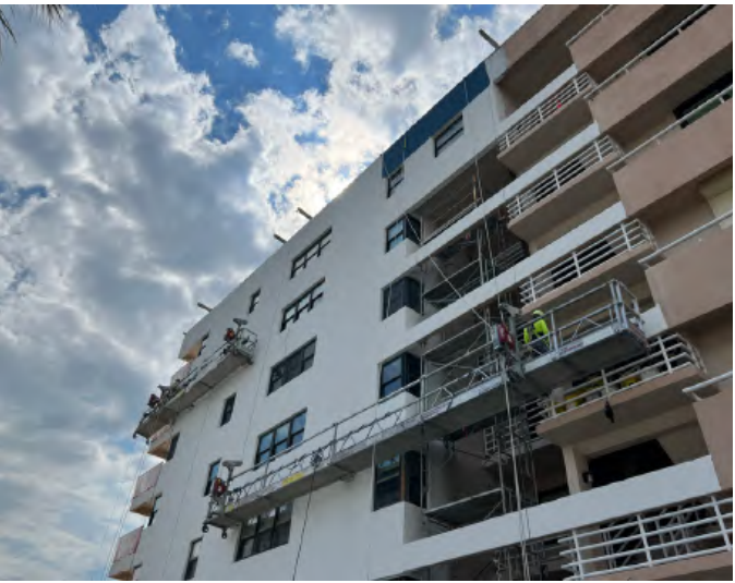
Fig. 9: Elastomeric coating installation in progress
