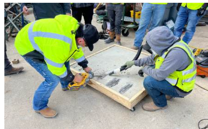
Fig. 4: Removing concrete from around reinforcing bars
