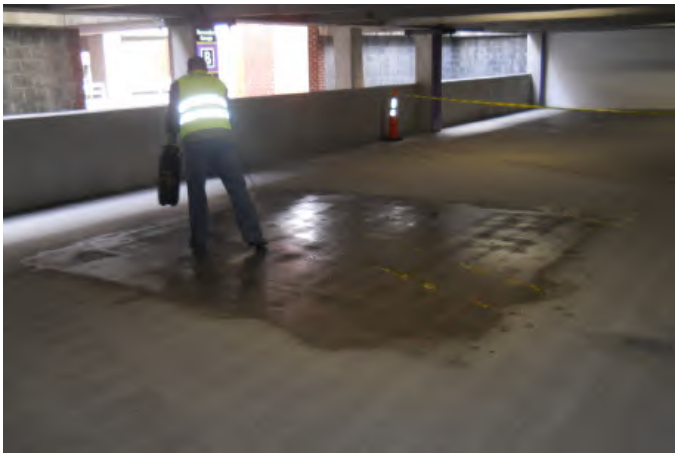
Fig. 8: Application of surface-applied corrosion inhibitor to parking garage surface at test area showing sectioned installation for ensuring adequate coverage rates
