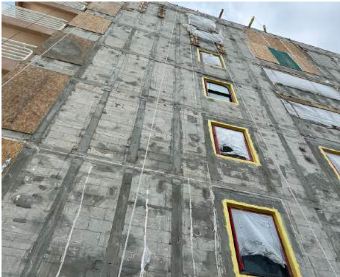
Fig. 7: Completed structural strengthening at the exterior of the building
