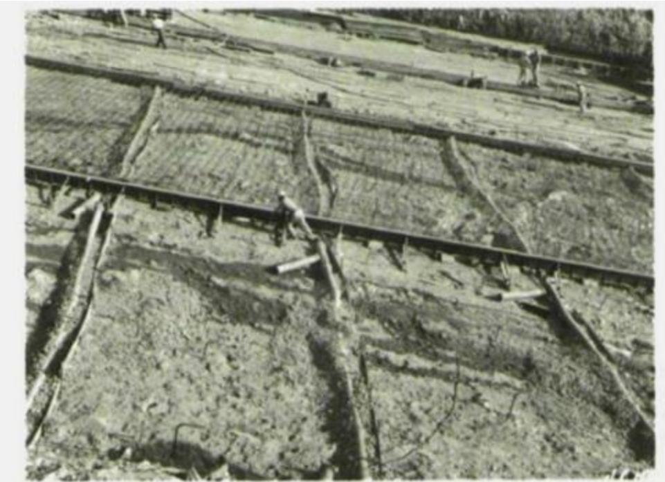
Photo 39. Chute foundation in vicinity of Sta. 33+60. Tile and gravel underdrains in lanes 2 and 3, rebar in lane 3. View southeast. Neg. No. 4644 11-2-66
