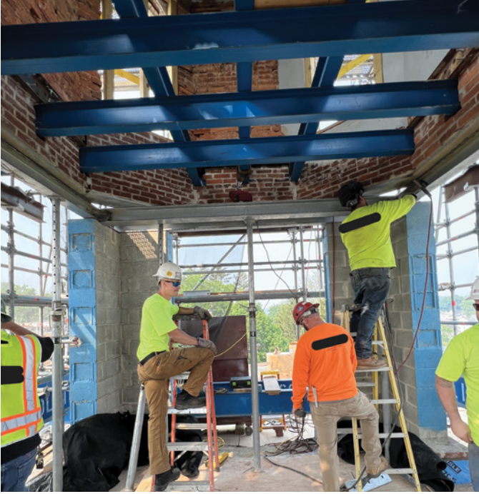
Image 5: Tower base reconstruction with structural steel installed
