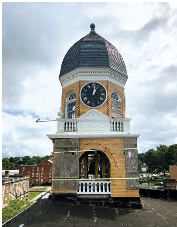
Image 2: Deficiencies in the tower base
