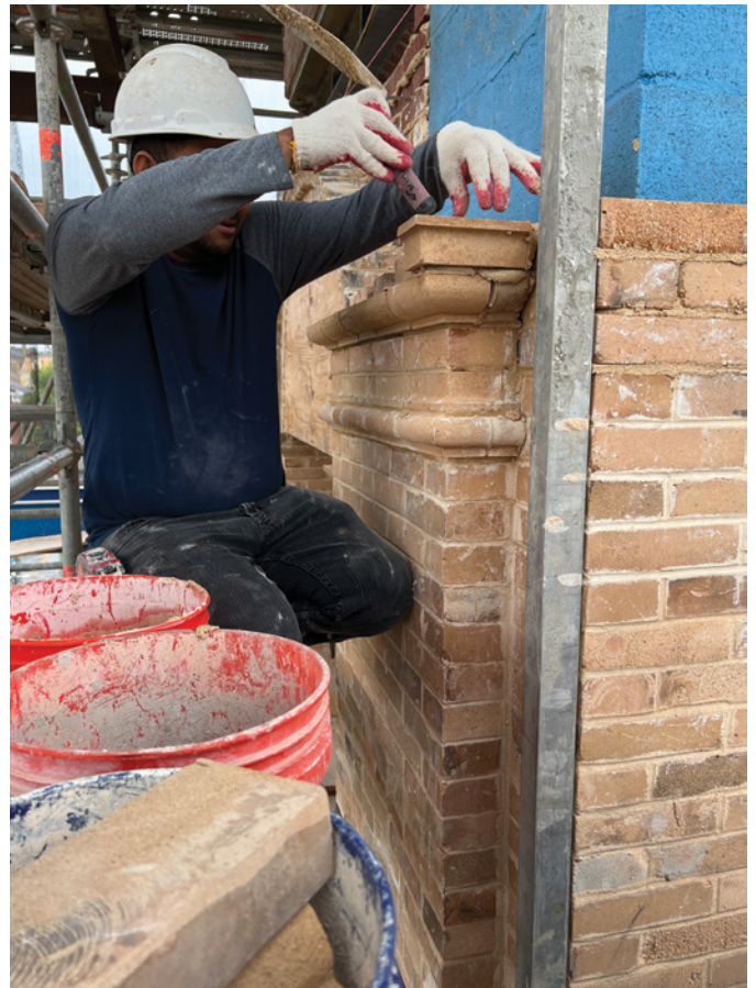
Image 8: Salvaged brick veneer installation
