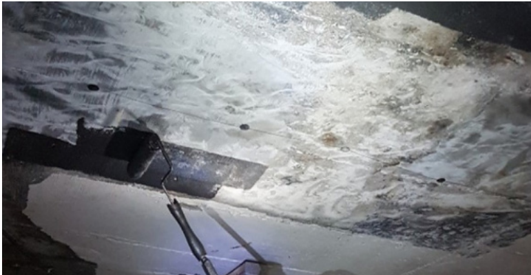
Applying the highly conductive coating (carbon rich coating that looks like black paint) to the soffit fully
