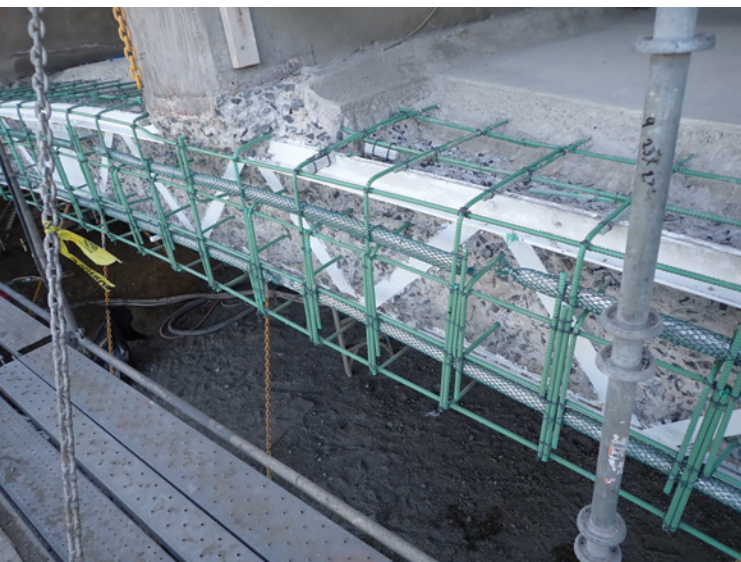
Image 7: Arch corner repair extending across full height of barrel arch, showing continuous and discrete CP anodes, supplemental rebar/anchorages, and coated Melan steel
