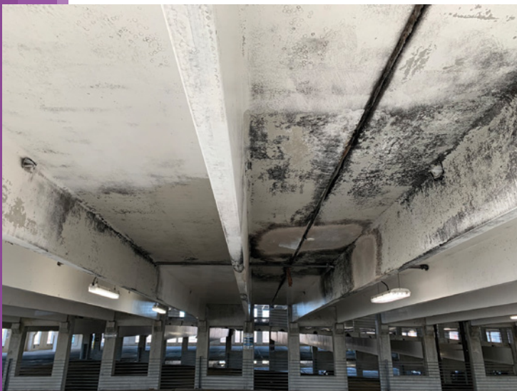
Image 2: Fire damage to the underside of the level four precast double tees
