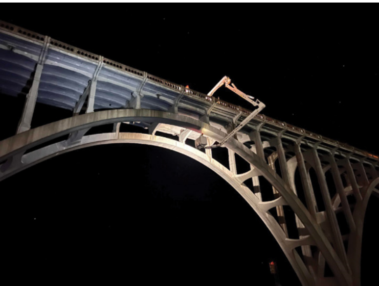
Metalizing from Snooper Truck
