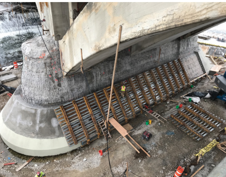
Image 9: Pier base jacket repair in progress, showing cofferdam, concrete removals, and supplemental rebar/anchorages at top, and formwork and new concrete jacket at bottom of pier
