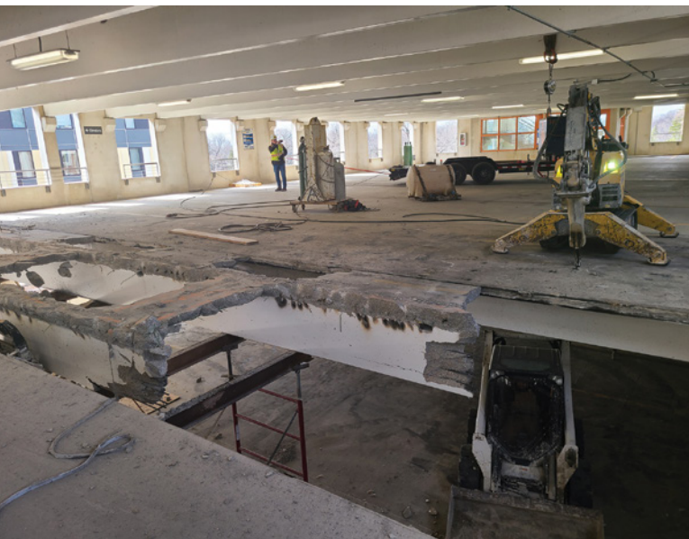
Image 6: Remote controlled demolition
