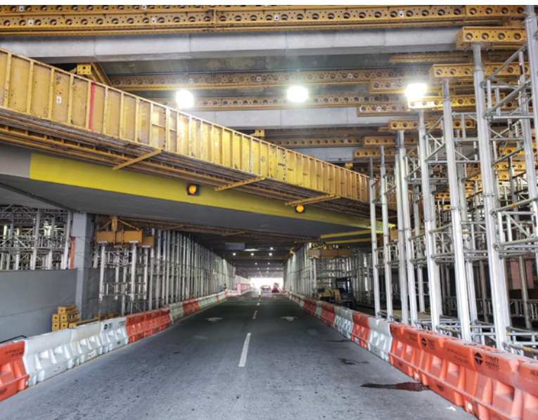
Shoring layout on Terminal Parkway to maintain partial use of the roadway during construction
