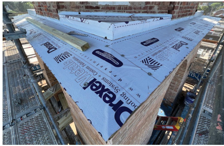
Image 7: Waterproofing and flashing materials installed
