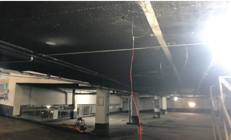
Installing bare platinized niobium wires embedded within the conductive coating
