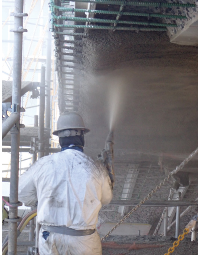
Image 8: Application of wet-mix shotcrete to arch underside
