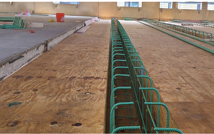
Image 9: Partial rebar detail with formed repair
