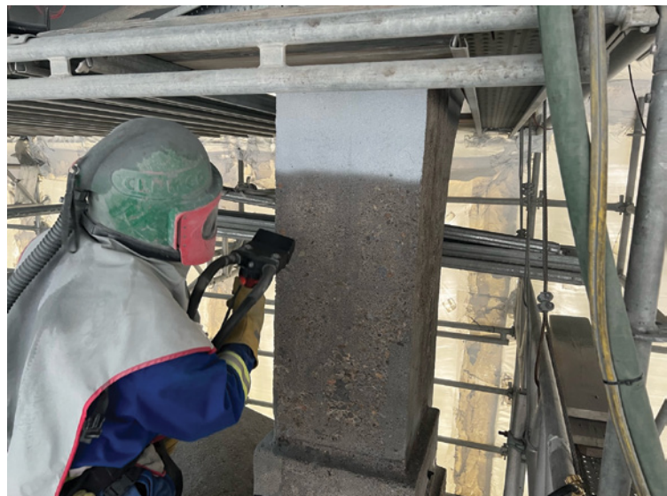
Metalizing on a properly prepared concrete surface
