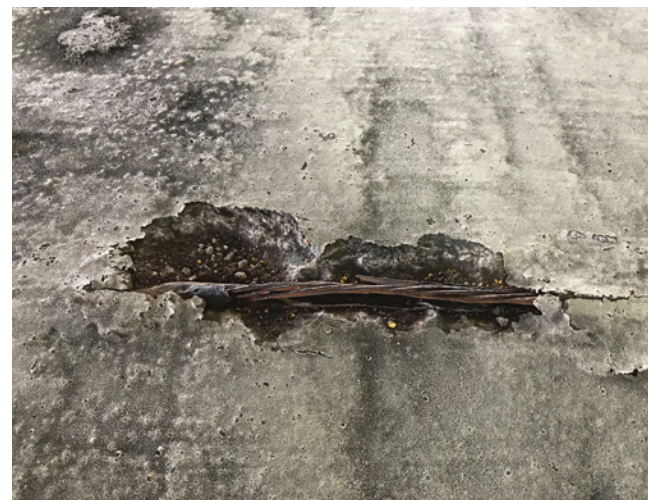
Failed PT tendon with multiple broken wires protruding from the top of the slab
