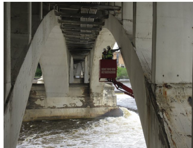
Image 2: Hands-on inspection from under-bridge inspection unit (snooper), illustrating deterioration of arch ribs and pier bases
