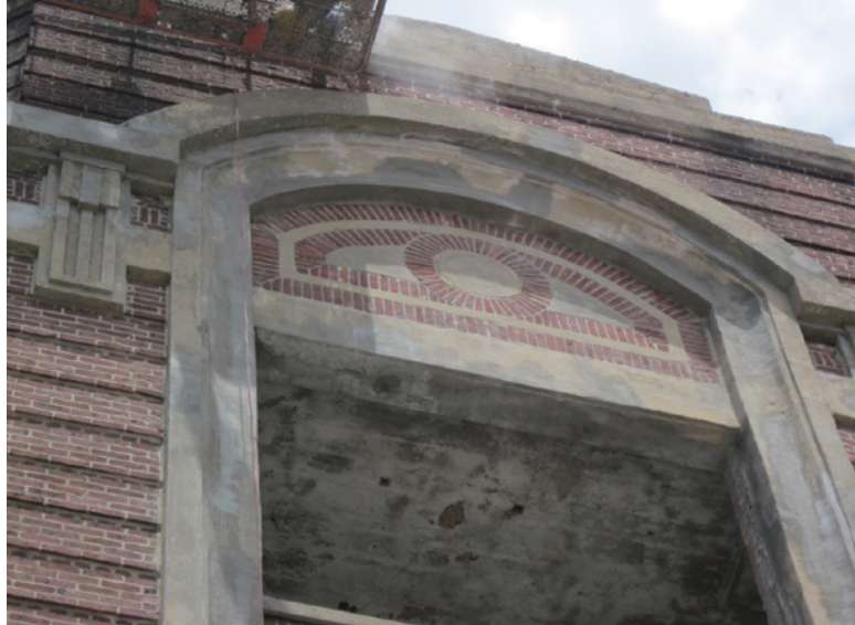
Image 8: Hand-applied mortar in 2014
