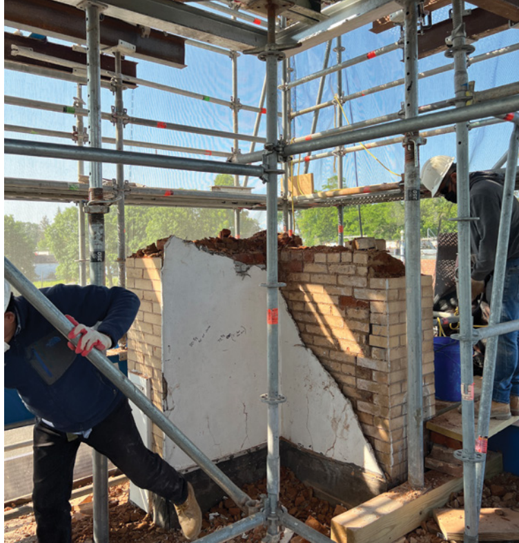
Image 4: Demolition of the tower base with shoring
