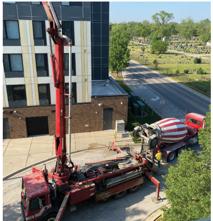
Image 5: Pump truck positioned to pump through opening
