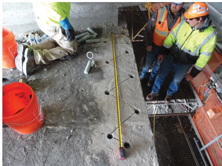
Image 11: Discrete, two-stage anodes installed in cored holes along sound arch corners between corner repairs
