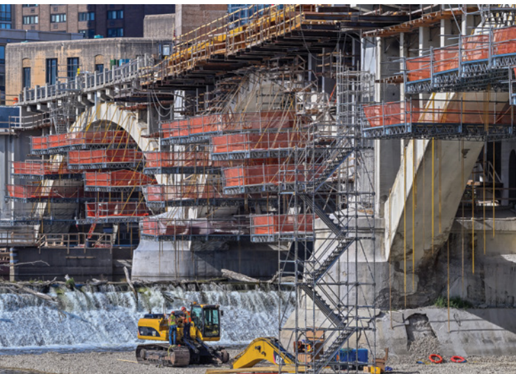
Image 6: View of multiple means of access, including suspended scaffolding and dewatered cofferdam. (Photo credit: Joe Szurszewski Photography)
