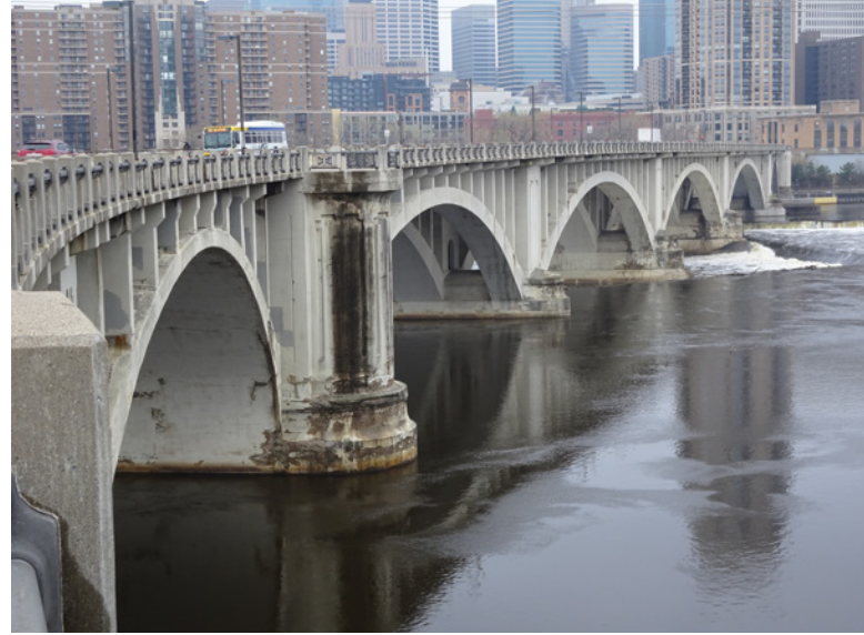
Image 13: "Before" photograph along upstream side of bridge, showing concrete deterioration in pier bases and arches
