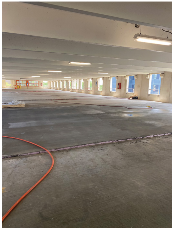
Image 11: Precambered form edge after concrete placement
