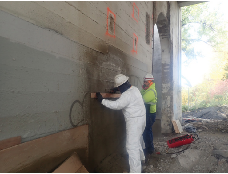
Image 12: Hand-finishing board form lines in shotcrete repairs on pier face to match existing surface texture
