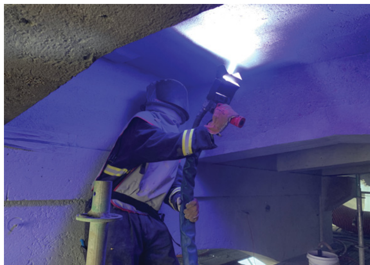
Installing thermally sprayed ICCP system
