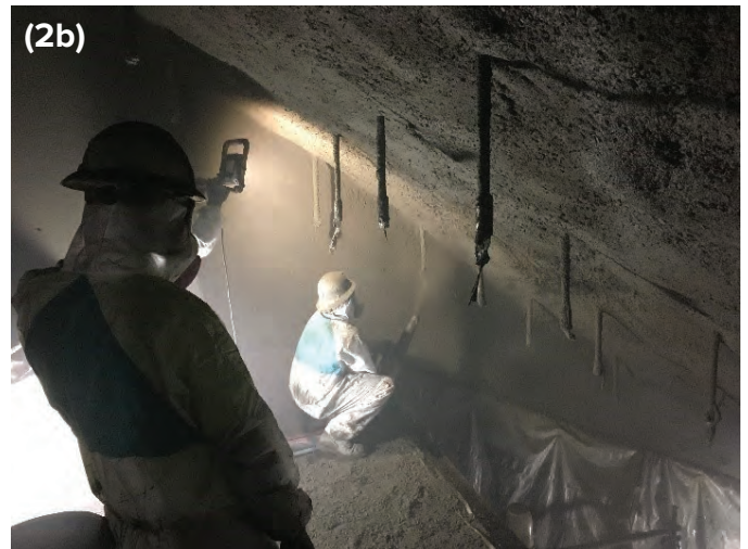
Fig. 2a) Slick line entering the draft tube from the power house; 2b) Nozzleman shooting overhead on a scaffold platform in a crouching position maintaining suitable shooting angle and distance to the receiving surface and building out shotcrete to the shooting wires.
