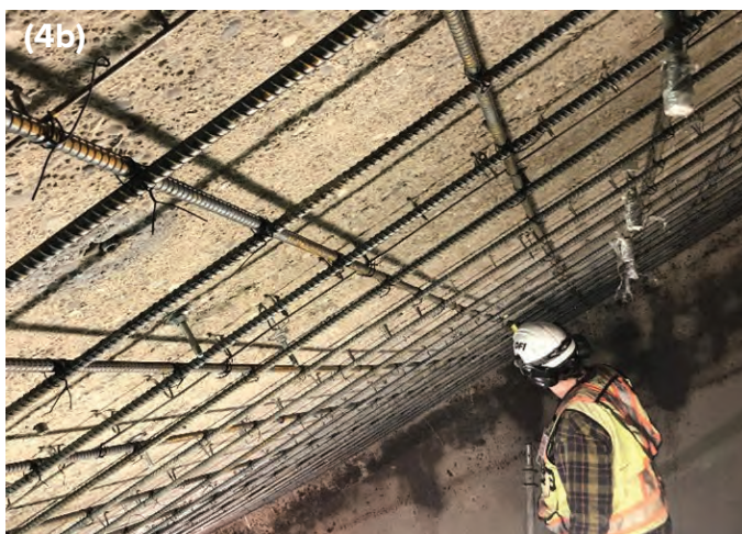
Fig. 4a) Permanent steel form; 4b) Ceiling slope, concrete substrate, 254 mm (1 in) anchors and 15M (No. 5) rebar installed for shotcrete application
