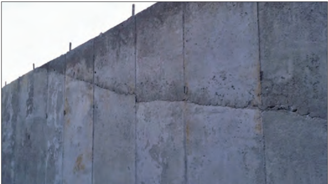
Fig. 7: Form-and-pour wall with cold joint
