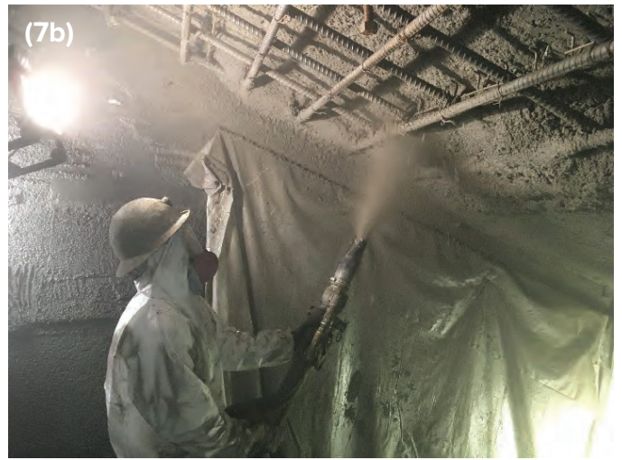
Fig. 7a): Nozzleman shooting in an upright position adjacent to steel form to achieve 90° shooting angle to receiving surface 7b): Nozzleman shooting to the 30M rebar at high impacting velocity
