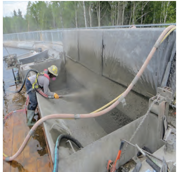
Fig. 1: Remote dam repair using dry-mix shotcrete and a cofferdam (Côté, Ferland, and Robertson 2014)
