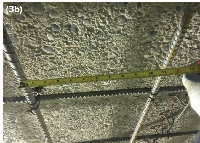
Fig. 3a): ICRI CSP 7 surface roughness profile; 3b): Substrate concrete surface and No. 5 bars measured to be approximately 12" O.C. E.W.
