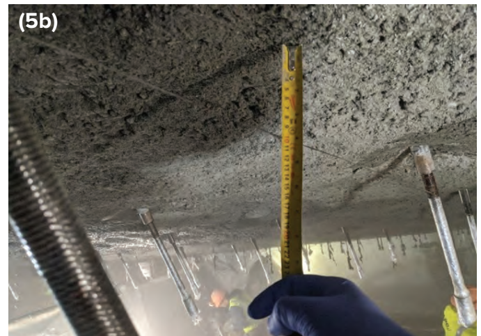
Fig. 5a): Formwork, 12.7 mm (0.5") anchors, 15M rebar and nozzleman shooting to prepared concrete substrate; 5b) 254 mm (1 in) diameter anchor and a shooting wire to control thickness
