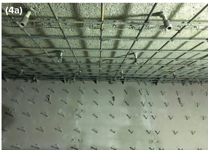
Fig. 4a) Permanent steel form; 4b) Ceiling slope, concrete substrate, 254 mm (1 in) anchors and 15M (No. 5) rebar installed for shotcrete application
