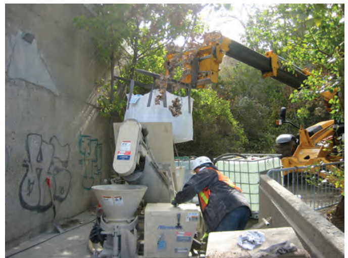
Fig. 4: Dry-mix equipment with supersack prebagged concrete materials
