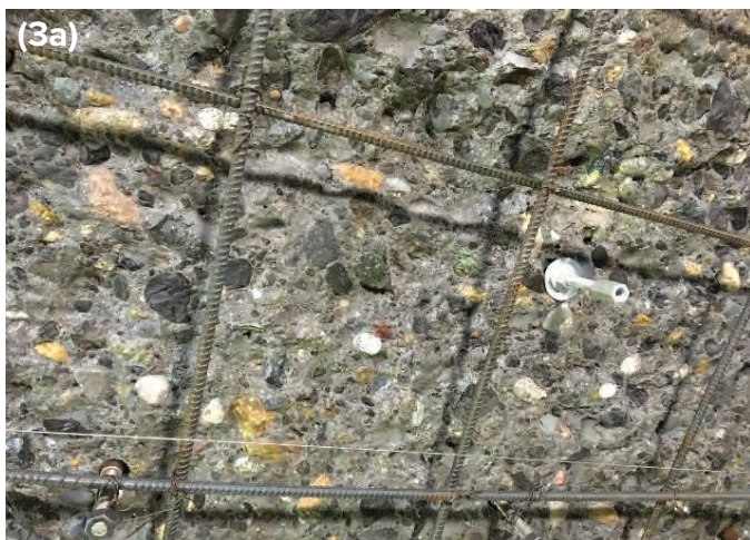
Fig. 3a): ICRI CSP 7 surface roughness profile; 3b): Substrate concrete surface and No. 5 bars measured to be approximately 12" O.C. E.W.
