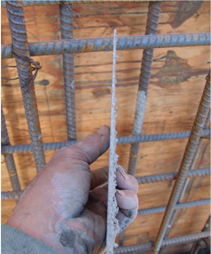
Fig. 8: Demonstration of thin paste-rich shotcrete layer at substrate
