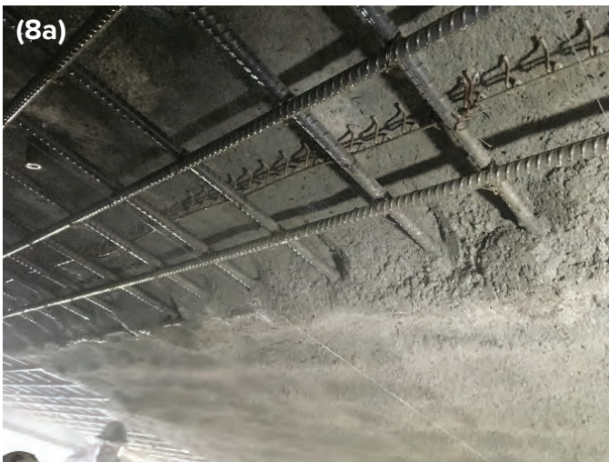
Fig. 8a) Inspecting quality of shotcrete around 30M rebar. 8b) using blow pipe to remove overspray from rebar
