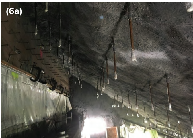
Fig. 6a): Profile of ceiling following shotcrete application to 15M rebar, anchor extensions, and steel form; 6b) high pressure water blasting shotcrete surface to clean the surface prior to shotcrete application of succeeding layers.
