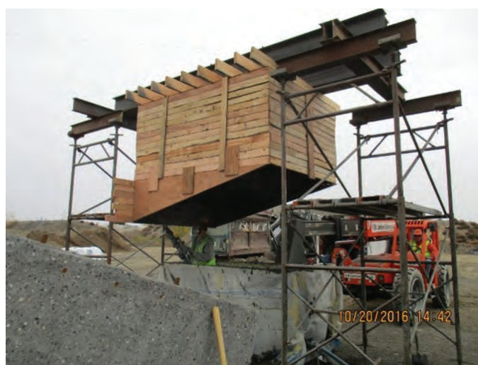
Fig. 1: Nozzleman shooting the final lift of the full-scale mock-up (Ref. 2)
