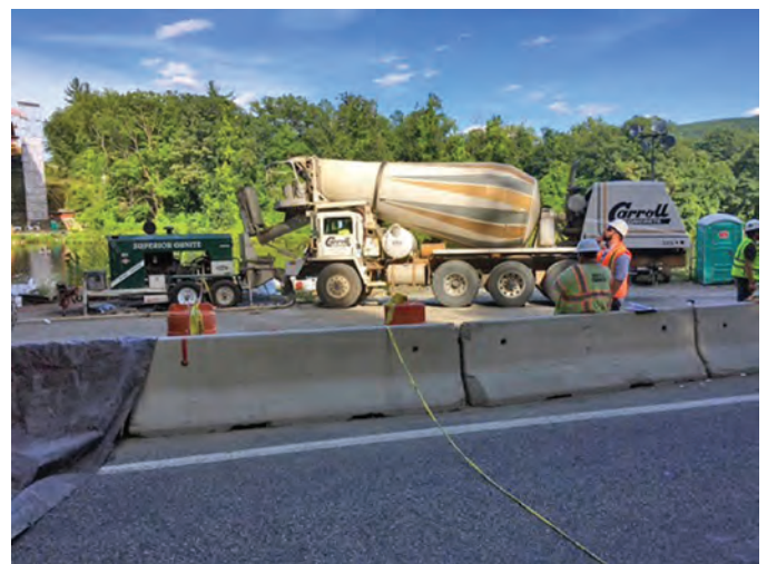
Fig. 6: Wet-mix equipment – small line concrete pump with ready-mix truck
