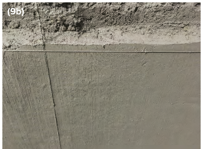
Fig. 9a): Dry-mix shotcrete to the finish line, cut and screed, and wood float finishing. 9b): A close up of the final broom finish appearance.
