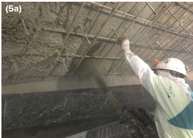
Fig. 5a): Formwork, 12.7 mm (0.5") anchors, 15M rebar and nozzleman shooting to prepared concrete substrate; 5b) 254 mm (1 in) diameter anchor and a shooting wire to control thickness
