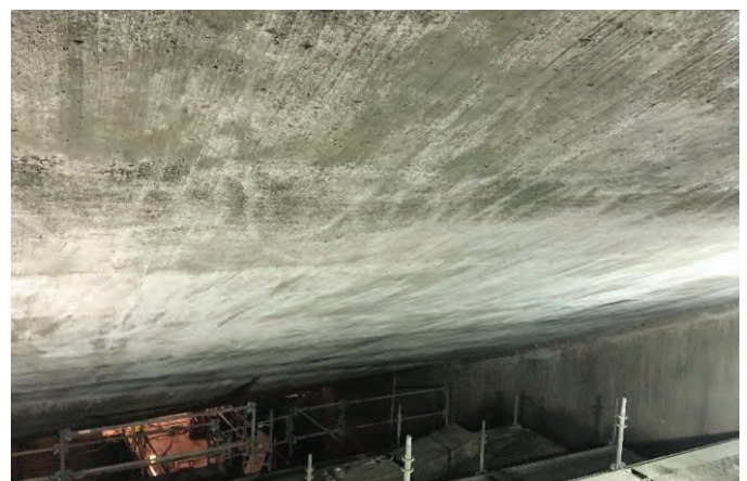
Fig. 11. Re-profiled draft tube
