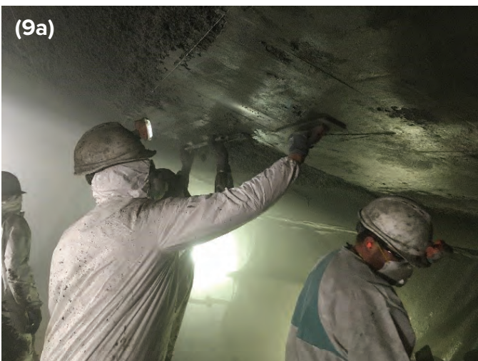
Fig. 9a): Dry-mix shotcrete to the finish line, cut and screed, and wood float finishing. 9b): A close up of the final broom finish appearance.
