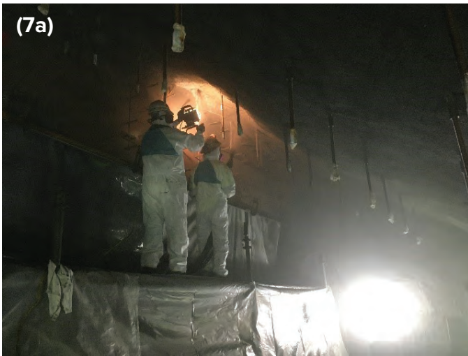
Fig. 7a): Nozzleman shooting in an upright position adjacent to steel form to achieve 90° shooting angle to receiving surface 7b): Nozzleman shooting to the 30M rebar at high impacting velocity
