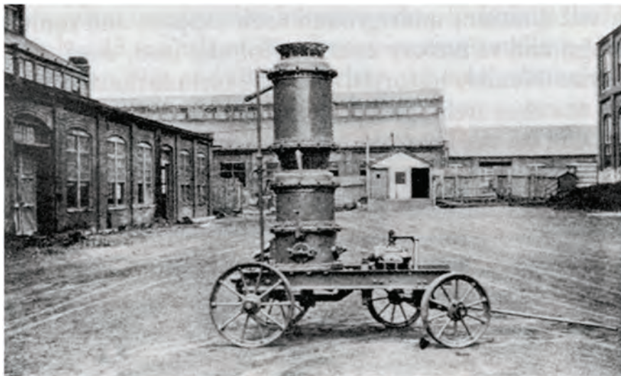
Fig. 1: Original shotcrete dual-chamber gun
