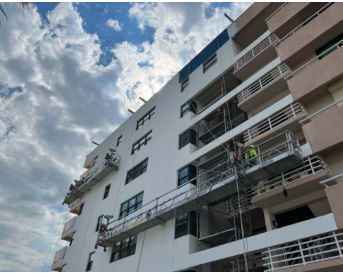
Fig. 9: Elastomeric coating installation in progress
