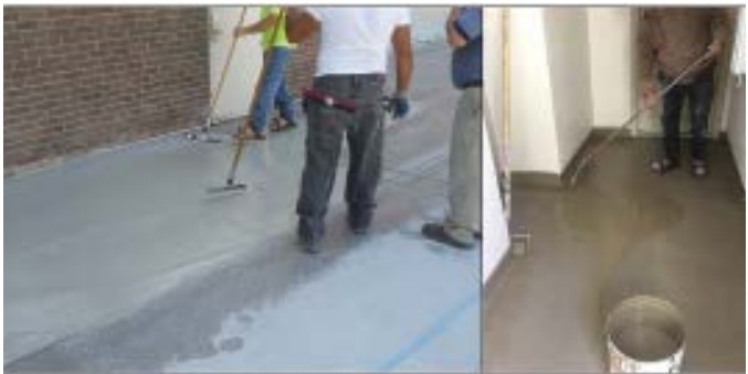
Fig. 7: (a) Cementitious and (b) polyurethane deck coatings
