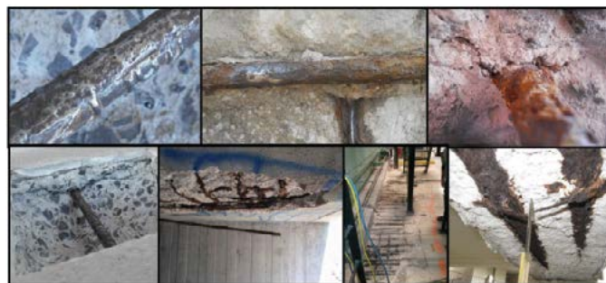
Fig. 3: Corrosion-related distress: (a) pitting from chloride-induced corrosion (after bar cleaning), (b) corrosion products compared to bare steel, (c) corrosion-induced cracking, (d) cross-section of delamination, (e) overhead delamination and spalling hazard, (f) horizontal spalling and tripping hazard, and (g) reinforcing steel disintegration
