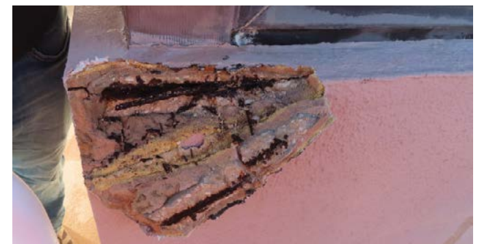
Fig. 4: Concrete spall due to corroded reinforcing steel at precast concrete window sill
