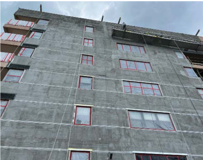
Fig. 8: Stucco installation in progress
