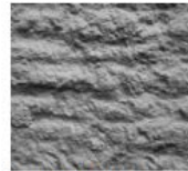
Fig. 6.9: CSP 9 (heavy scarification— rotomilled)
