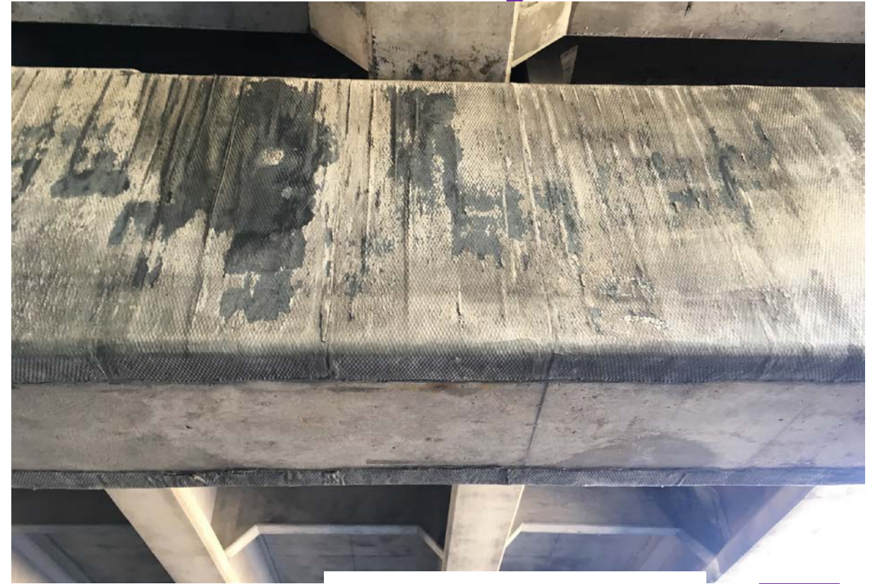
WB Pier 34, West Face, North End (2018)
