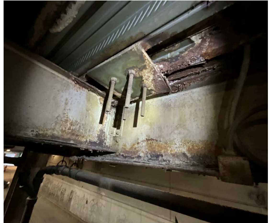
Flagpole attachment from underside
