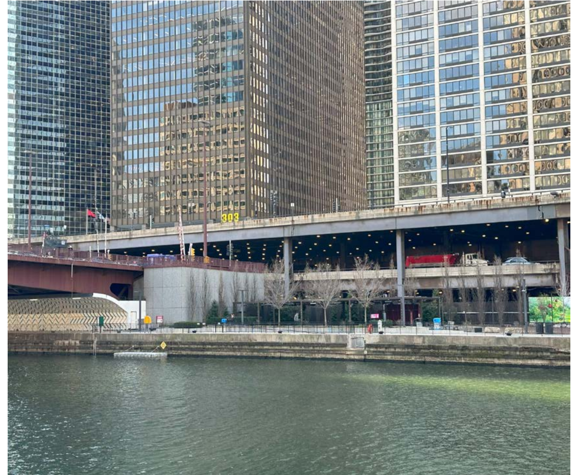
3-level section of Wacker Drive
