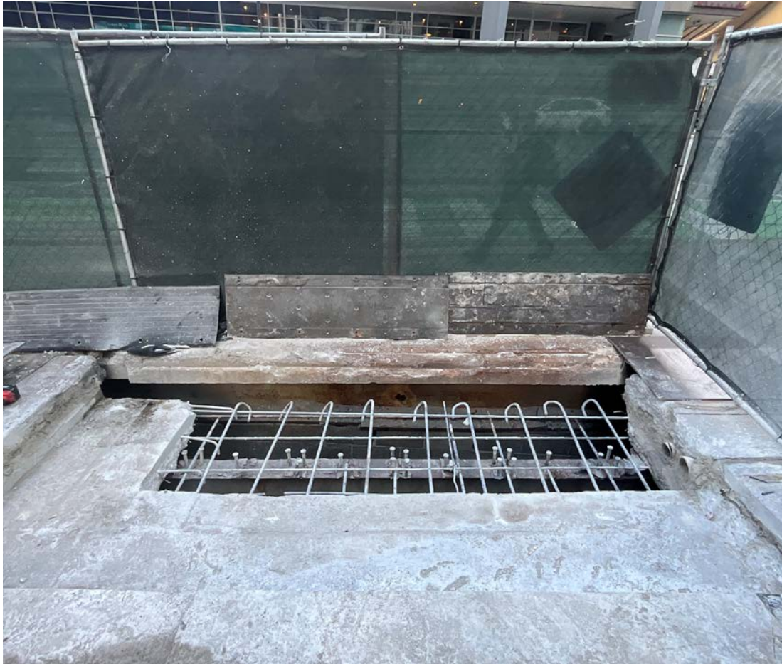
Unsound concrete removed
