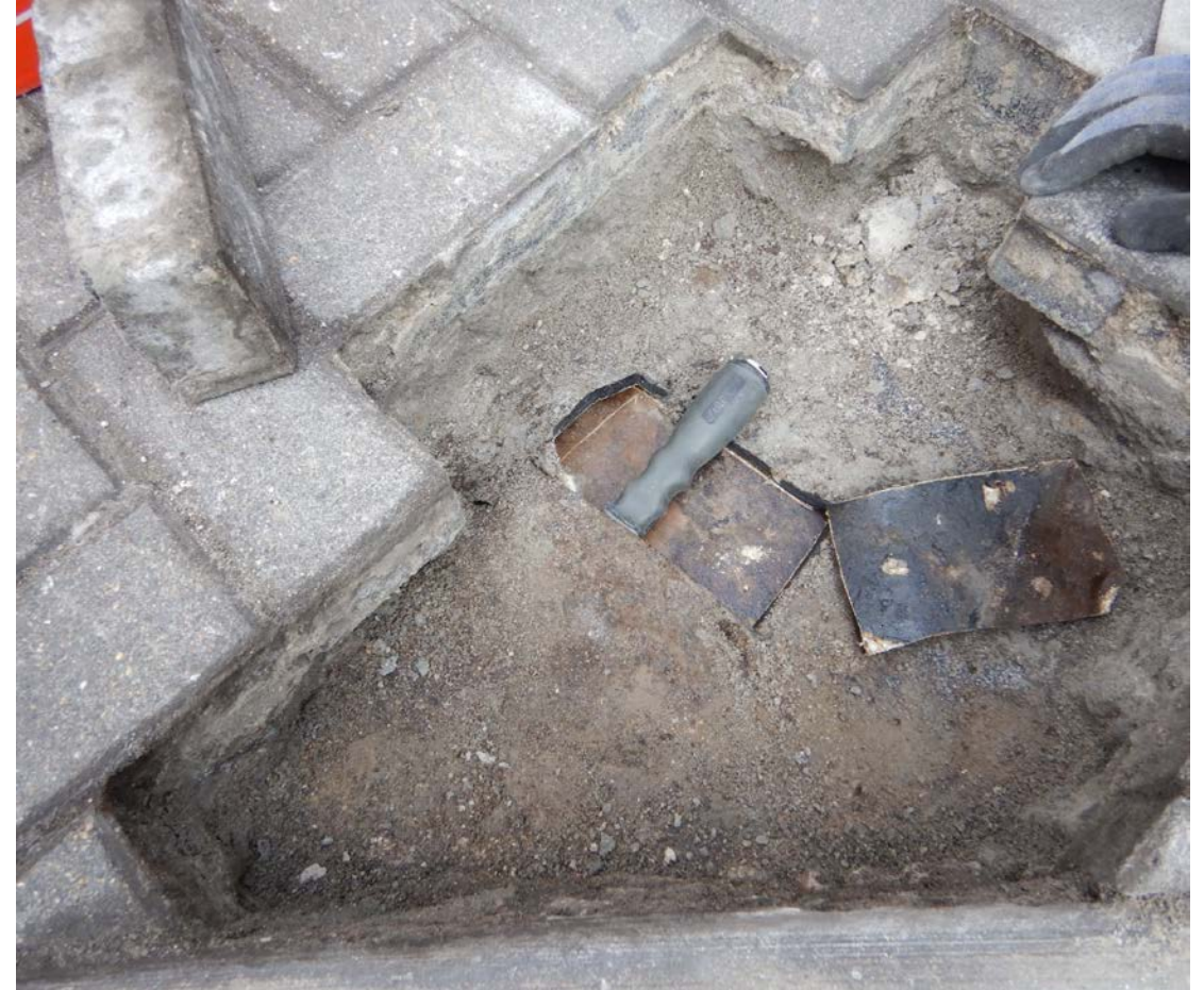
Debonded waterproofing
