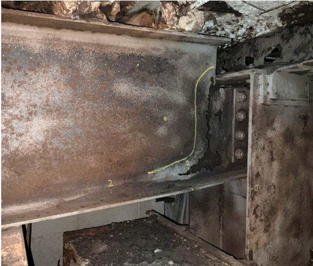
Markings on beam for field notes
