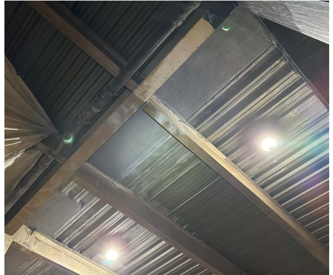
Completed shotcrete repair
