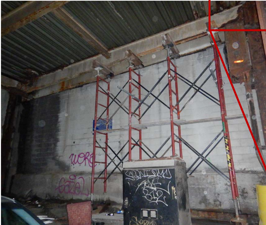
Shoring installed below beam
