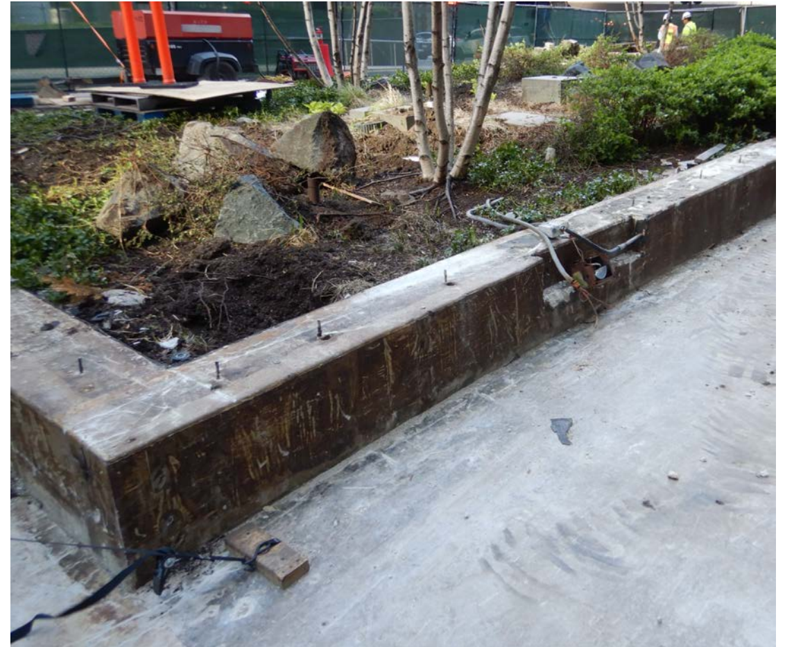
Planter with granite and waterproofing removed
