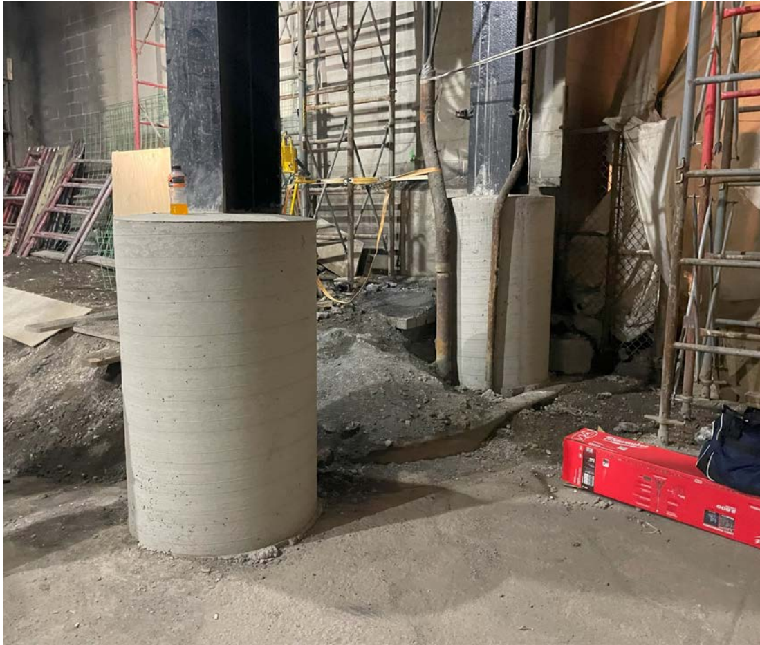
Completed encasement repair
