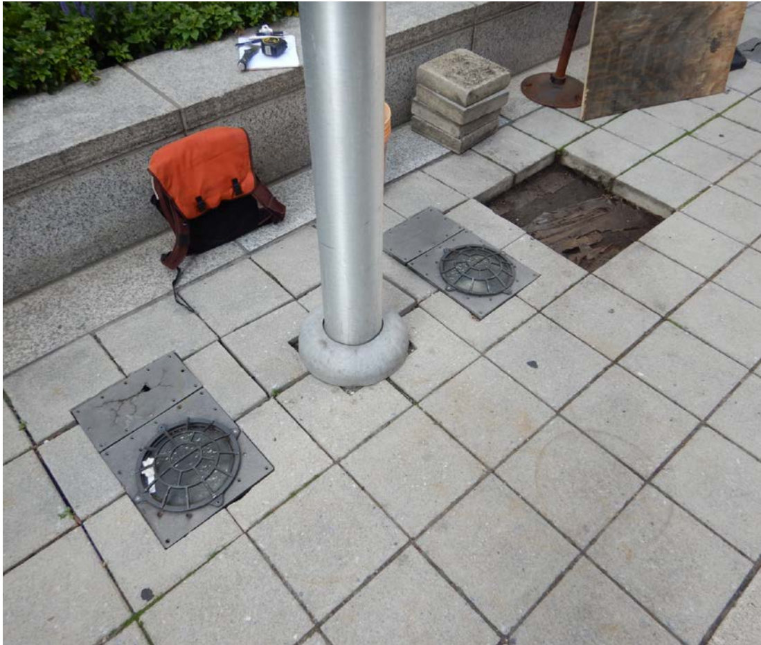
Flagpole and lights at topside
