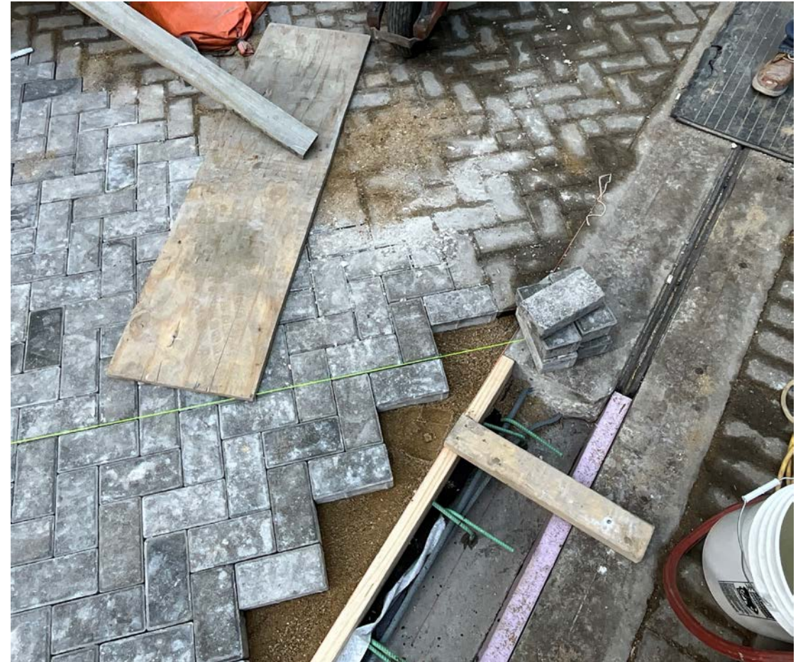
Tying in temporary pavers to existing
