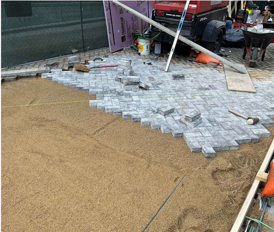
Temporary paver installation in progress
