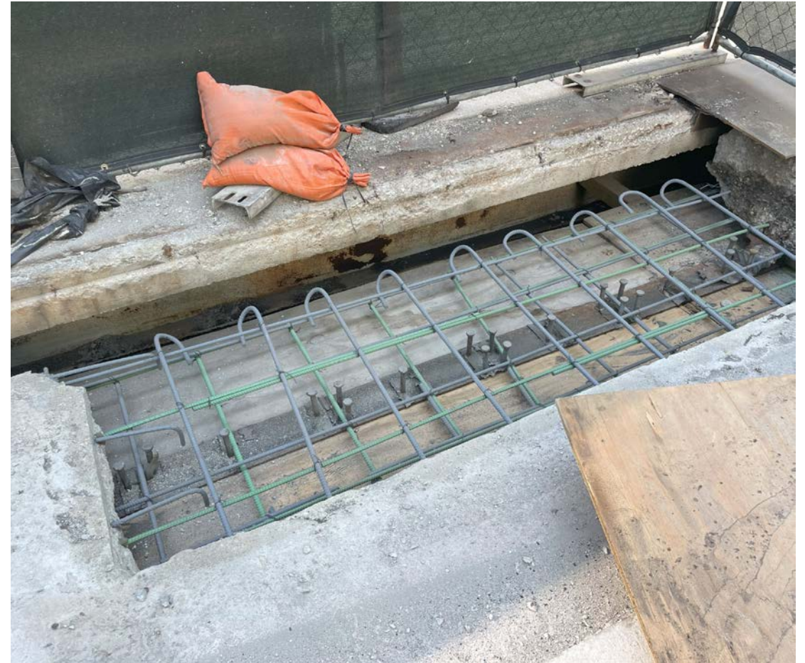
Cleaned steel, applied zinc-rich coating, and added supplemental reinforcing
