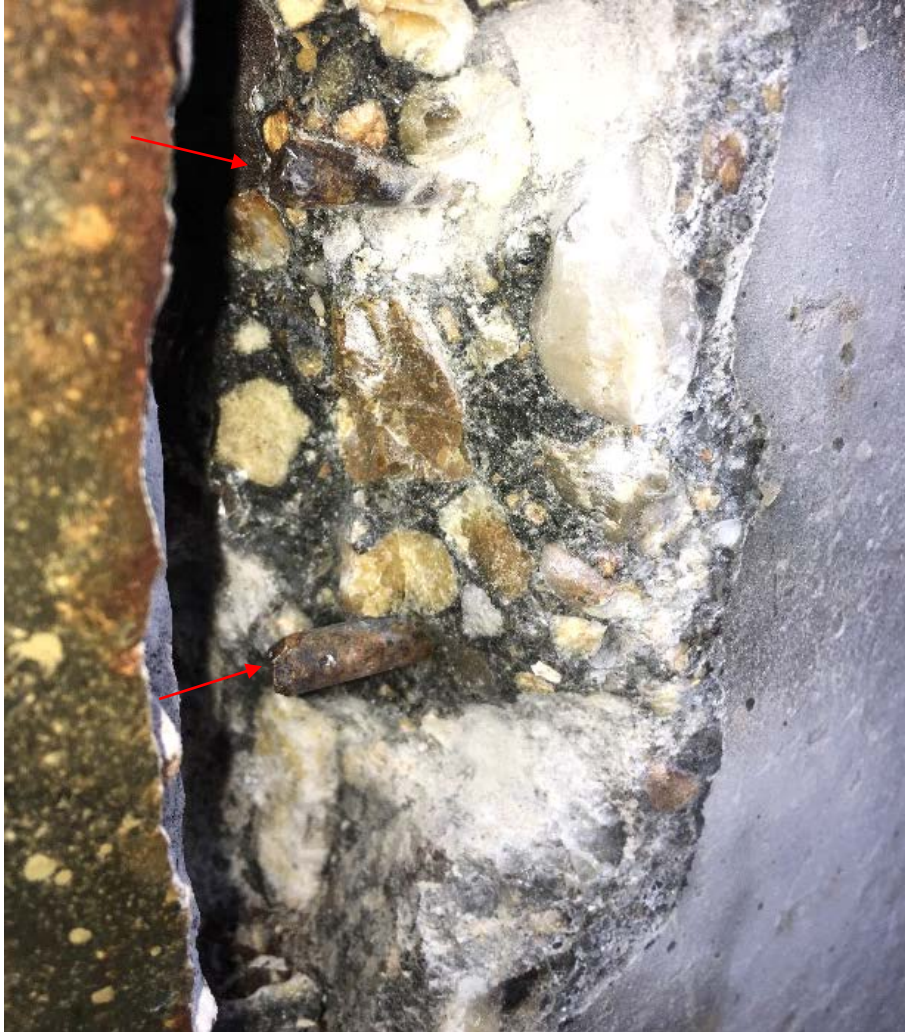
Opening Identified Completely Corroded Ties
