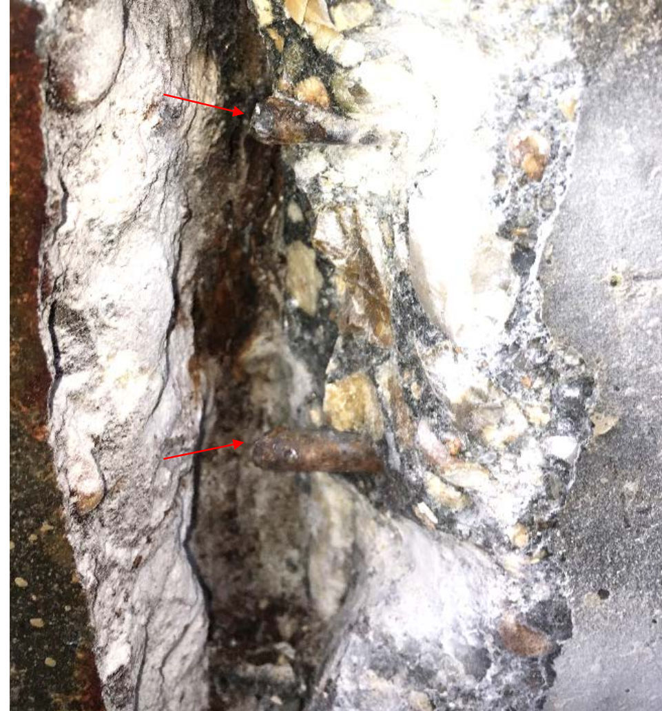
Opening Identified Completely Corroded Ties
