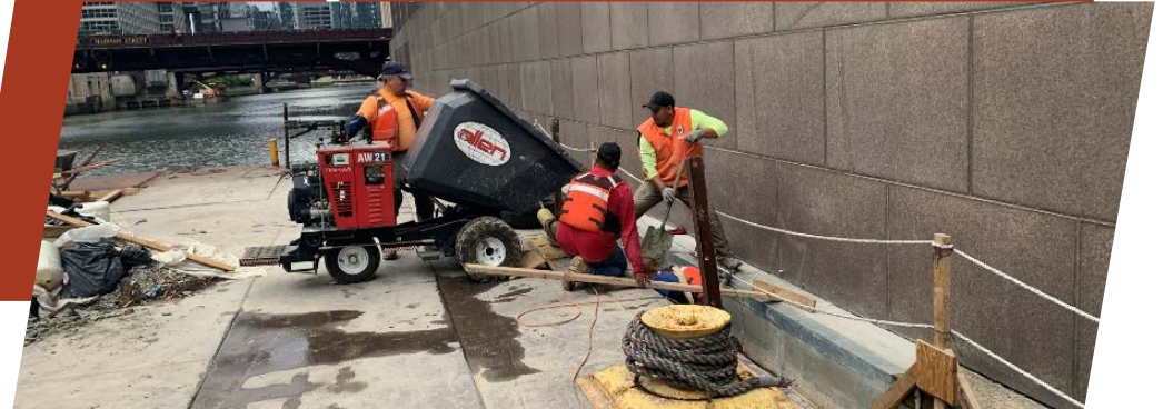
Partial Depth Below Water Concrete
