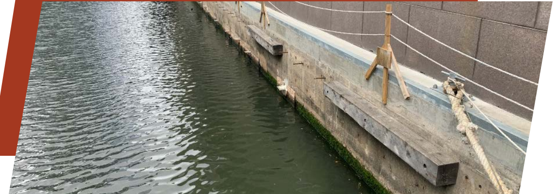
Crack Sealing & Installation of Sealer
