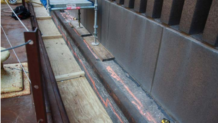
Overall and close-up views of delaminated concrete at the river wall concrete cap marked for removal
