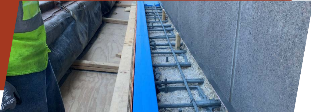
Partial-Depth Concrete Repairs
