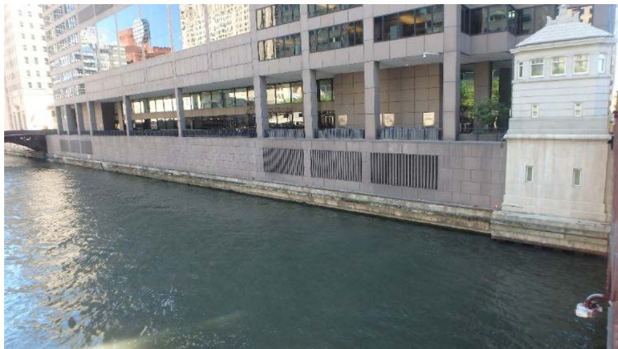
Overall view of river wall from Monroe Street bridge
