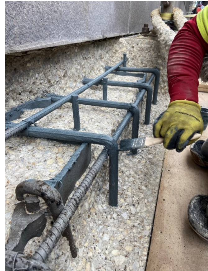
Painting of reinforcing bars with corrosion inhibiting paint
