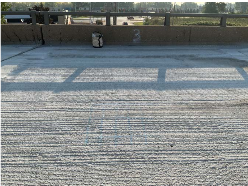
➤ Milling to final grade
