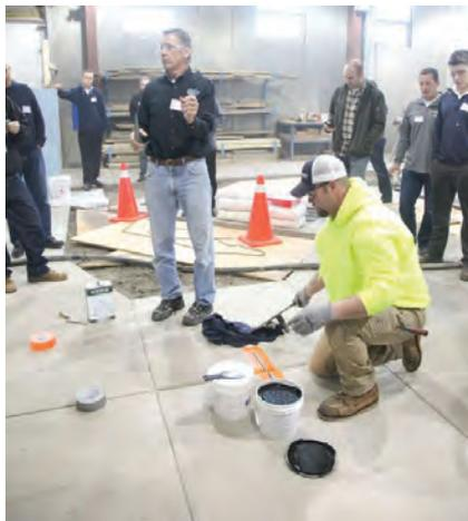
*Will Warlick from V2 Components demonstrated the use of custom glass fiber reinforced polymer “biscuits” and how they can be used in precast double tee beam repair*
