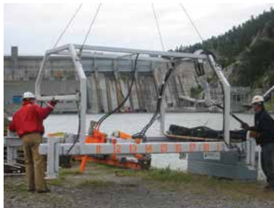
Fig. 5: Hydrodemolition cutting frame
