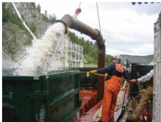
Fig. 3: Airlift system used to vacuum debris from the basin floor
