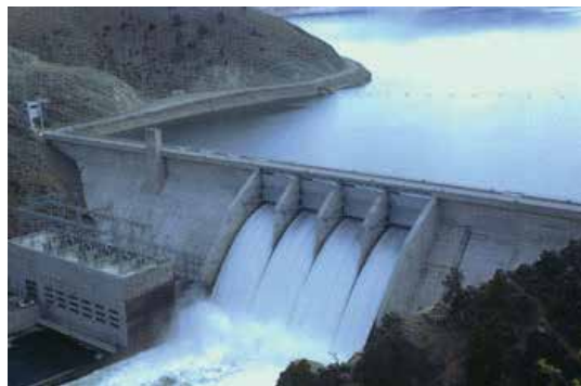
Fig. 1: Canyon Ferry Dam
