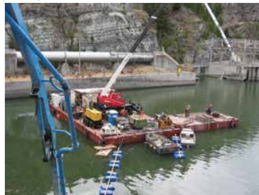
Fig. 7: Work barge in basin
