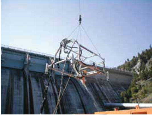
Fig. 8: Hydrodemolition cutting frame attached to crane
