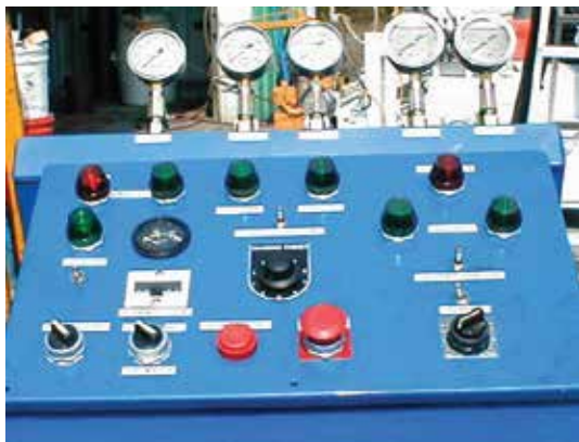
Fig. 6: Hydrodemolition control panel and hydraulic power pack
