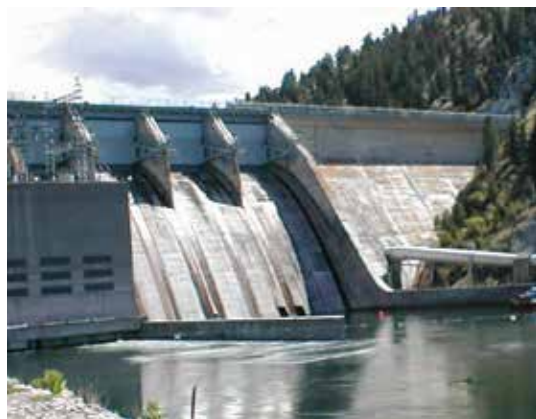
Fig. 2: Canyon Ferry Dam spillway, stilling basin and training wall
