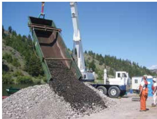
Fig. 4: Rubble removed from the basin floor
