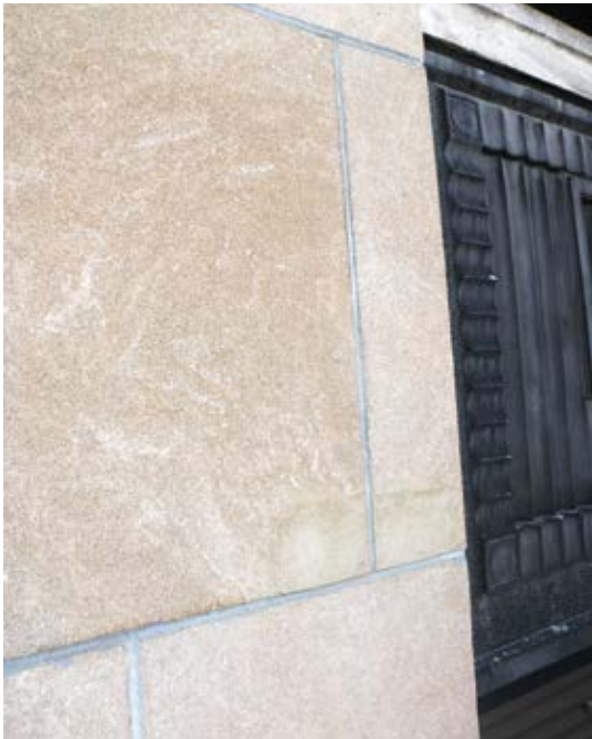
Fig. 6: Completed tuck-pointing of joints at stone panels
