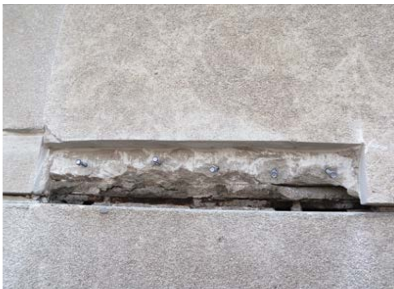
Fig. 4: Corrosion-resistant screws installed for anchorage of repair material
