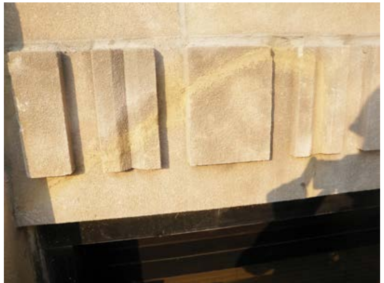
Fig. 8: Repaired crack shown in Fig. 7
