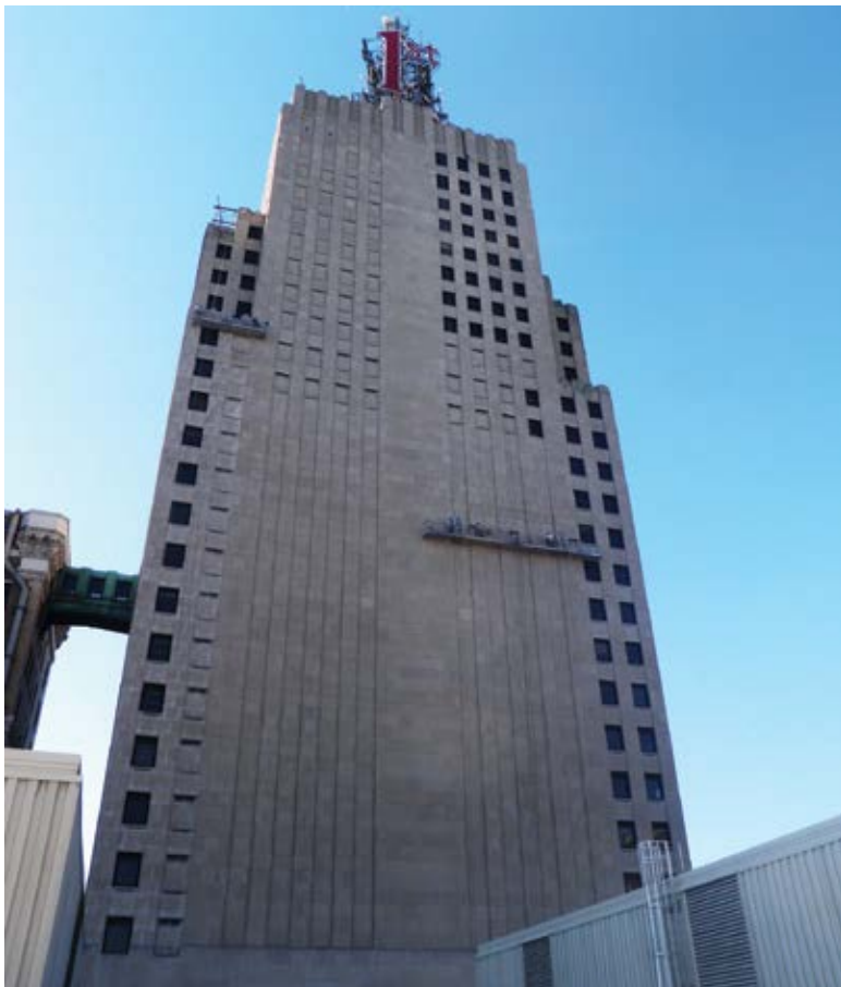
Fig. 1: North face of the First National Bank Building
