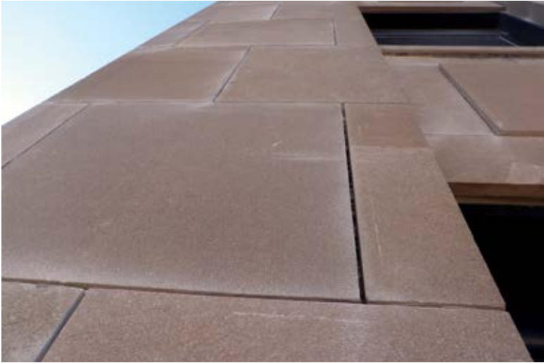
Fig. 5: Existing mortar at stone panel joints was removed prior to tuck-pointing
