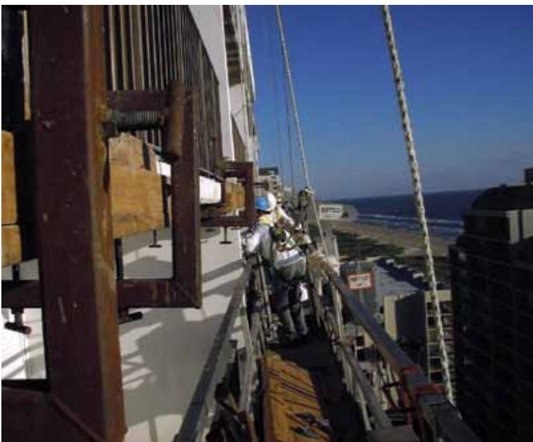
Repair work accomplished using swing stages
