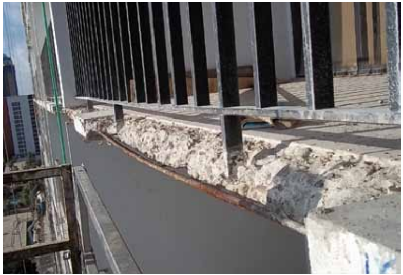
Balcony ready for repair material
