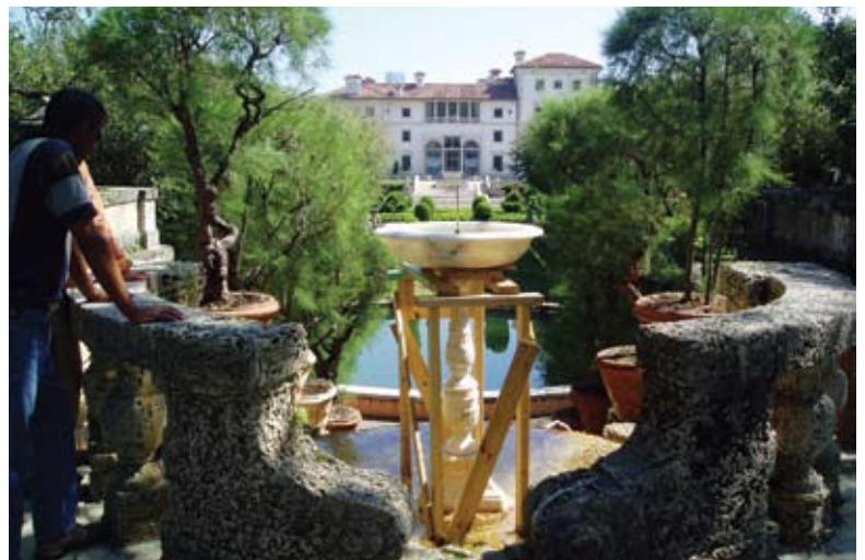
Temporary bracing on priceless marble fountain
