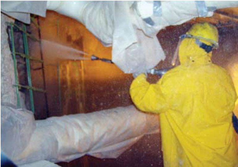
Final hydrodemolition preparation prior to applying shotcrete
