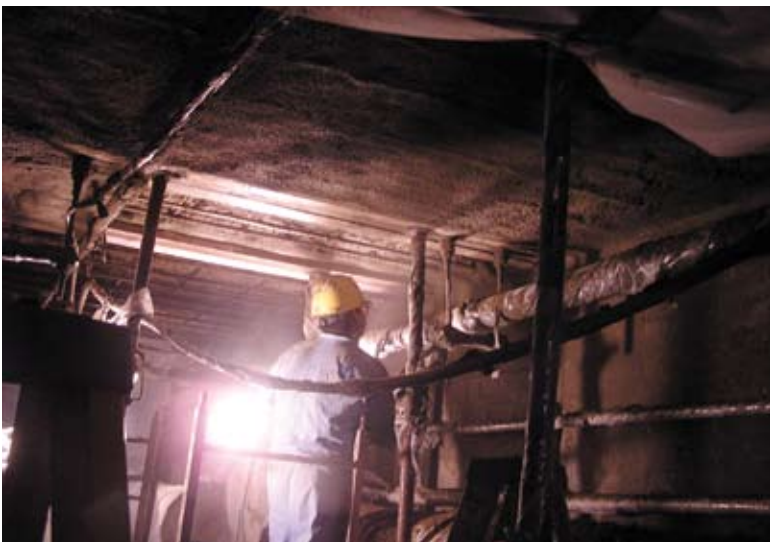
Nozzleman applying shotcrete
