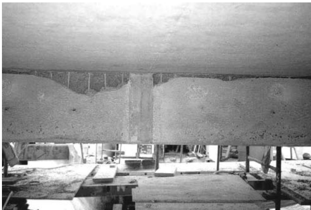
Effects of not filling the cavity.
