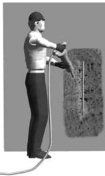
Unsound concrete removed with 15-lb chipping hammer. Hammers larger than 15-lb class may cause damage to substrate and reinforcement.
