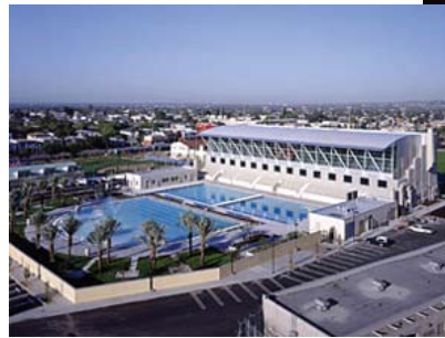
Overall view of completed project
