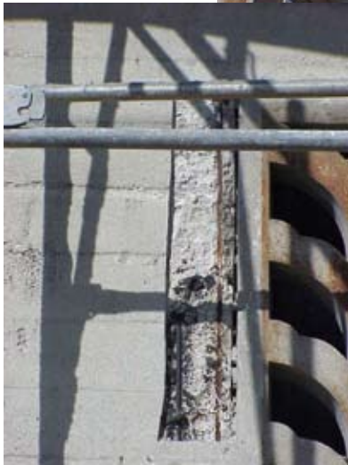
Close-up of ornamental detail repair
