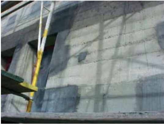
Patched area before coating
