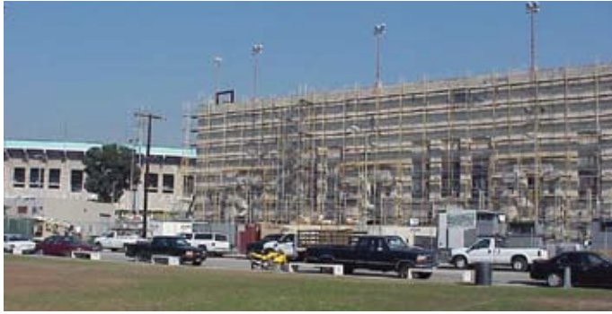
Extensive scaffolding was necessary for repairs
