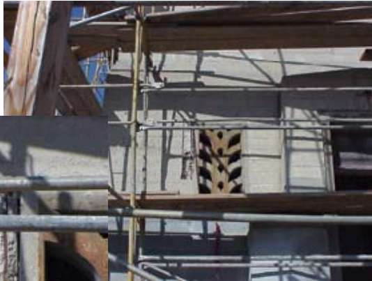
Ornamental detail repair
