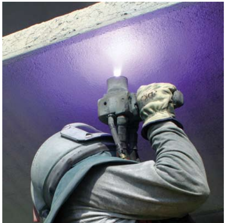
Installation of metallized cathodic protection system on underside of deck
