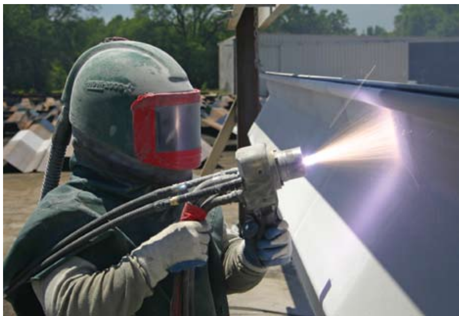
Metallizing for corrosion protection of steel using wire arc system
