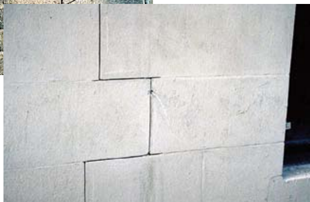
Fig. 4: Installation of ceramic discrete anodes
