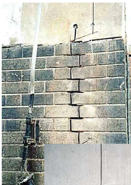
Fig. 4: Installation of ceramic discrete anodes
