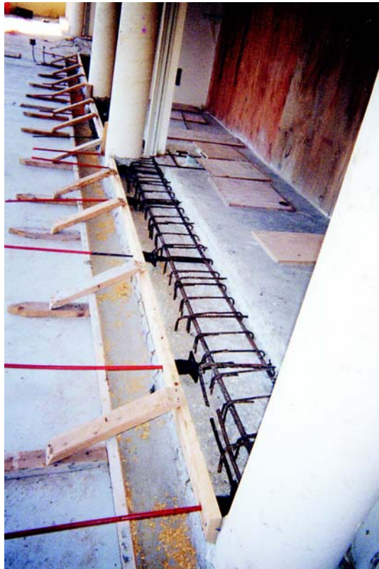
Correct repair of post-tensioned slab edge/beam
