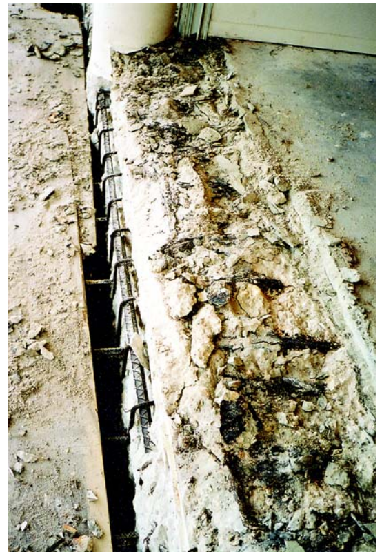
View of same area before repair
