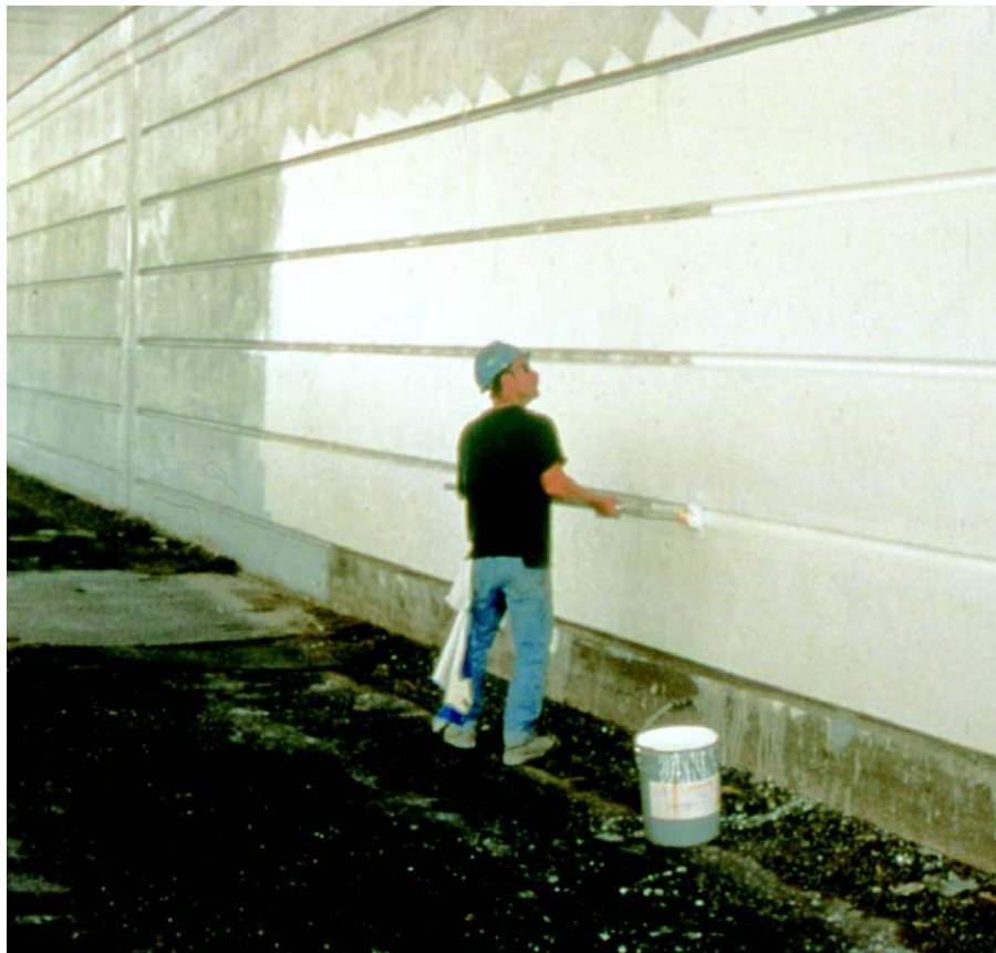
Urethane coatings can be applied easily by brush, roller, or sprayer at a thickness of 3 to 4 mils DFT
