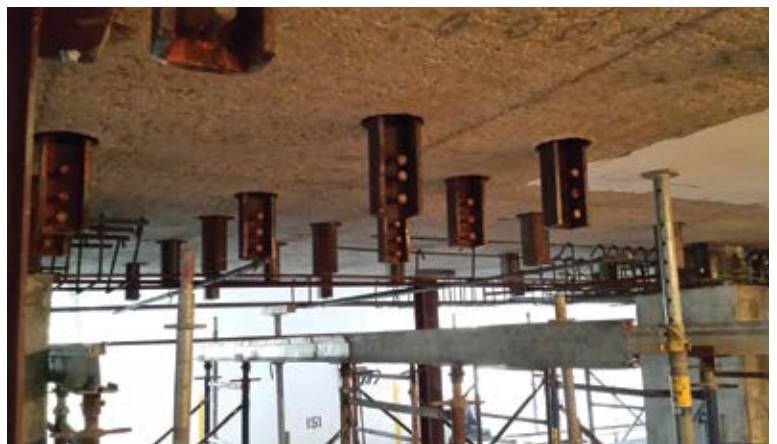
Steel lug keys and reinforcing bars in the drop panels
