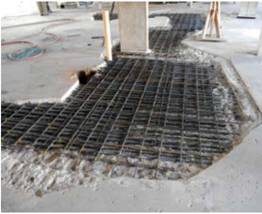
Fourth-level transfer slab crack repair after demolition
