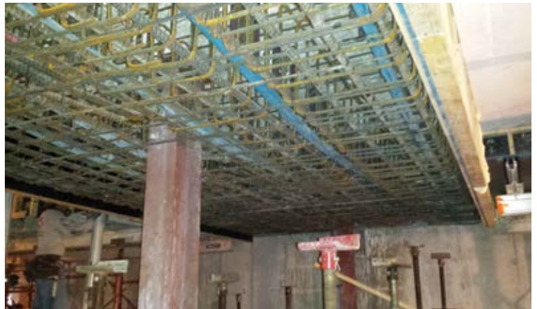
Post-tensioned drop panels with formwork
