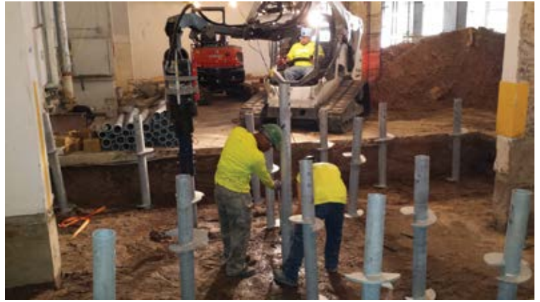
Helical pile installation in the foundation area
