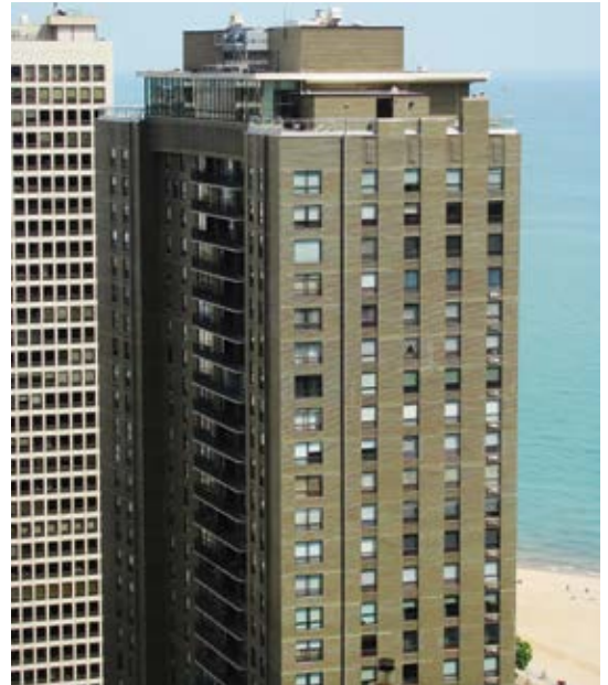
Chicago condominium complex where roof sundeck rehabilitation was performed
