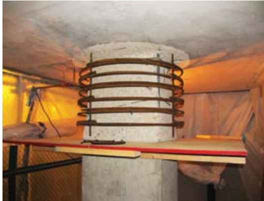
Typical interior column strengthening with hoop reinforcement for shear collar
