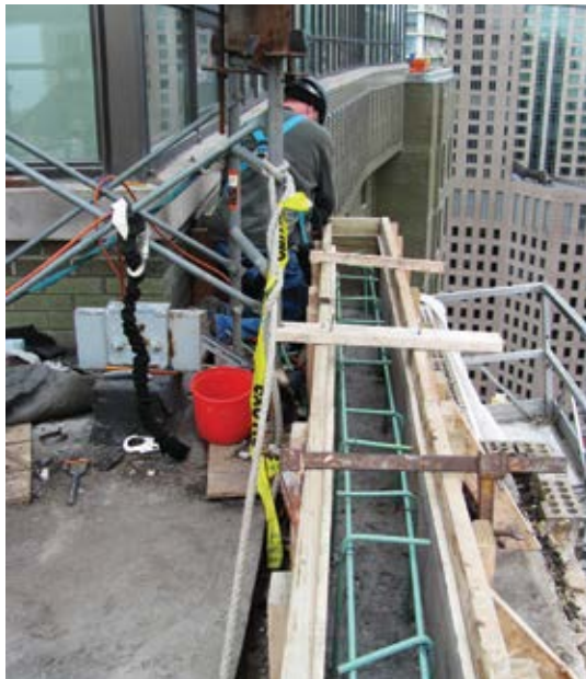
Typical perimeter concrete curb prior to concrete placement
