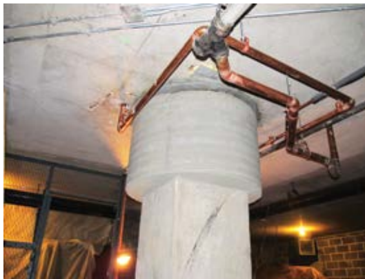
Typical interior column with shear collar
