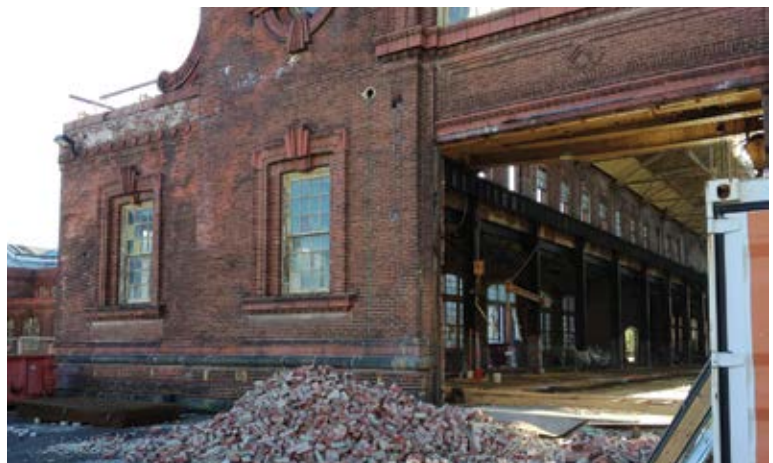
Removal of damaged masonry
