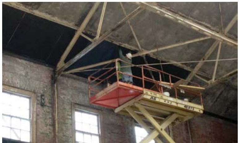
Installation of carbon fiber wrap
