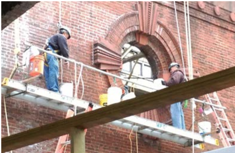
Repair of masonry in progress
