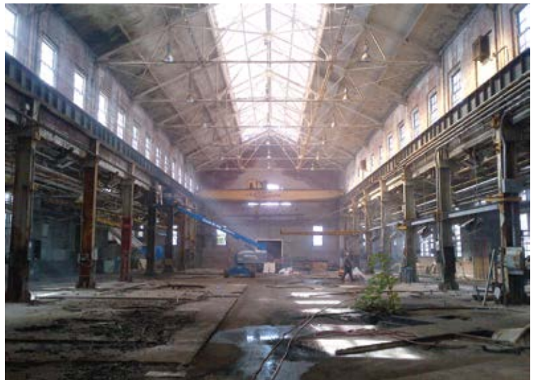
Inside Building 18 before the renovations
