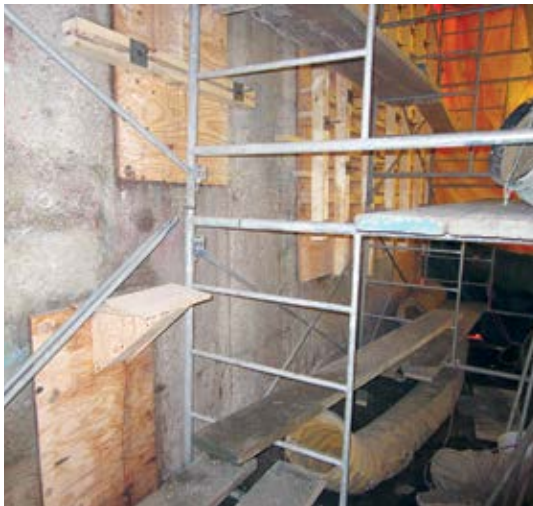
Plywood formwork in place for form-and-pour repairs
