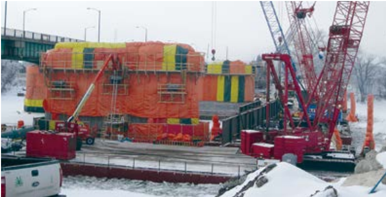
Repair and corrosion mitigation of piers proceeded inside heated enclosures
