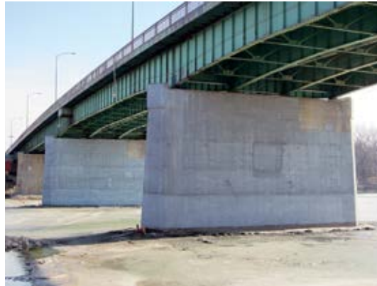
Humectant-activated arc sprayed zinc was used to protect the two interior piers
