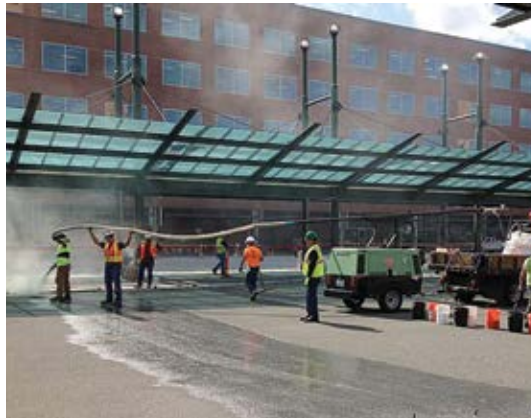
Crews apply a traffic-bearing coating in the public transportation area
