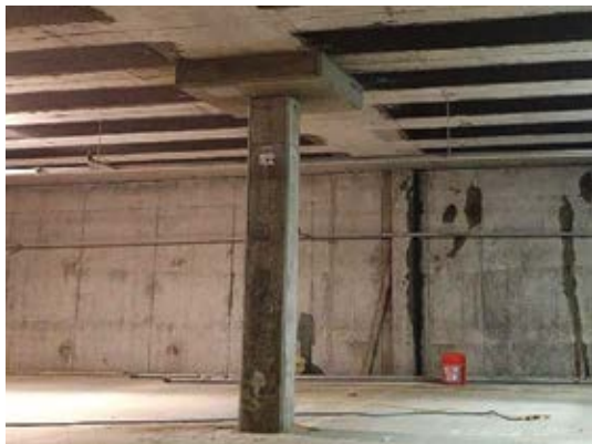
FRP system installed
