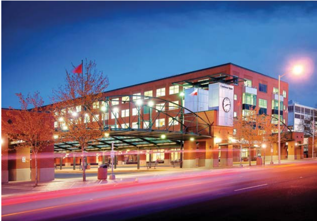
Courthouse Square is a five-story complex that contains municipal space, retail, offices, a public transportation center, and an underground parking garage
