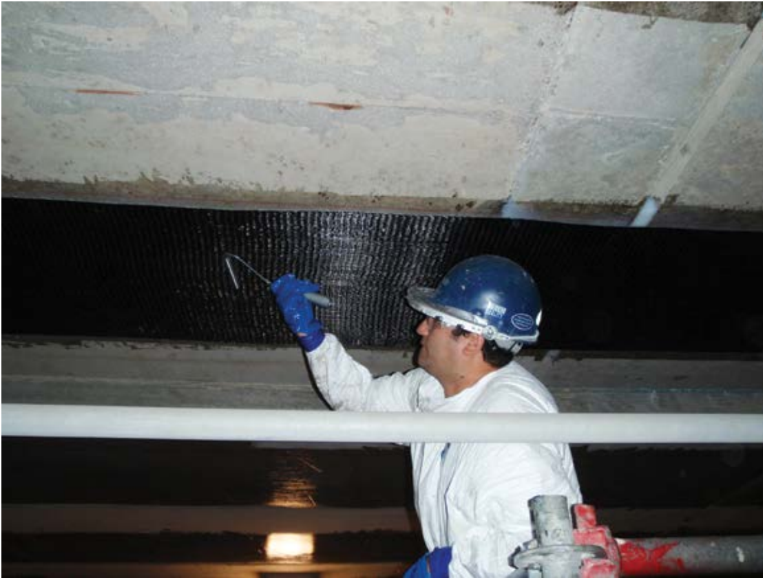
Installation of the FRP composite strengthening system
