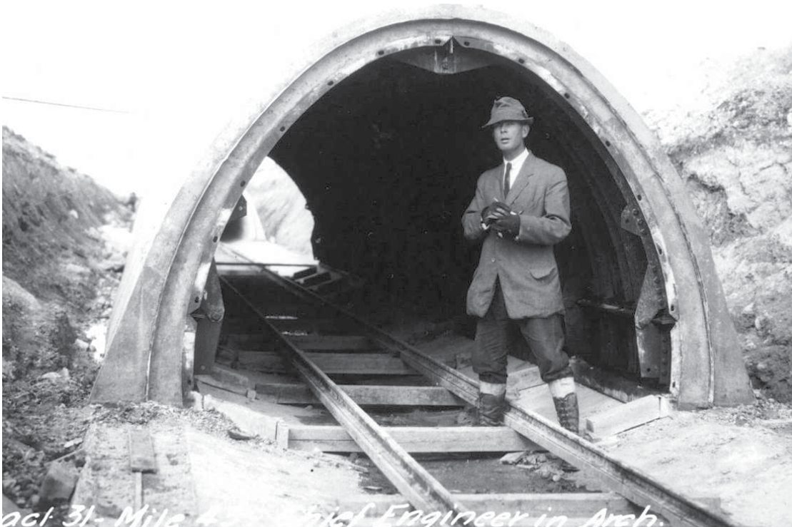
Photo of aqueduct during original construction
