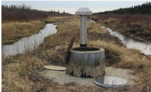
Manhole in section of underground aqueduct
