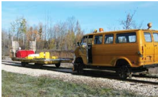
System of moving materials and equipment using original railway
