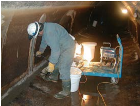
Worker preparing to inject urethane
