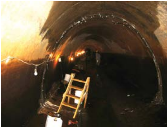
Inside of aqueduct after injection
