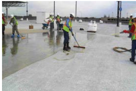
Fig. 5: Epoxy overlay installation
