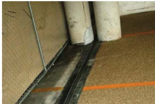
Fig. 4: Replacement expansion joint (epoxy overlay on right; existing concrete slab on left)
