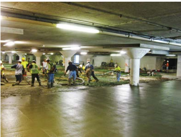
Crews placing concrete
