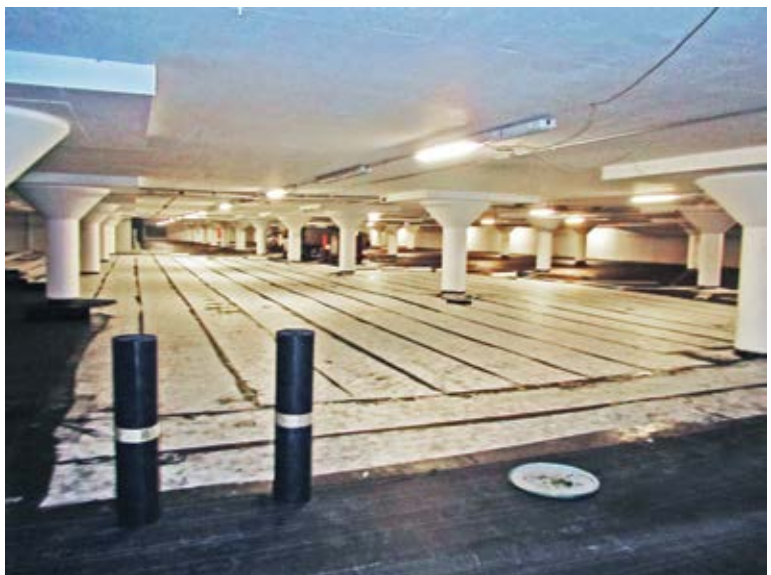
Waterproofing of the parking garage and repaired ceiling prior to painting
