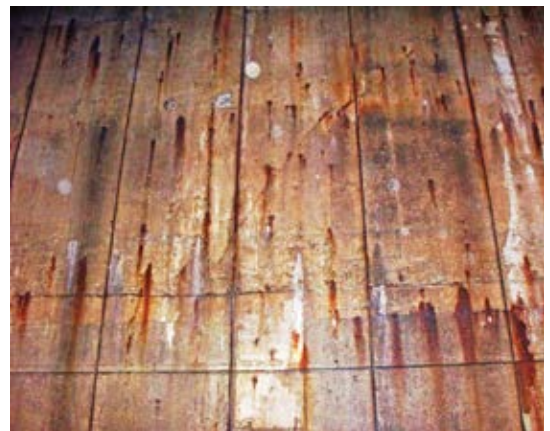
Existing conditions on the north wall prior to repair
