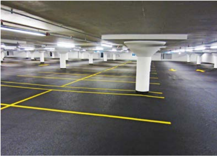
Finished drive lane of the parking garage
