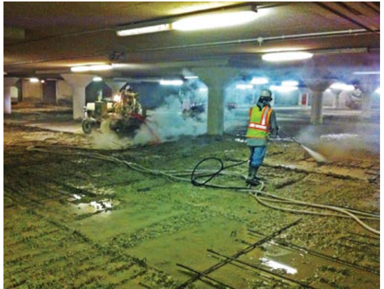
Up to five hydrodemolition machines working at once
