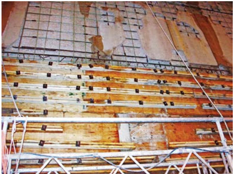
Placing of concrete at the north wall
