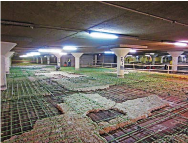
Prepour inspection of a concrete slab that includes full-depth repairs
