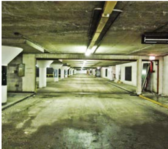
Existing drive lane of the parking garage prior to repair
