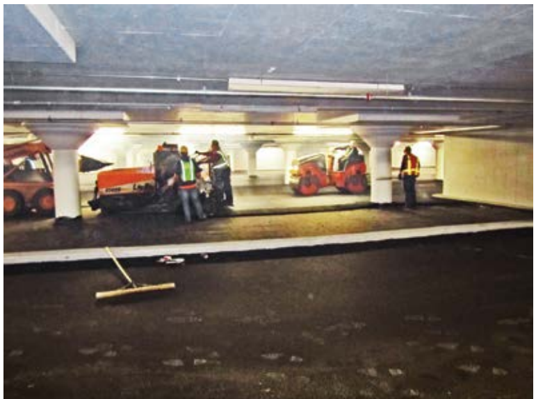
Waterproofing and asphalt process on the upper level
