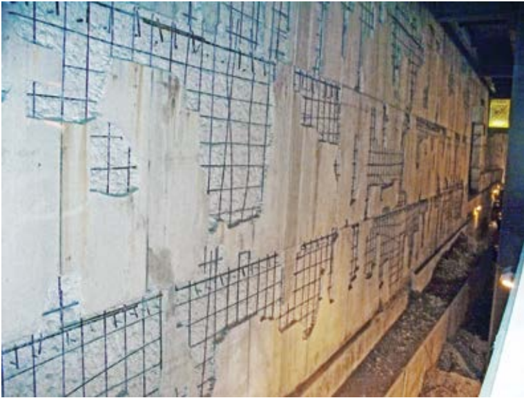
North wall demolition and prep for receiving concrete
