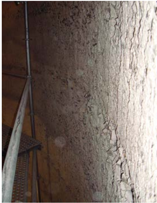
Existing condition of silo wall prior to rehabilitation
