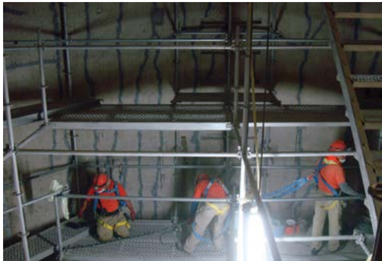
Epoxy injection of cracks
