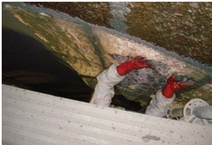
Worker applying reinforcing mesh to silo wall
