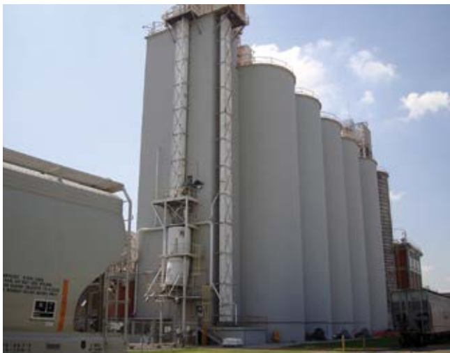
Exterior view of silo facility
