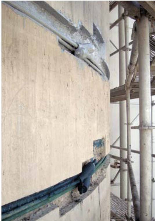
Post-tensioning cable installation
