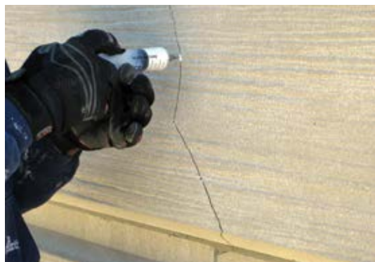
Dispersed hydrated lime being injected into crack
