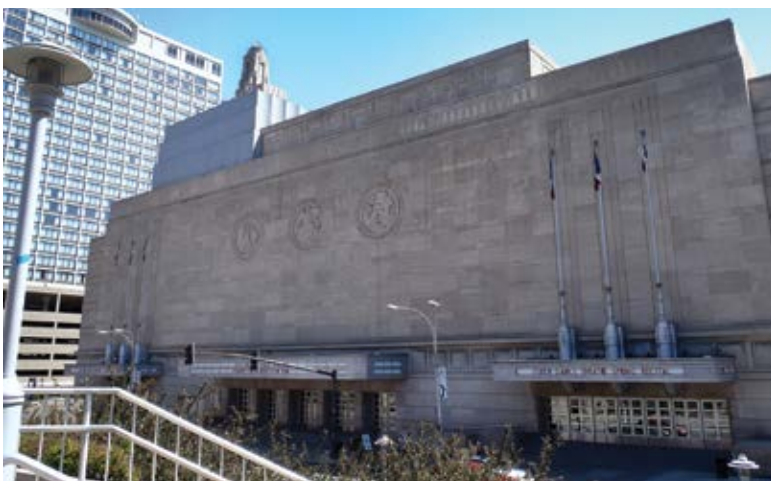
Exterior view of completed restoration
