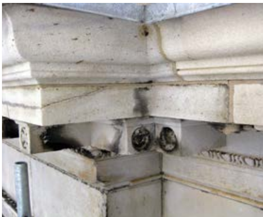
Condition of cornice prior to restoration
