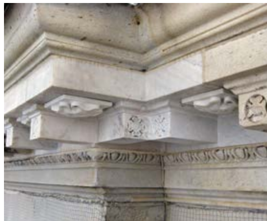
Repaired cornice area
