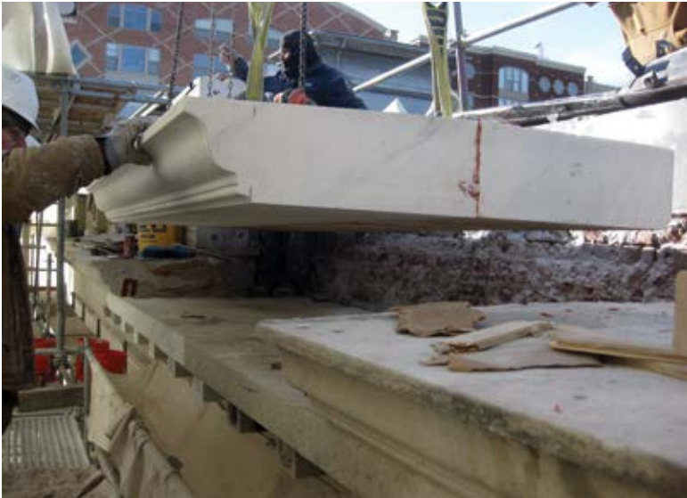
Setting new cornice section
